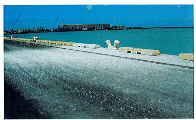
Photo 7, cement spatter covers pier pavement and bollard
