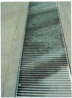
Photo 8, trench drain grates caked with cement
