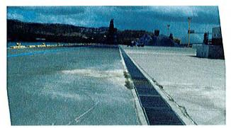
Photo 3, sand used a oil spill blotter not cleaned up, also present in trench drain
