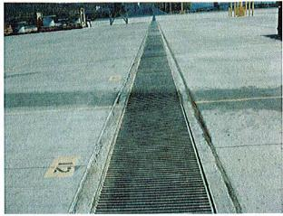
Photo 2: Oil spill residue across trench drain, drain interior has oily sand
