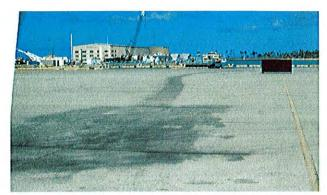
Photo 1: Residue from oil spill extending from Pier Shed towards Harbor
