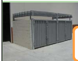
Secured Enclosure – Minimized Illegal Dumping. Add non- galvanized corrugated roofing to prevent rain runoff.
