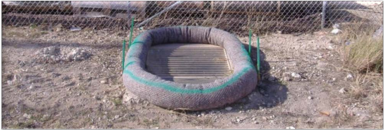
Drain Inlet Control, Barbers Point. January 2006.
