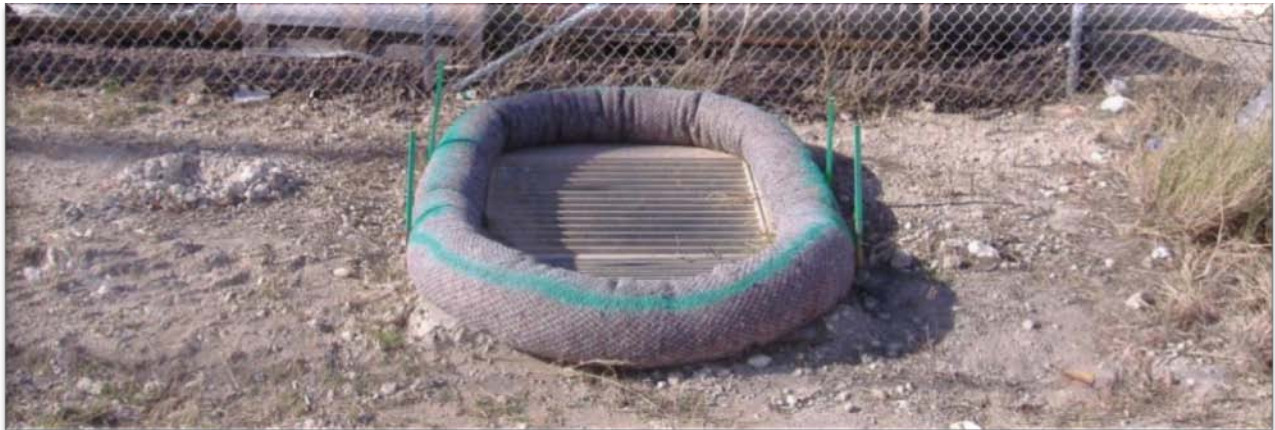
Drain Inlet Control, Barbers Point. January 2006.
