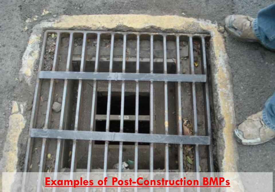
PERMANENT DRAIN INLET FILTERS
