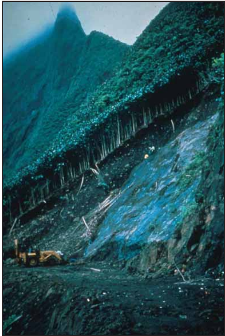
In Tahiti, landslides occur in places invaded by dense stands of miconia ( Miconia calvescens ) and interfere with road building. There is still time to prevent the widespread invasion of miconia on Maui, O'ahu and Kaua'i.
