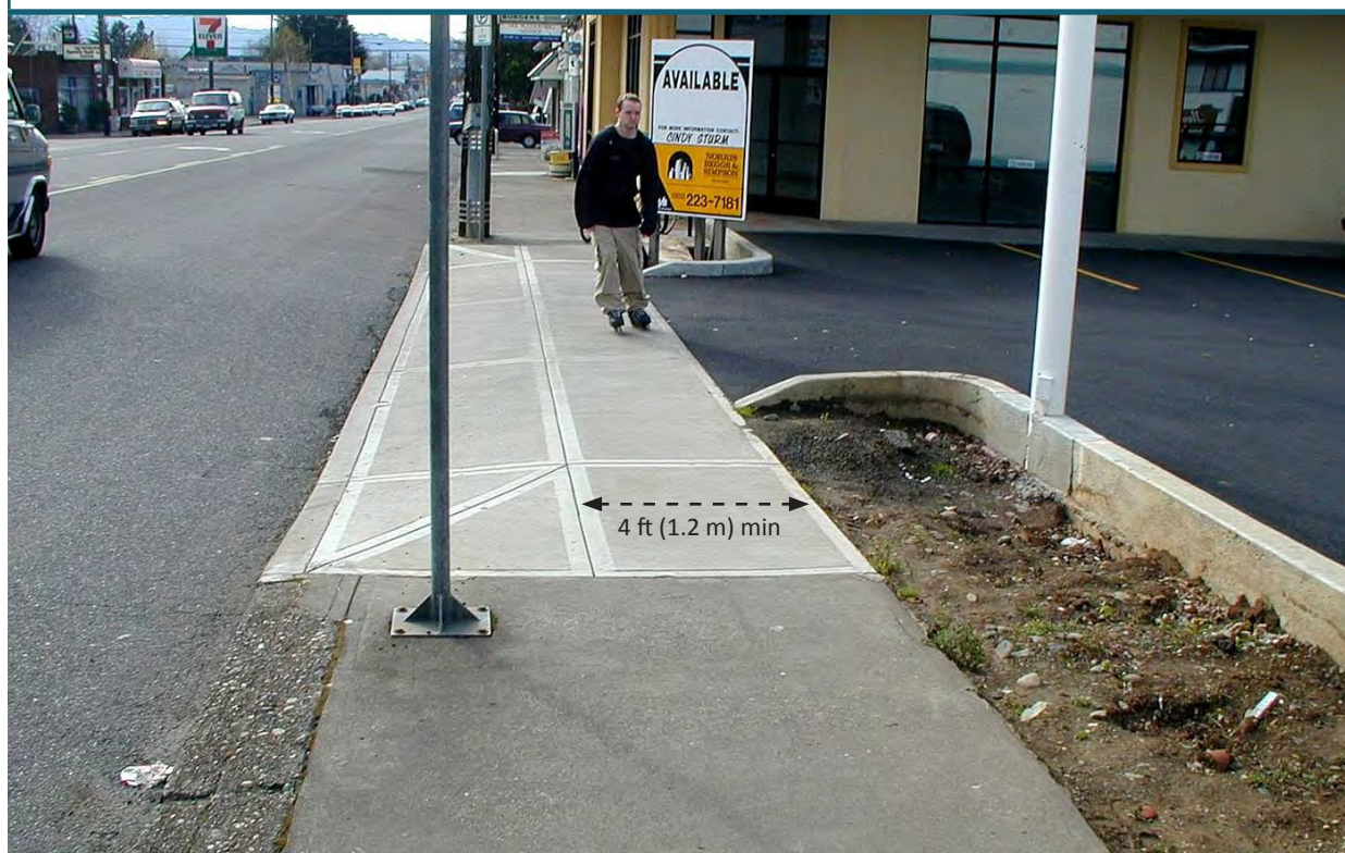
EXHIBIT 3.25 An existing driveway apron has been reconstructed to provide a level pedestrian route across it.
