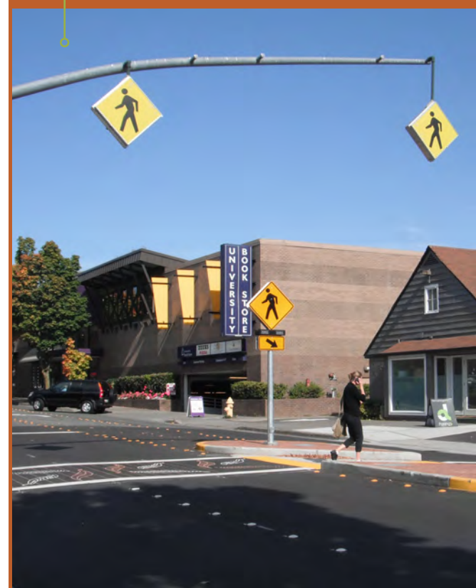
New mid-block crossing in a busy commercial area, designed with flashing signs and high contrast crossing area, Downtown Bellevue, WA
