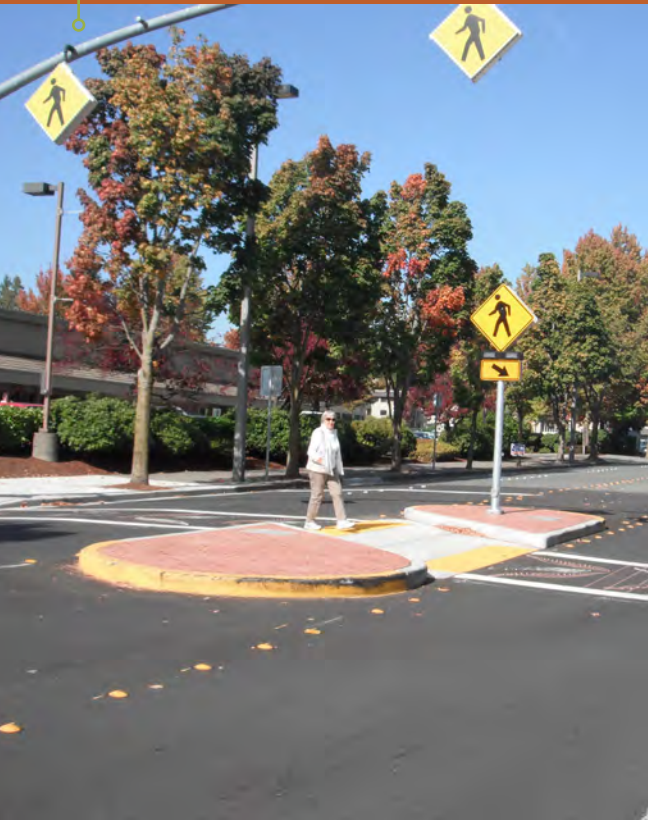
The crossing area is angled to orient pedestrians to the view of oncoming traffic.
