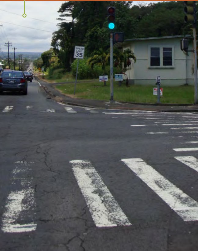
Painted markings can deteriorate quickly. Regular inspection and maintenance contribute to pedestrian safety.
