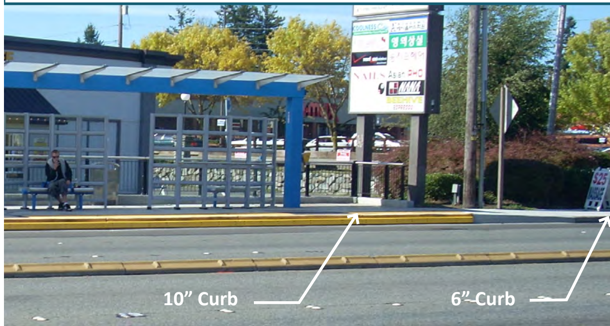
EXHIBIT 6.15 Sidewalk Ramping from a 6 in (15.2 cm) Curb Height to a 10 in (25.4 cm) Platform Height
