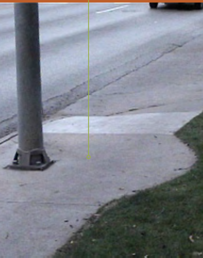
Sidewalk widens as it passes obstruction to maintain PAR width.
