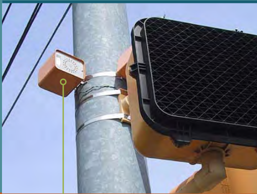
Speaker mounted above a pedestrian signal (NCHRP)
