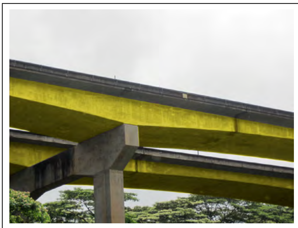
Photo: Element 104 - Prestressed Concrete Closed Web / Box Girder (Highlighted)
