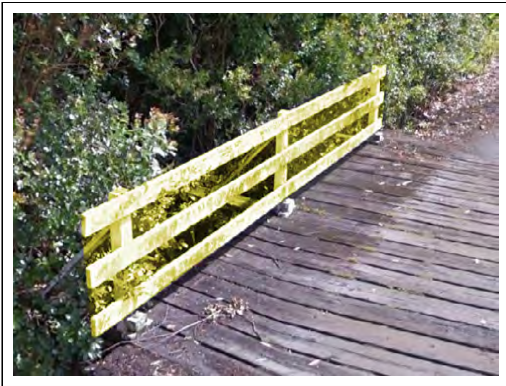
Photo: Element 332 - Timber Bridge Railing (Highlighted)
