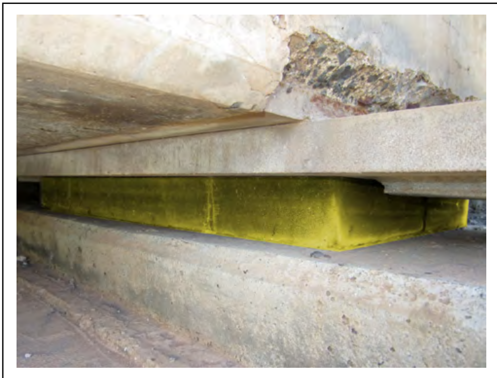
Photo: Element 310 - Elastomeric Bearing (Highlighted)
