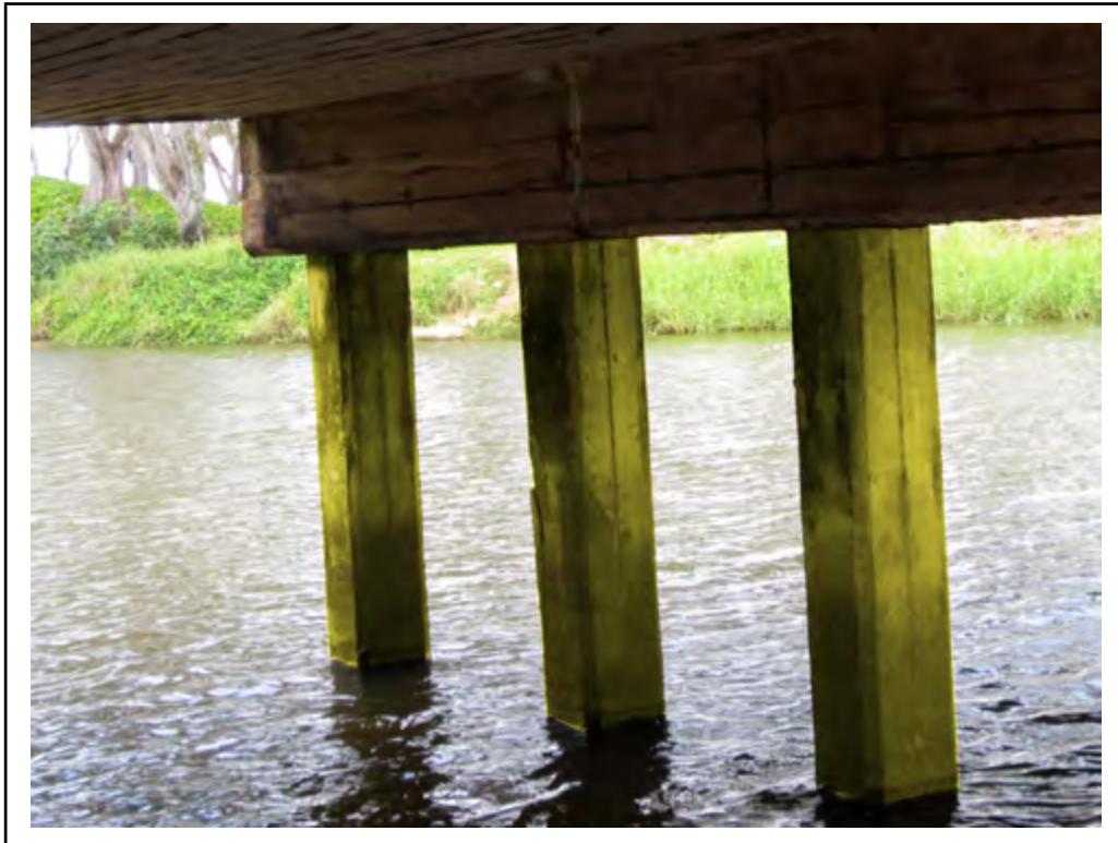
Photo: Element 227 - Reinforced Concrete Pile (Highlighted)
