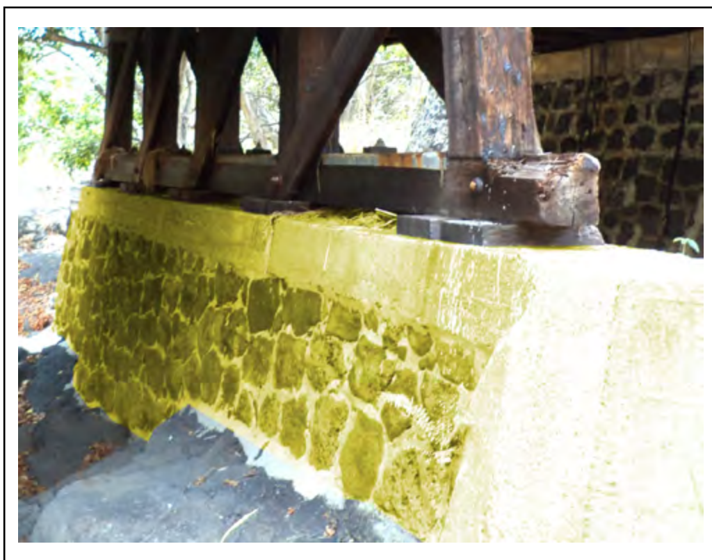
Photo: Element 213 - Masonry Pier Wall (Highlighted)
