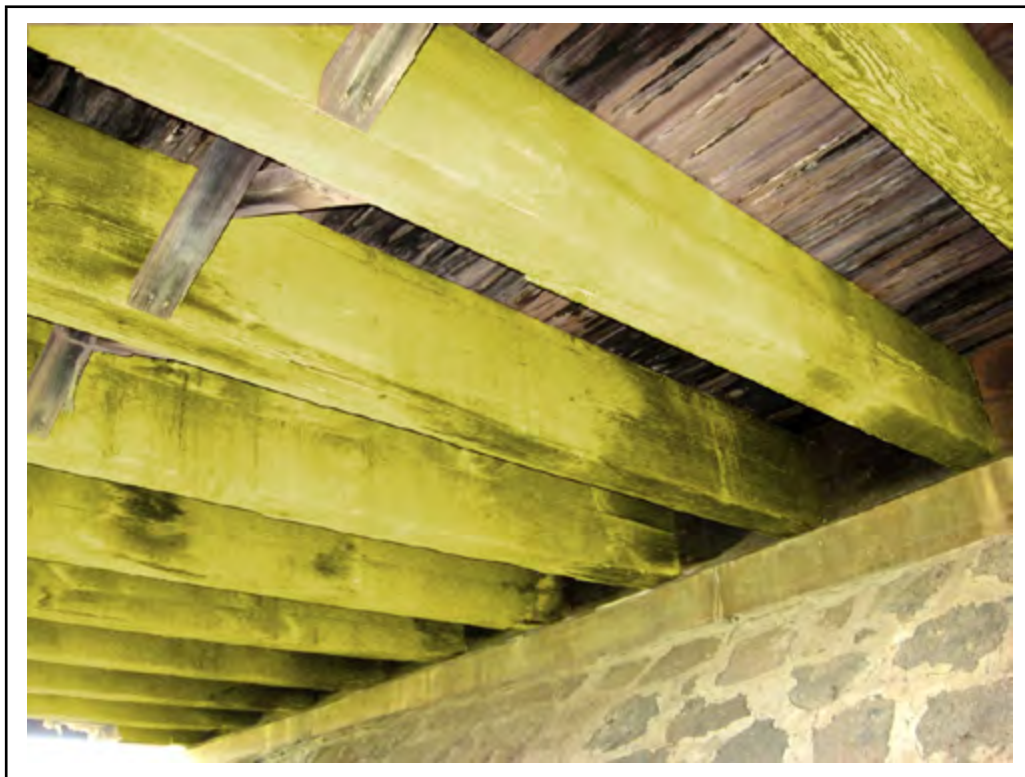
Photo: Element 111 - Timber Open Girder / Beam (Highlighted)
