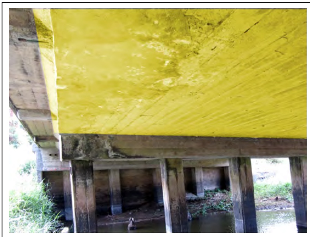
Photo: Element 38 - Reinforced Concrete Slab (Highlighted)
