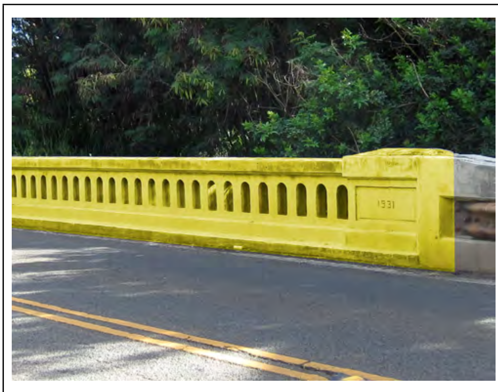
Photo: Element 331 - Reinforced Concrete Bridge Railing (Highlighted)
