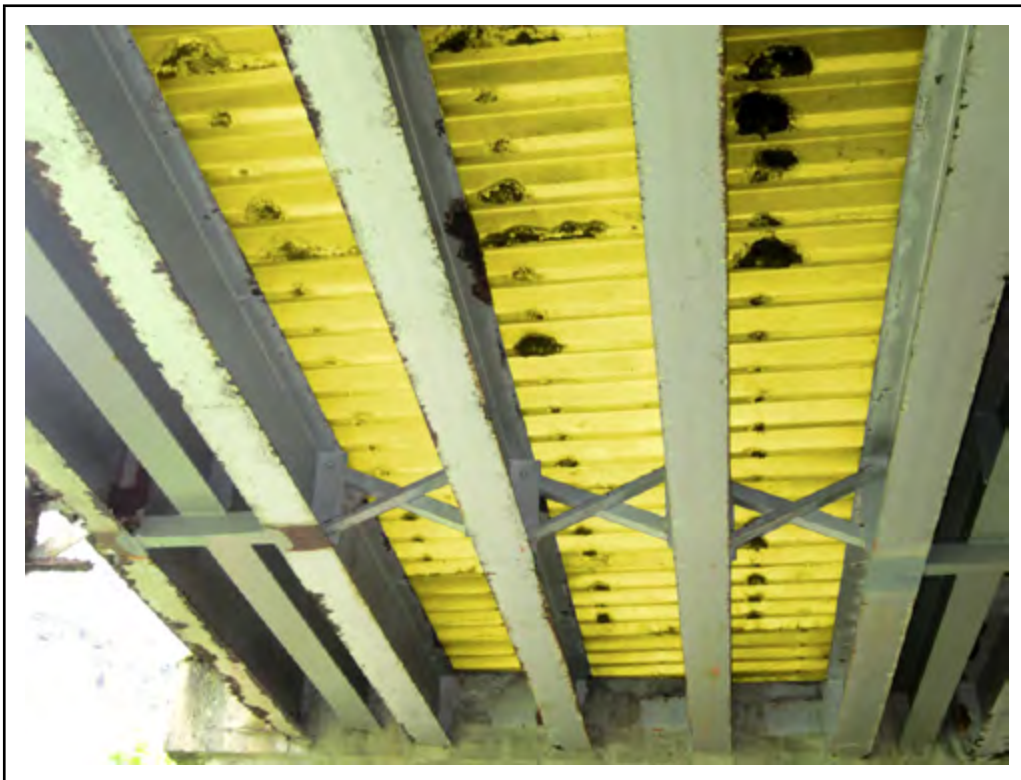
Photo: Element 30 - Steel Deck with Corrugated / Orthotropic / Etc. (Highlighted)
