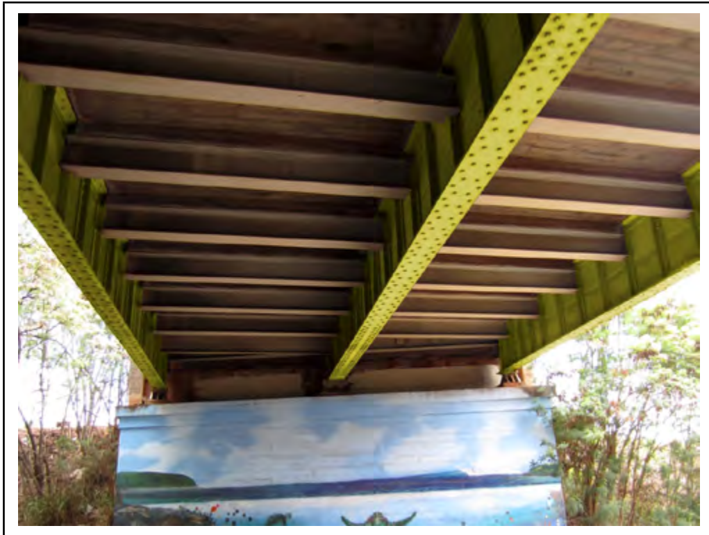
Photo: Element 107 - Steel Open Girder / Beam (Highlighted)
