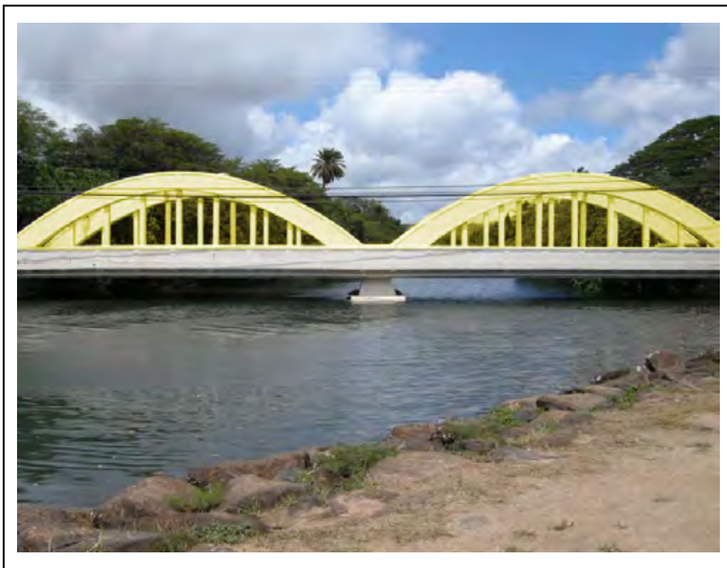
Photo: Element 144 - Reinforced Concrete Arch (Highlighted)
