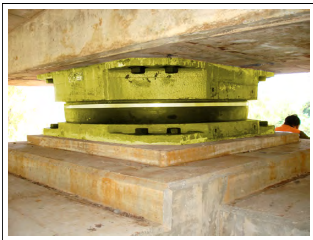
Photo: Element 314 - Pot Bearing (Highlighted)
