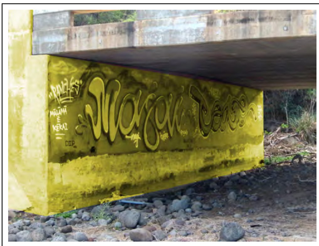
Photo: Element 215 - Reinforced Concrete Abutment (Highlighted)
