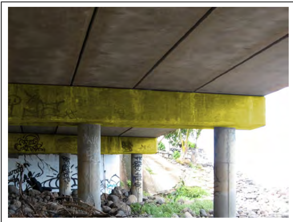
Photo: Element 234 - Reinforced Concrete Pier Cap (Highlighted)
