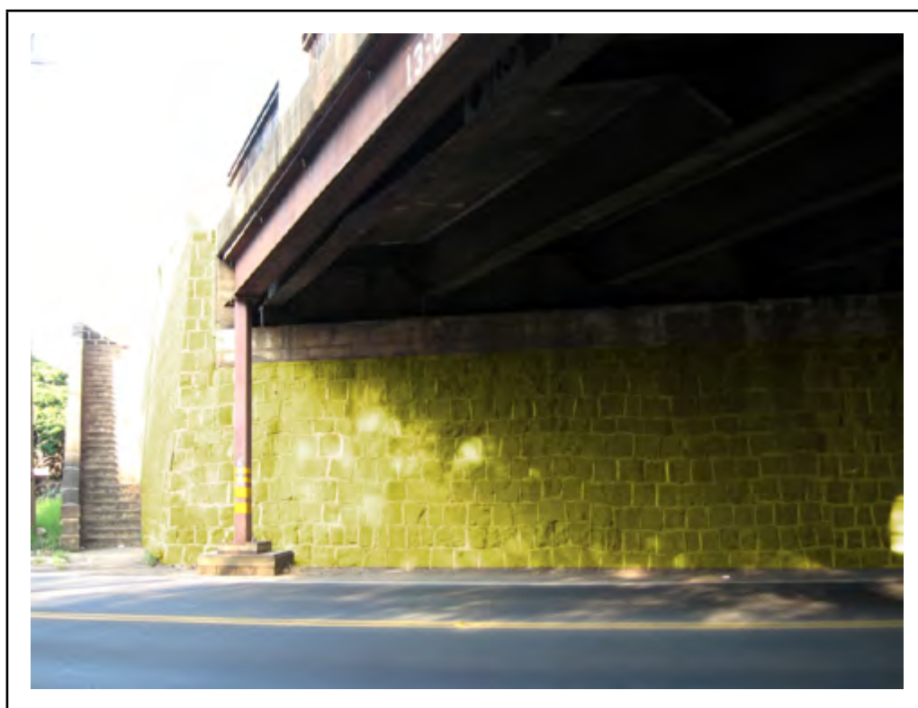
Photo: Element 217 - Masonry Abutment (Highlighted)
