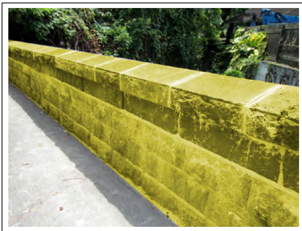
Photo: Element 334 - Masonry Bridge Railing (Highlighted)
