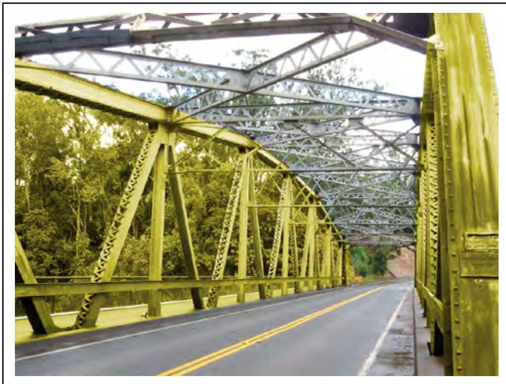
Photo: Element 120 - Steel Truss (Highlighted)
