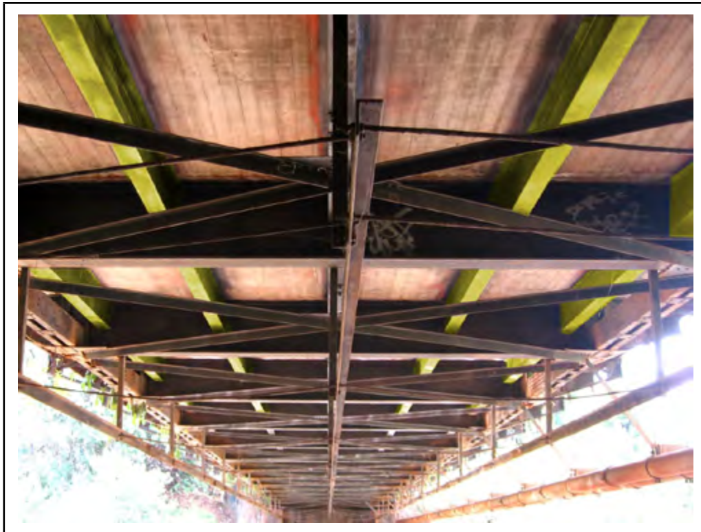
Photo: Element 113 - Steel Stringer (Highlighted)
