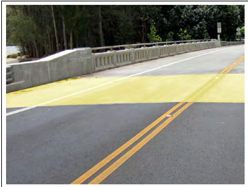
Photo: Element 321 - Reinforced Concrete Approach Slab (Highlighted)
