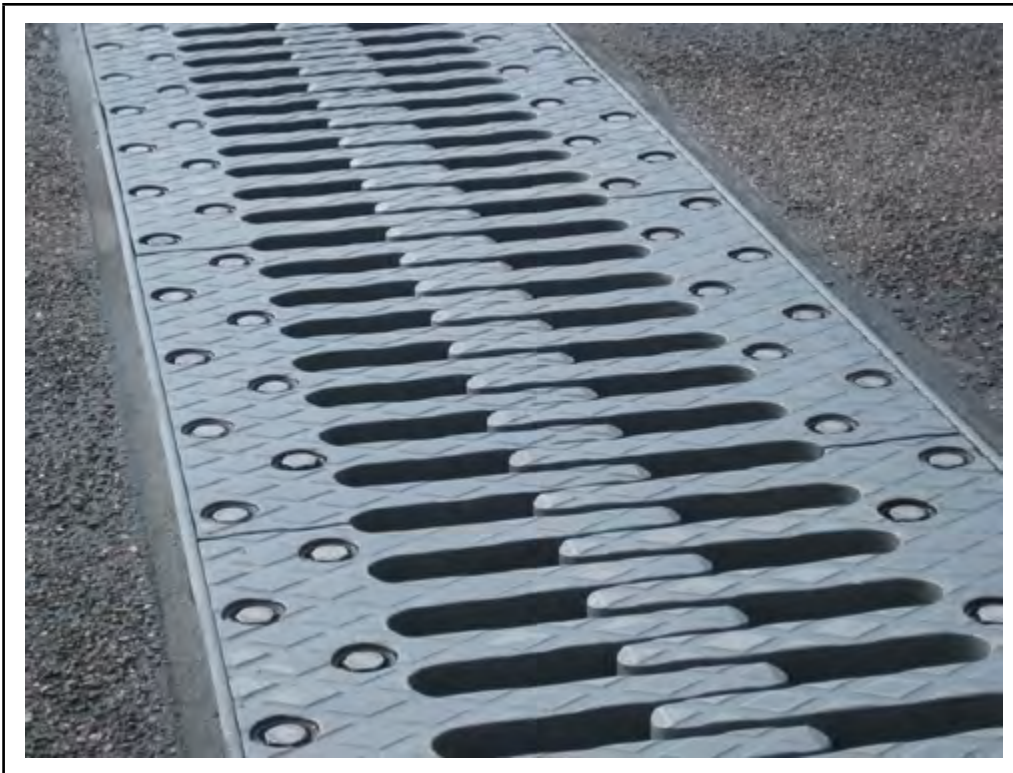
Photo: Element 305 - Assembly Joint without Seal
