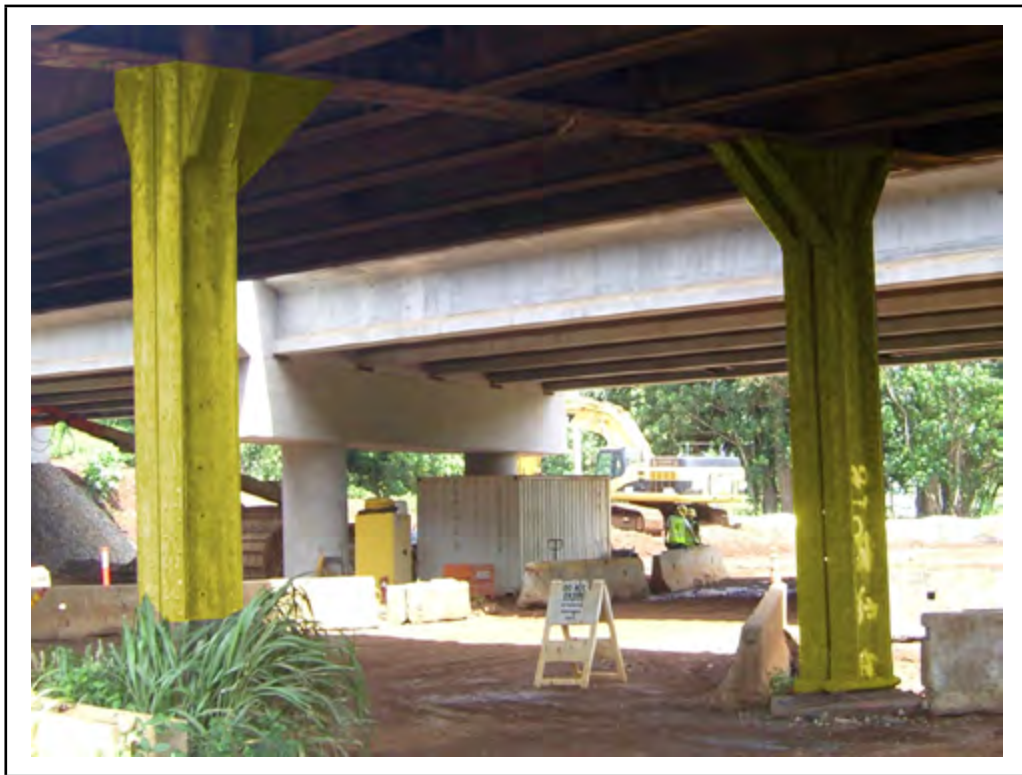
Photo: Element 202 - Steel Column (Highlighted)
