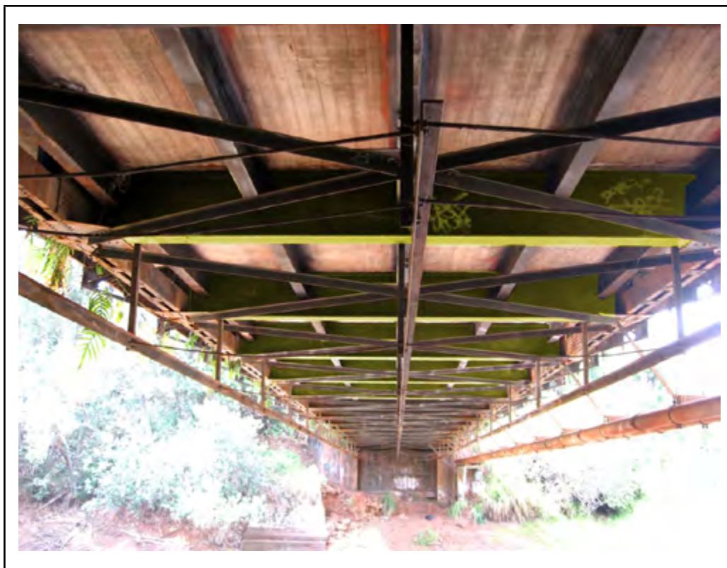
Photo: Element 152 - Steel Floor Beam (Highlighted)
