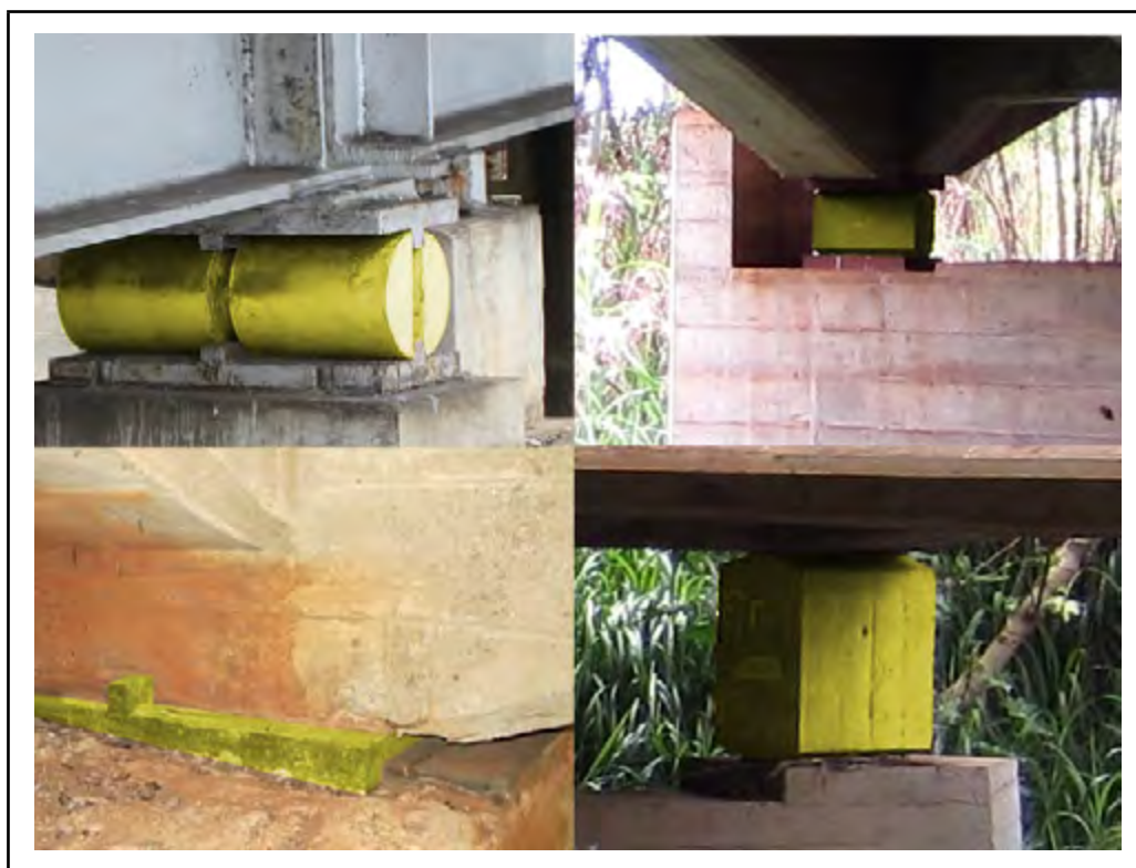
Photo: Element 311 - Moveable Bearing (Highlighted)
