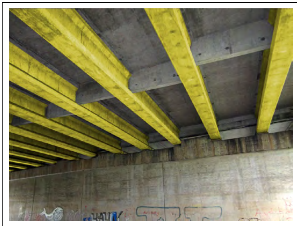
Photo: Element 109 - Prestressed Concrete Open Girder / Beam (Highlighted)
