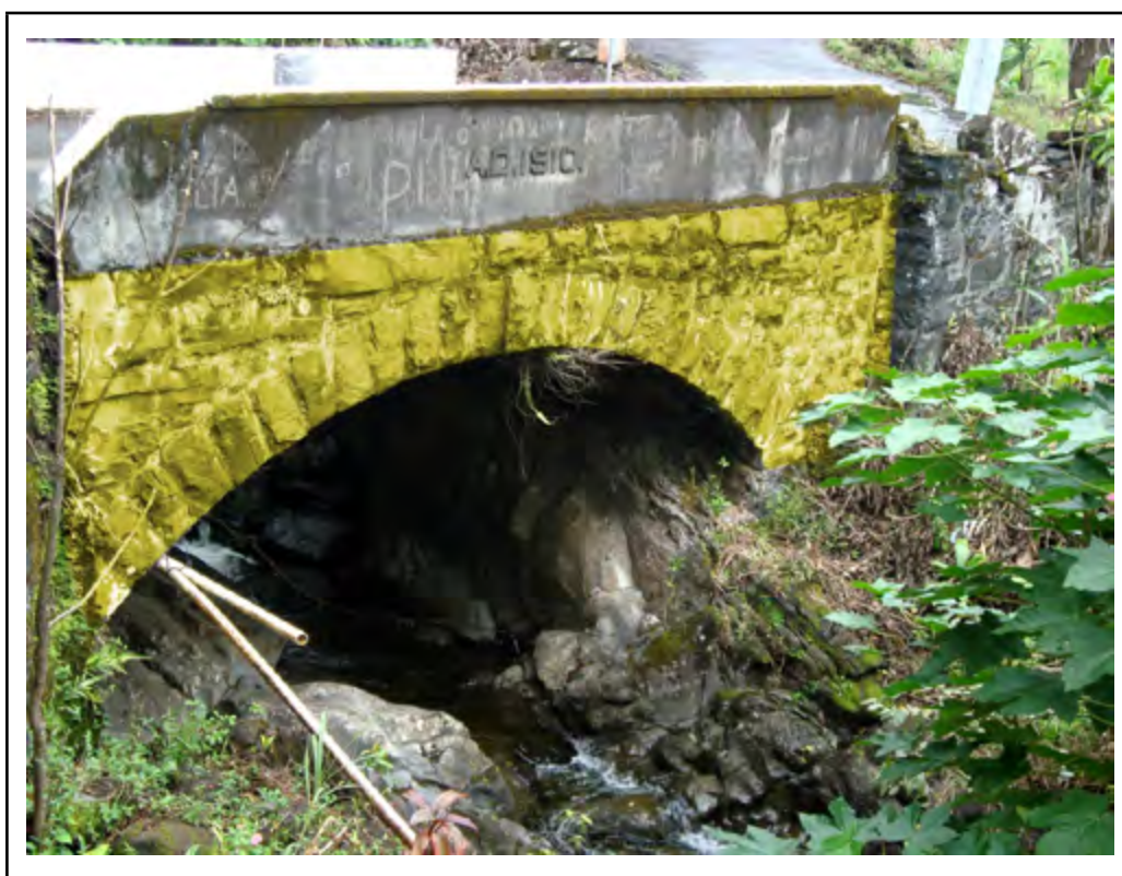
Photo: Element 145 - Masonry Arch (Highlighted)
