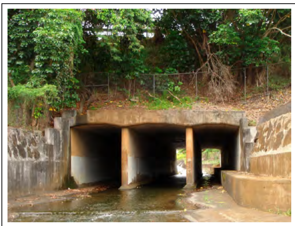
Photo: Element 241 - Reinforced Concrete Culvert
