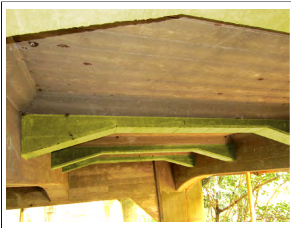
Photo: Element 155 - Reinforced Concrete Floor Beam (Highlighted)
