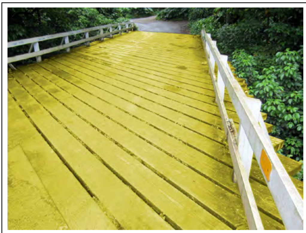
Photo: Element 31 - Timber Deck (Highlighted)
