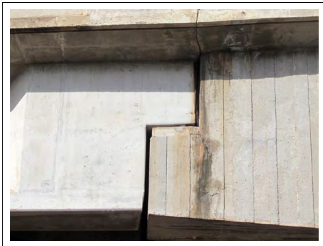
Photo: Element 312 - Enclosed / Concealed Bearing
