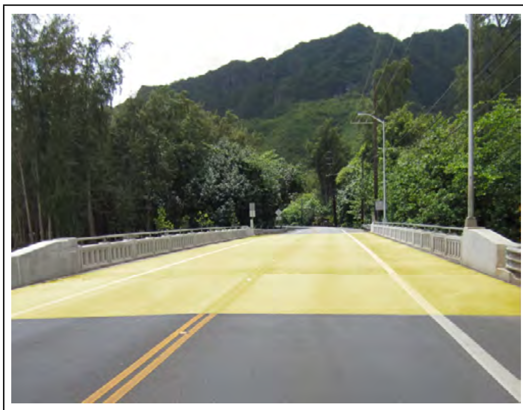
Photo: Element 12 - Reinforced Concrete Deck (Highlighted)
