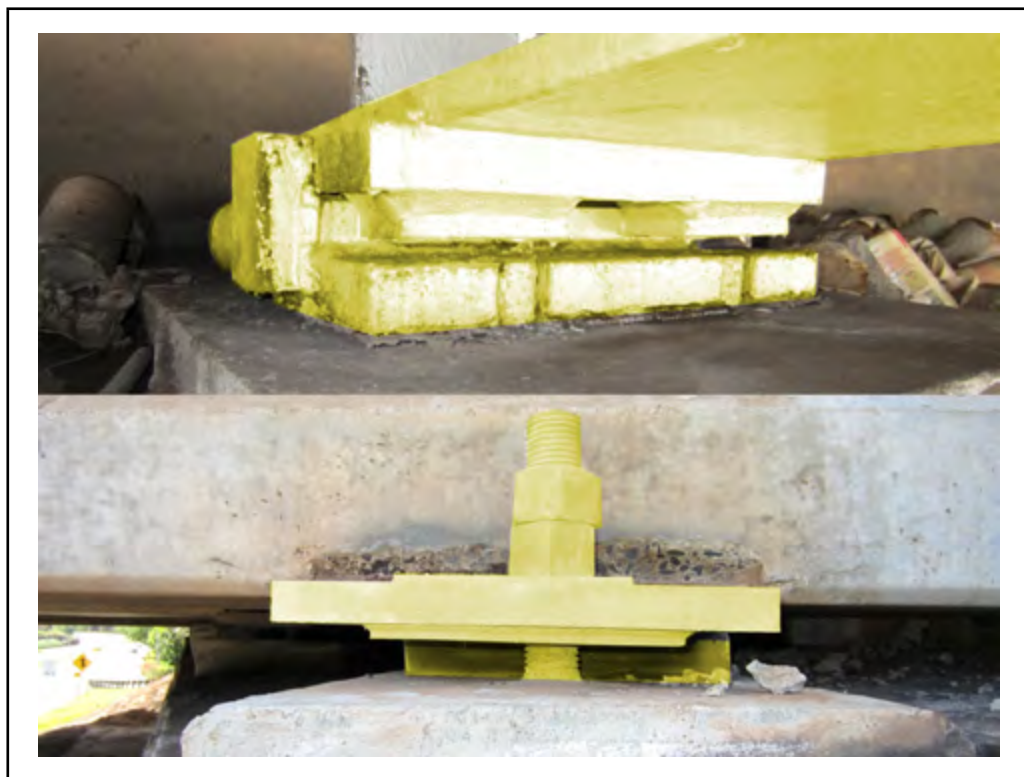
Photo: Element 313 - Fixed Bearing (Highlighted)
