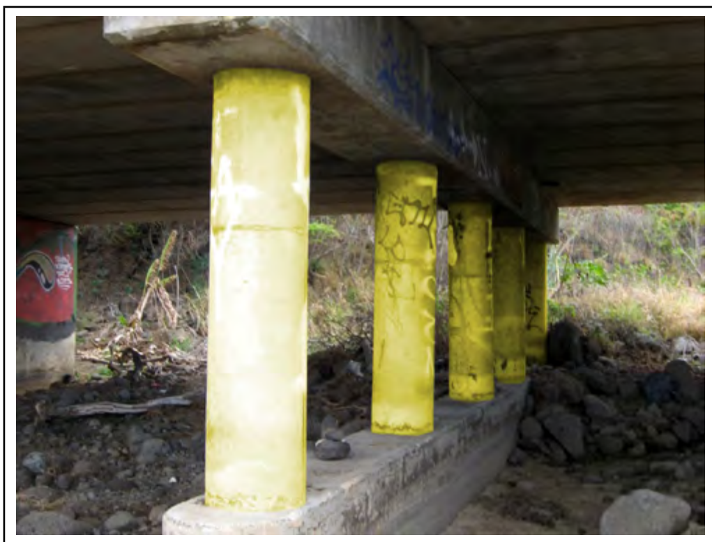
Photo: Element 205 - Reinforced Concrete Column (Highlighted)
