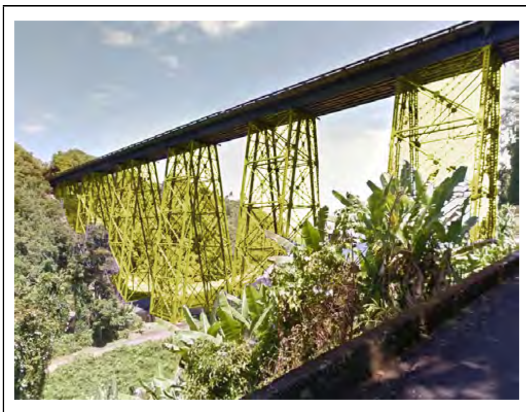
Photo: Element 202 - Steel Tower (Highlighted)
