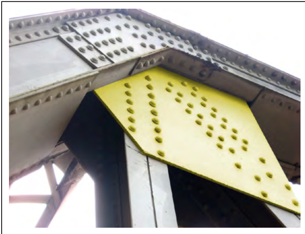
Photo: Element 162 - Steel Gusset Plate (Highlighted)
