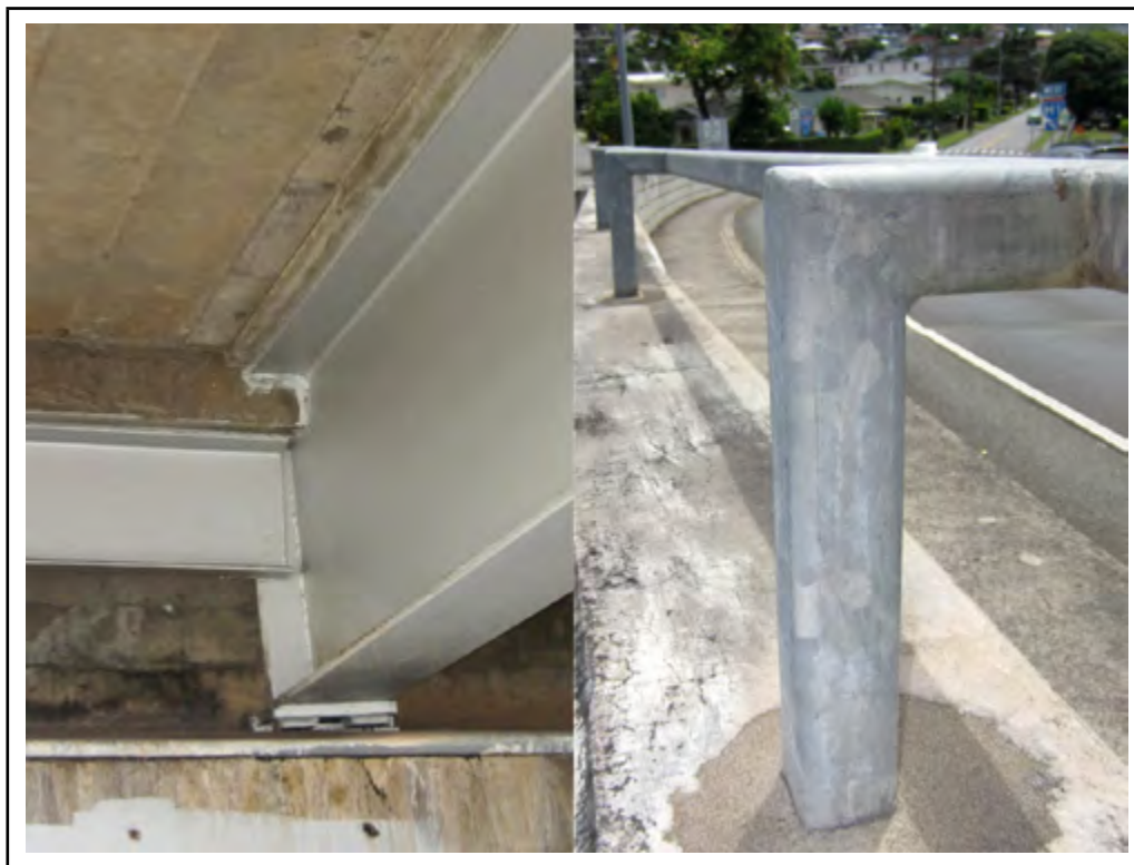
Photo: Element 515 - Steel Protective Coating
