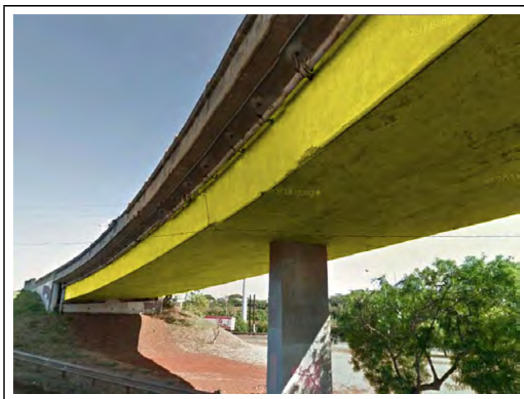
Photo: Element 105 - Reinforced Concrete Closed Web / Box Girder (Highlighted)
