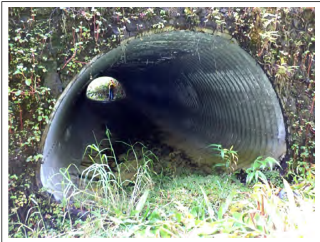
Photo: Element 240 - Steel Culvert
