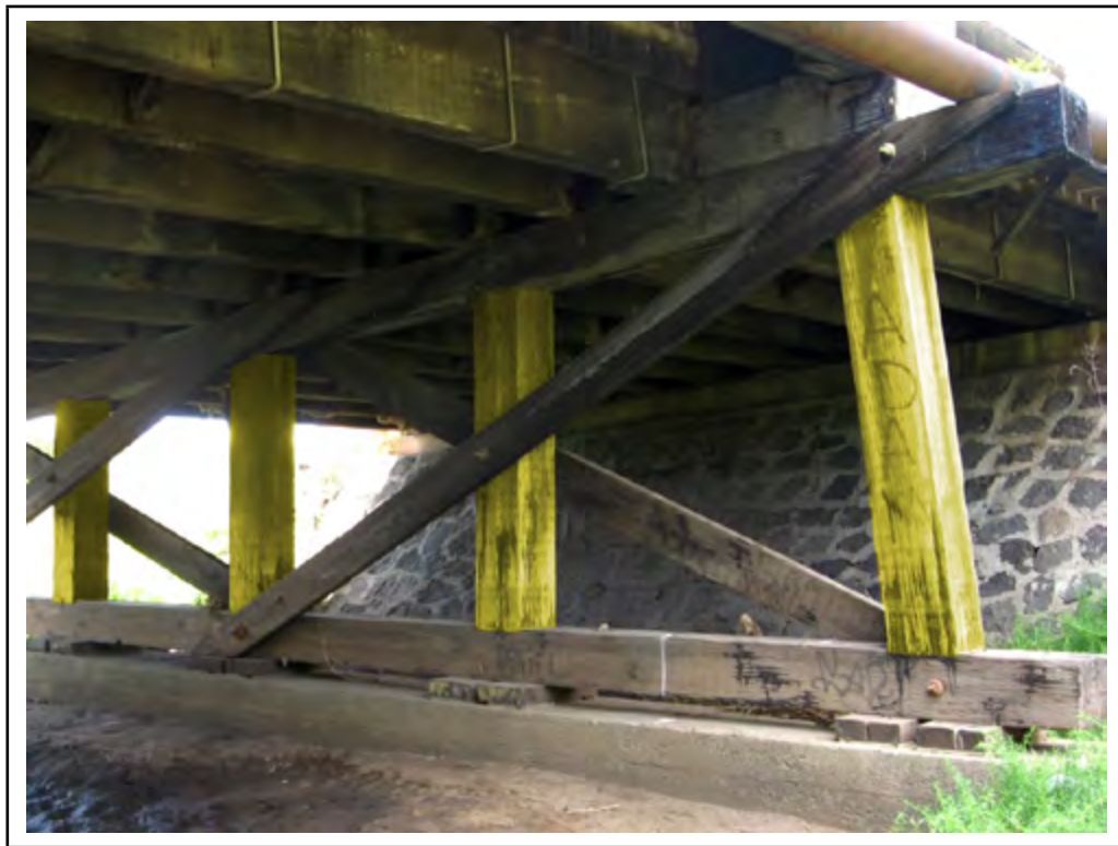
Photo: Element 206 - Timber Column (Highlighted)
