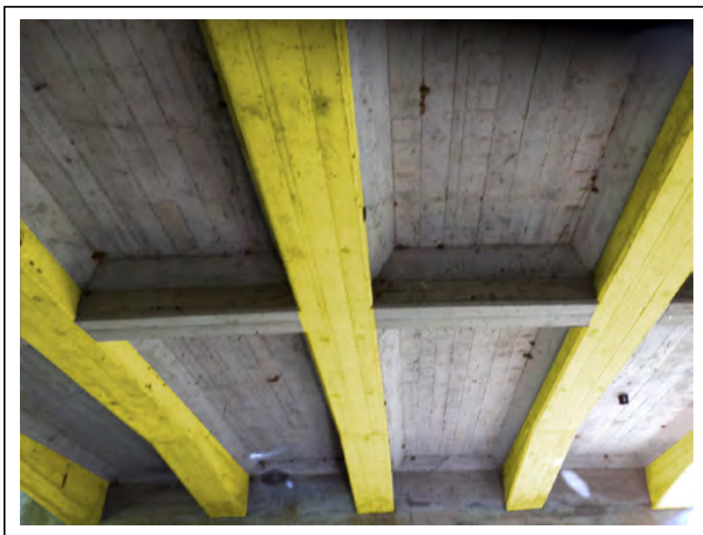
Photo: Element 110 - Reinforced Concrete Open Girder / Beam (Highlighted)
