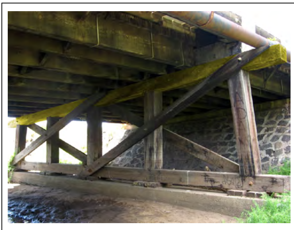
Photo: Element 235 - Timber Pier Cap (Highlighted)
