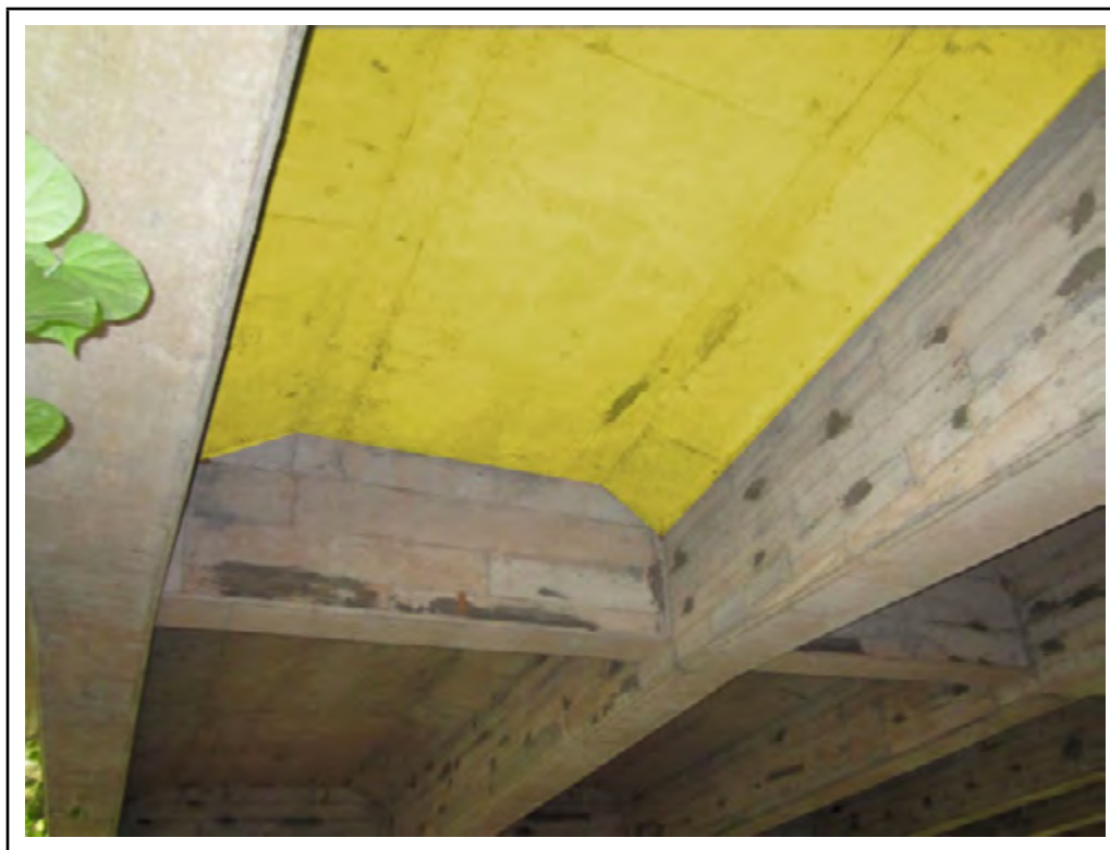
Photo: Element 16 - Reinforced Concrete Top Flange (Highlighted)
