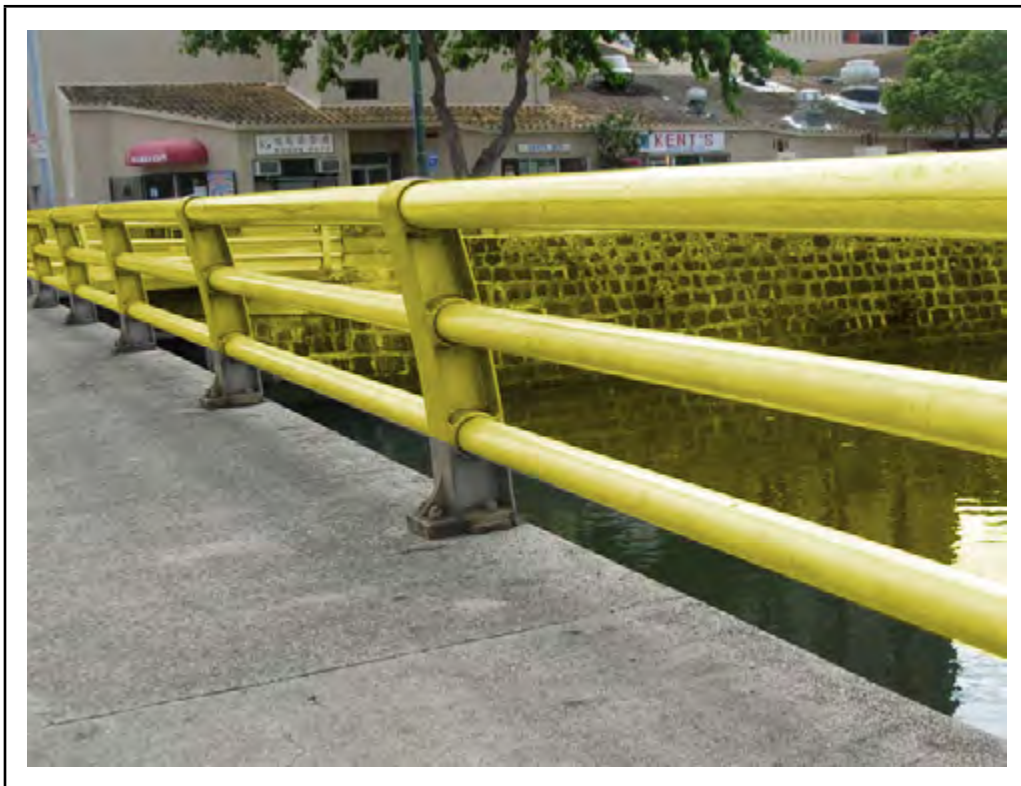
Photo: Element 330 - Metal Bridge Railing (Highlighted)
