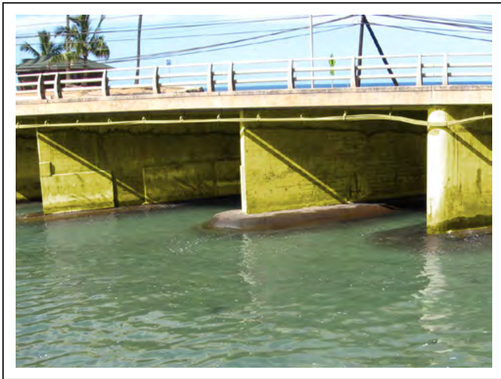
Photo: Element 210 - Reinforced Concrete Pier Wall (Highlighted)
