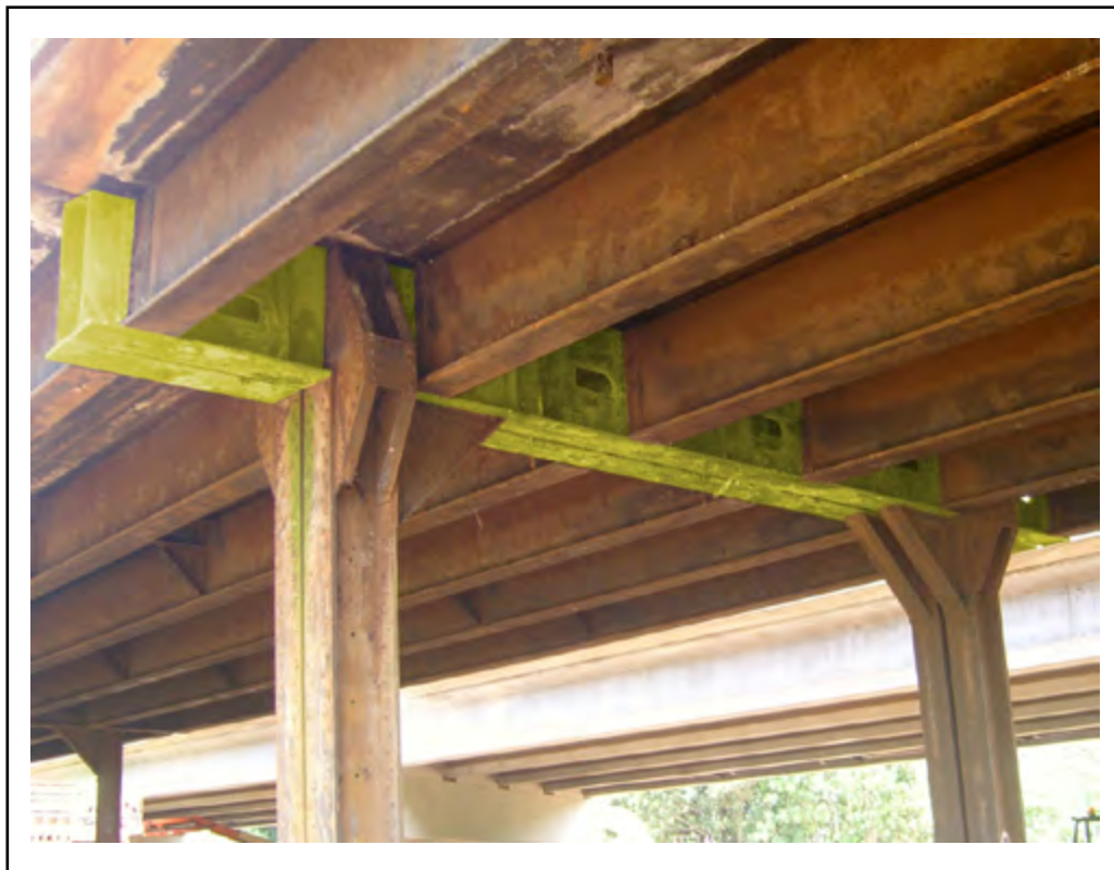
Photo: Element 231 - Steel Pier Cap (Highlighted)
