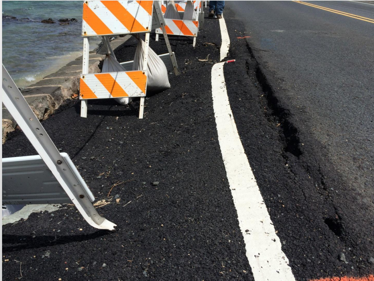
Continual Pavement Cracking along Lane Line
