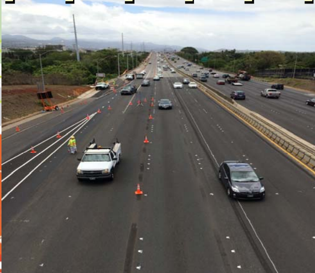
H1 Facing Westbound lanes
