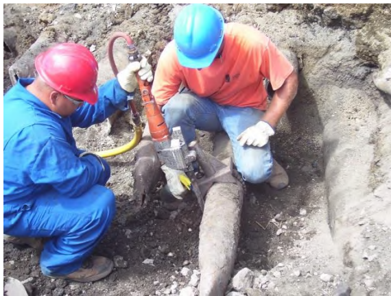
Workers tapping and draining abandoned pipelines
