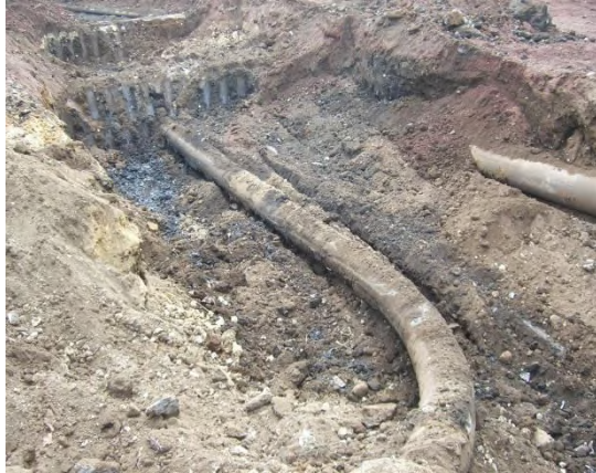
Exposed abandoned pipelines
