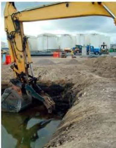
Example of large-scale excavation
