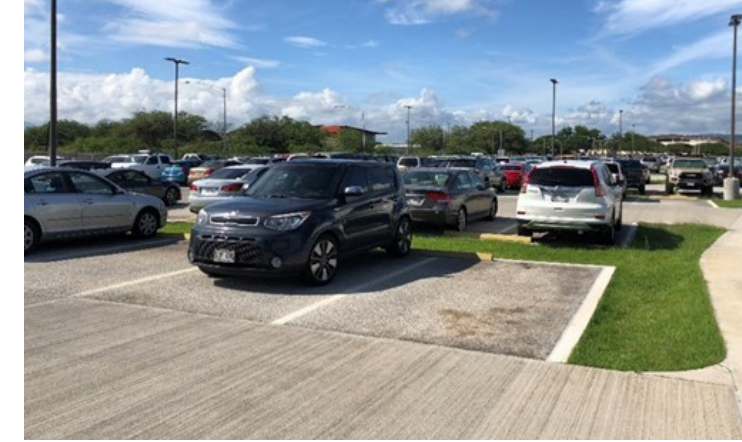
Elliott Street Parking Lot Permeable Pavement, Daniel K. Inouye International Airport Source: Hawaii DOTA
