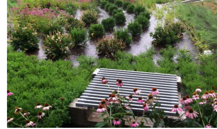
Bioretention Source: https://www.epa.gov/system/files/documents/2021-11/bmp-bioretention-rain-gardens.pdf
