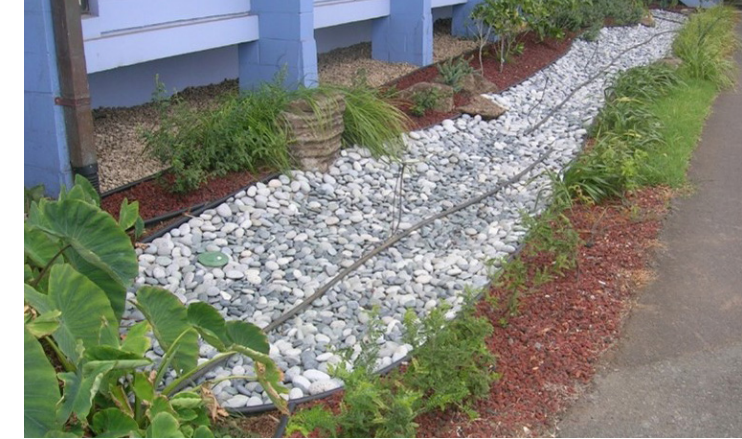
Infiltration Trench at Kakoi Baseyard, Oahu Source: HDOT Highways Division
