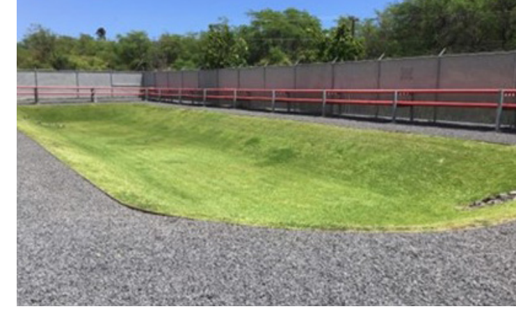
Infiltration Basin, Kahului Airport Source: Hawaii DOTA
