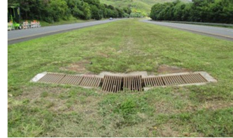
Vegetated Swale along H-3, Oahu Source: HDOT Highways Division
