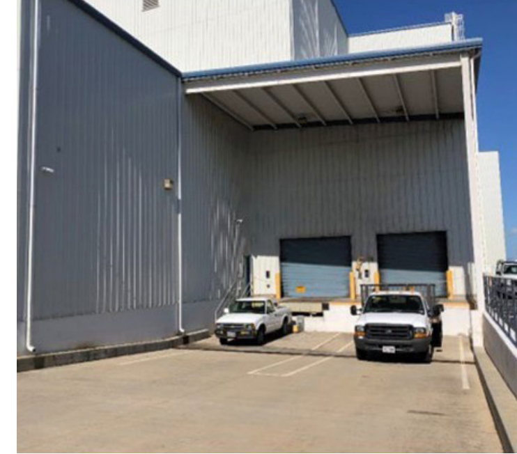
Loading Area at Cargo Facility, Daniel K. Inouye International Airport Source: Hawaii DOTA
