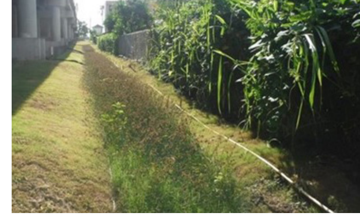
Vegetated Buffer Strip, Oahu Source: HDOT Highways Division
