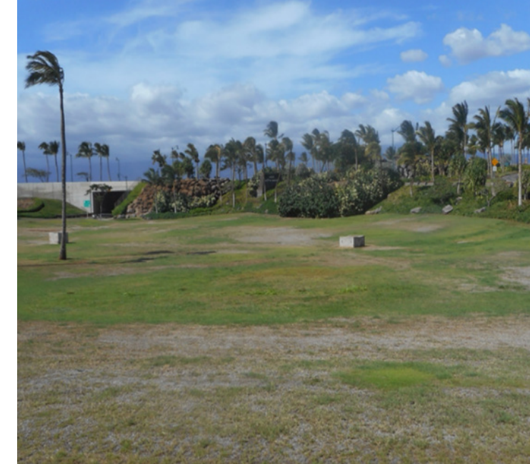
Detention Basin at Kahului Airport Source: Hawaii DOTA
