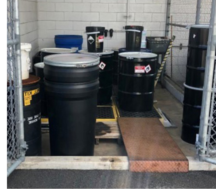
Material Storage Area with a Containment Berm at Hangar, Daniel K. Inouye International Airport Source: Hawaii DOTA
