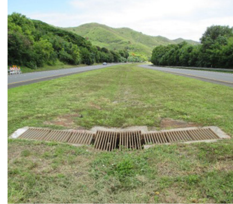
Vegetated Swale along H-3, Oahu Source: HDOT Highways Division
