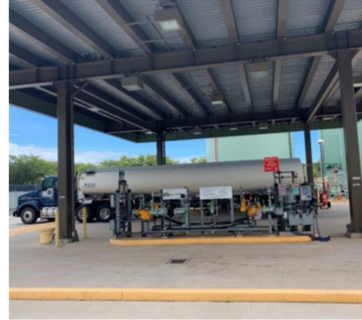
Jet Fuel Loading Rack at Fueling Facility, Kahului Airport Source: Hawaii DOTA
