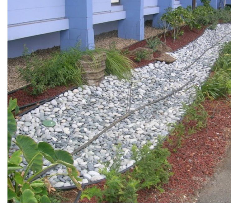
Infiltration Trench at Kakoi Baseyard, Oahu Source: HDOT Highways Division
