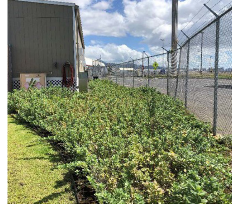
Bioswale at Terminal 3 Parking Lot, Daniel K. Inouye International Airport Source: Hawaii DOTA
