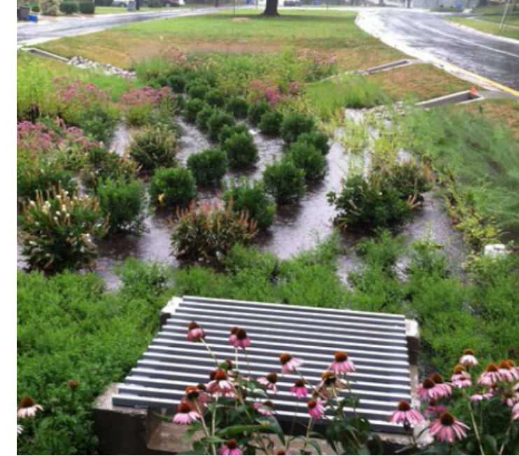
Bioretention Source: https://www.epa.gov/system/files/documents/2021-11/bmp-bioretention-rain-gardens.pdf
