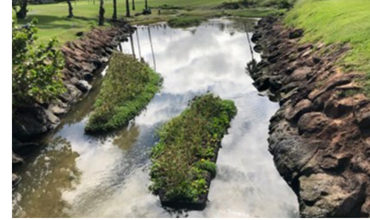
Floating Wetland in Kaanapali Lagoon, Maui Source: West Maui Ridge 3 Reef Initiative
