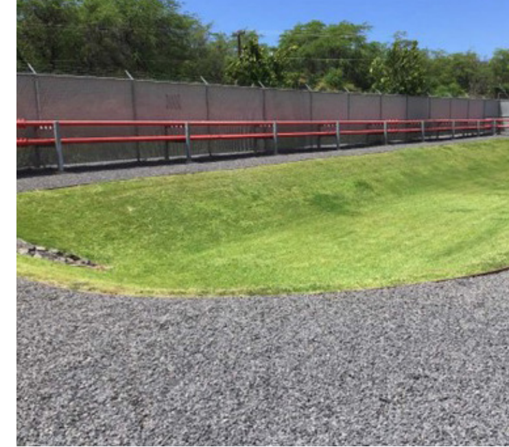
Infiltration Basin, Kahului Airport Source: Hawaii DOTA
