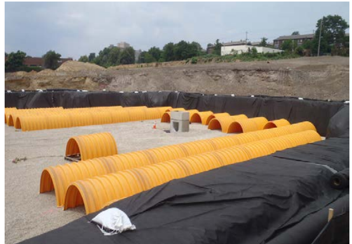
Subsurface Detention Installation, Philadelphia Source: Philadelphia Stormwater Management Guidance Manual, Version 3.2
