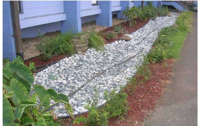
Bioretention at Kakoi Baseyard, Oahu Source: HDOT Highways Division
