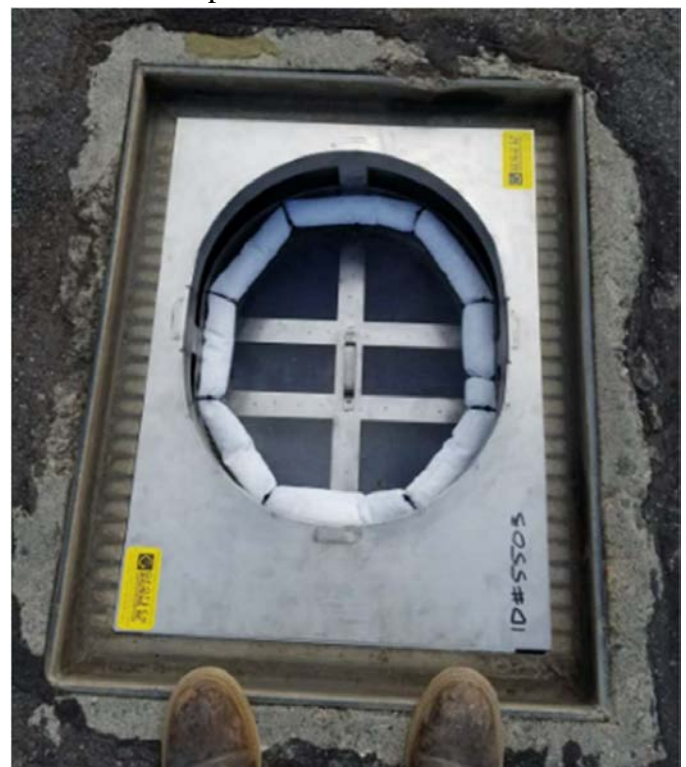
Example of Bio Clean Grate Inlet Media Filter at Daniel K. Inouye Airport Maintenance Baseyard
