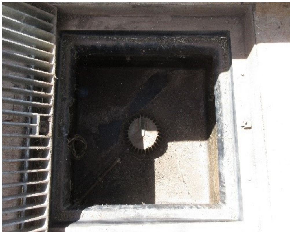
Oil water separator at the DOTA Wash Rack, Kahului Airport
