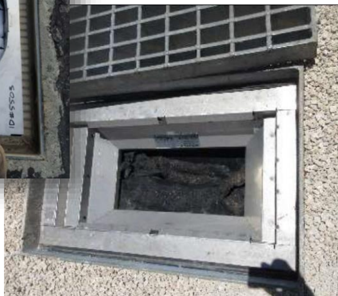
Drain Inlet Insert at Maintenance Baseyard (left) and Drain Inlet Insert at Elliott Street Parking Lot (right), Daniel K. Inouye International Airport
