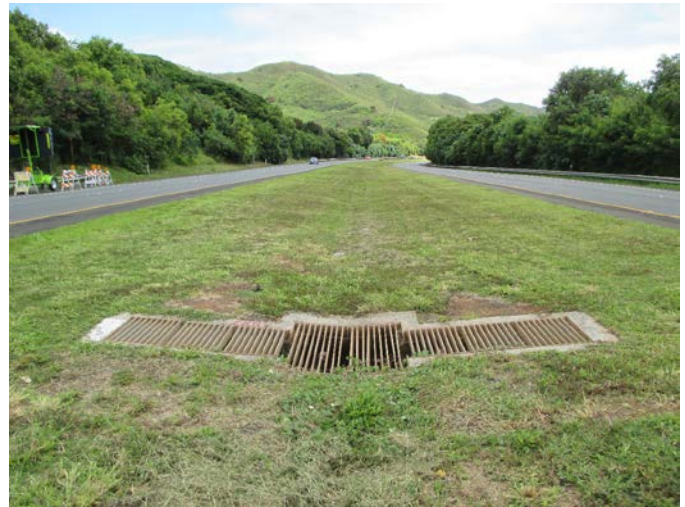
Vegetated Swale along H-3, Oahu Source: HDOT Highways Division
