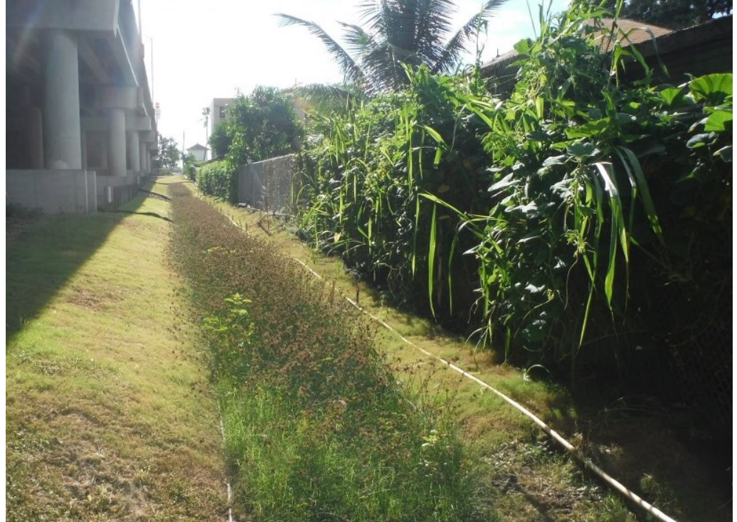
Vegetated Buffer Strip, Oahu Source: HDOT Highways Division
