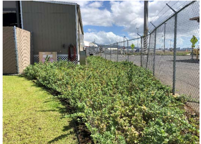
Bioswale at Terminal 3 Parking Lot
