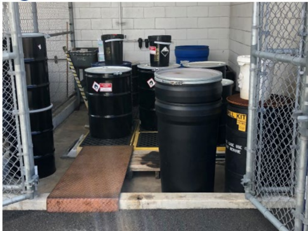
Material Storage Area with a Containment Berm at a Hangar, Daniel K. Inouye International Airport
