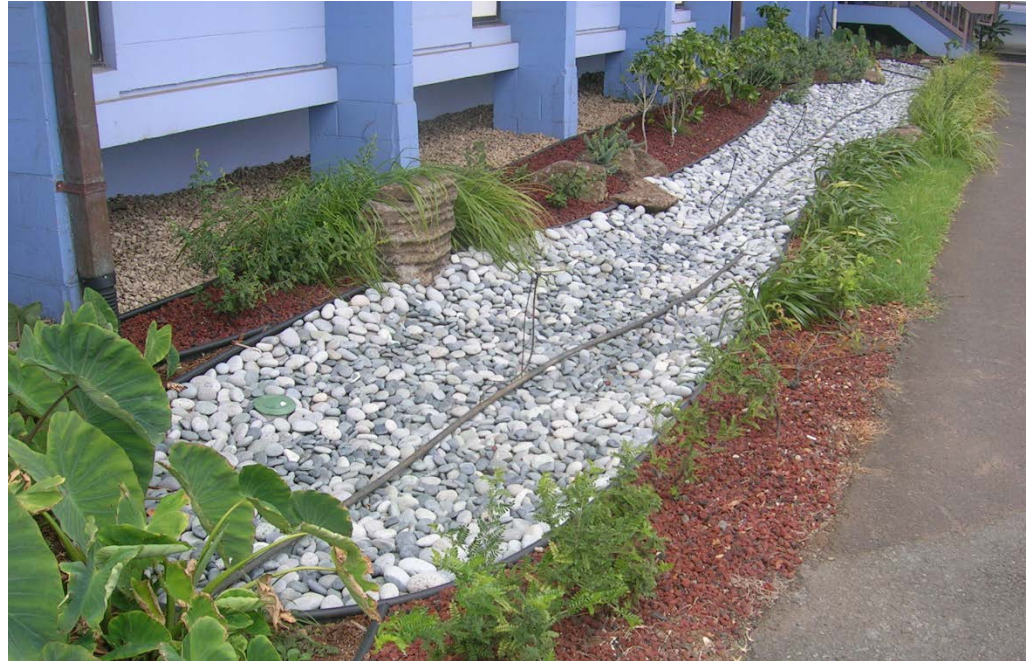
Bioretention at the Kakoi Baseyard, Oahu
