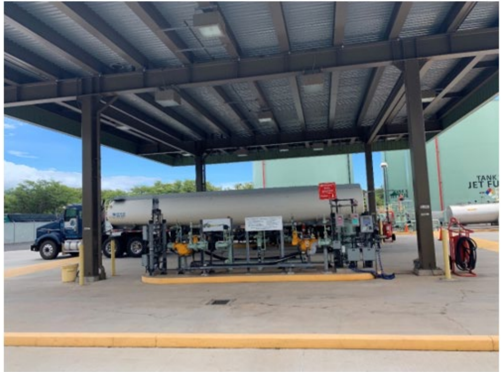
Jet Fuel Loading Rack at a Fueling Facility, Kahului Airport
