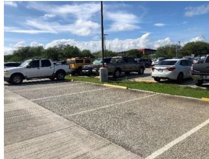
Permeable pavement and grass swale at HNL Elliott Street parking lot
