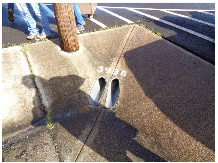
Photograph 47: Drain inlet EID 3908, an opening in the Concrete Channel.
