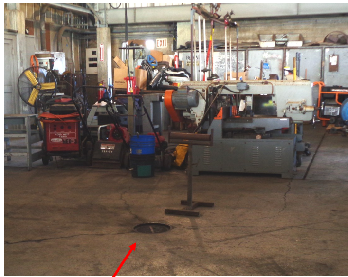
Photograph 7: Floor drain in the Maintenance Shop that goes to the oil water separator (3907).
