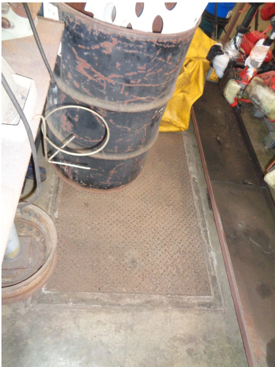
Photograph 6: 100-gallon oil water separator (3907) in the Maintenance Shop.
