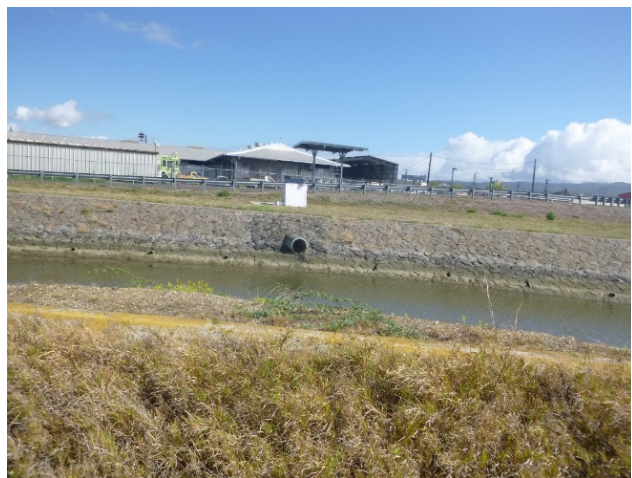
FIGURE 1: Outfall 4576 on June 1, 2015. Photo taken at 9:15 a.m. during low tide. The high tide water marks are visible above the outfall.
