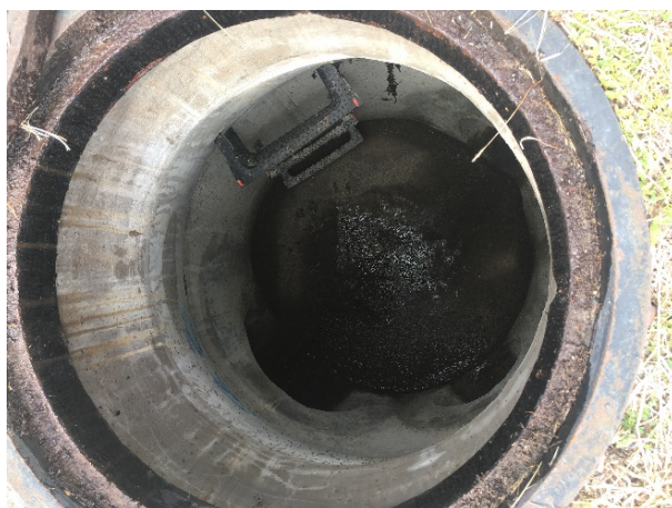
FIGURE 4: Manhole 5501 on March 26, 2018. Photo taken at 11:40 a.m. during high tide. There is no standing water.
