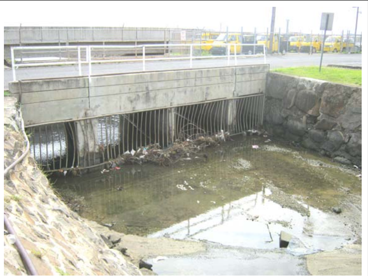
Photograph 32: Drainage canal along the eastern boundary of the Maintenance Baseyard. Bridge provides access to the main gate. Salvage vehicles are stored on the other side of the bridge.
