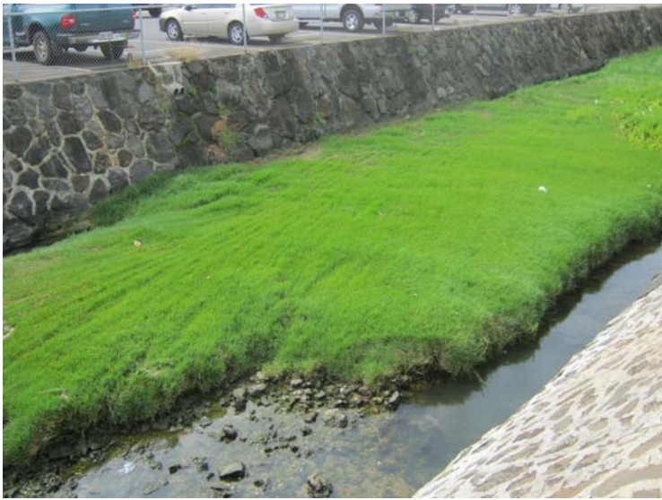
Photograph 31: Drainage ditch along the eastern boundary of the Maintenance Baseyard, adjacent to Aolele Street.
