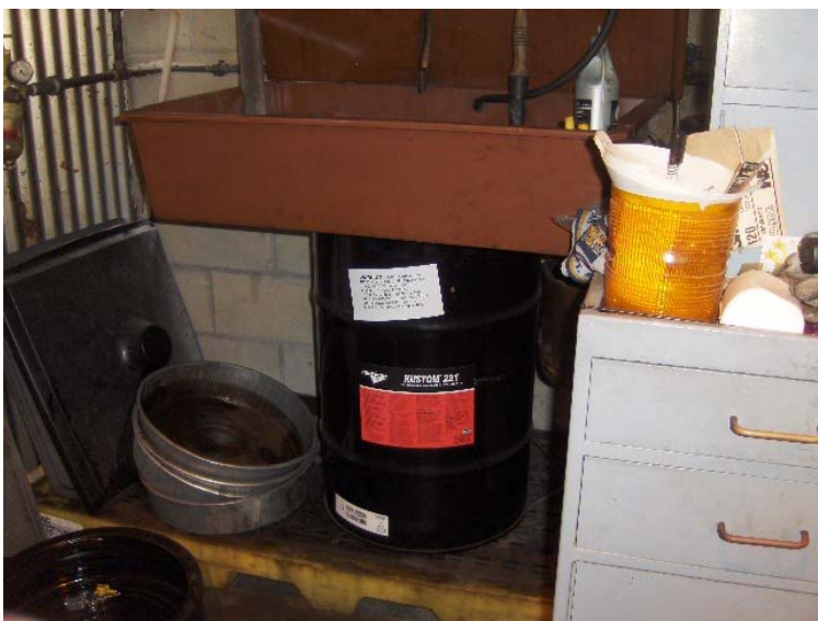
Photograph 6: Parts washer on secondary containment in the maintenance shop.
