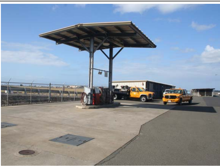
Photograph 12: Covered fueling Area.
