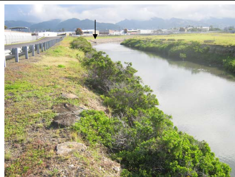
Photograph 33: Kaloaloe Canal on the southern side of the Maintenance Baseyard. Monitoring Point HNL 003 identified by arrow.
