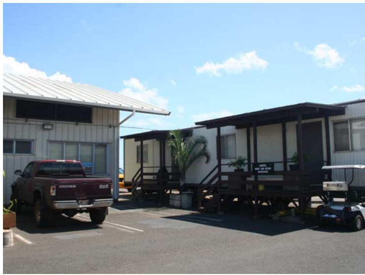
Photograph 22: Office trailers in the northern portion of the Maintenance Baseyard.
