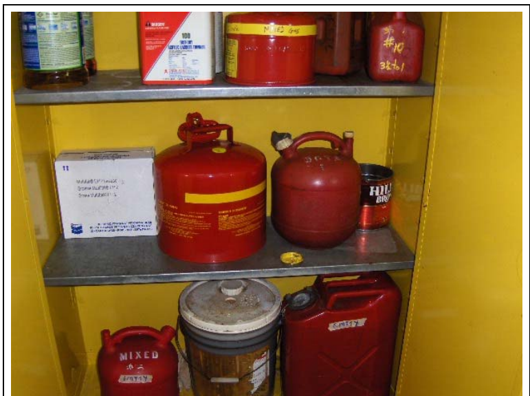
Photograph 17: Flammable storage locker in the Warehouse area.
