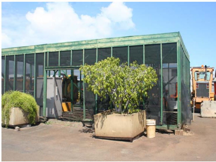
Photograph 19: Greenhouse area near the Carpentry Shop.
