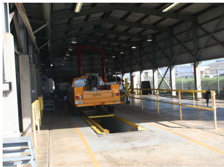
Photograph 3: Interior of the maintenance bay and vehicle washing area inside of the maintenance shop.
