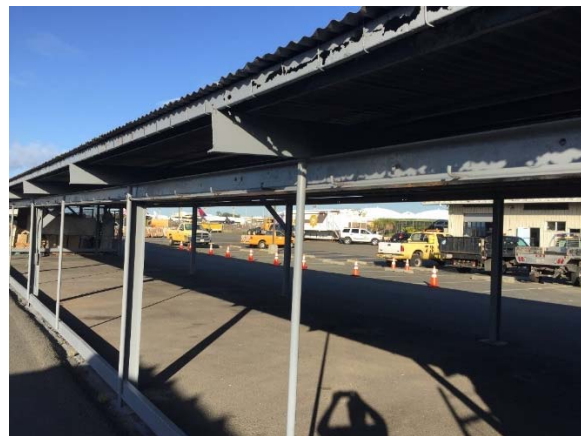
FIGURE 2. COVERED PARKING STRUCTURE MITIGATED (MARCH 27, 2019). Metal surfaces painted with corrosion inhibiting paint. Corroded fencing removed. Rust flakes on the ground swept up.
