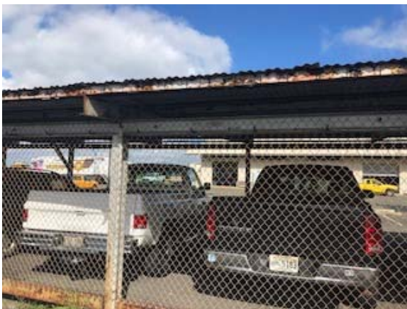
FIGURE 1. RUSTY COVERED PARKING STRUCTURE (MARCH 13, 2019).
