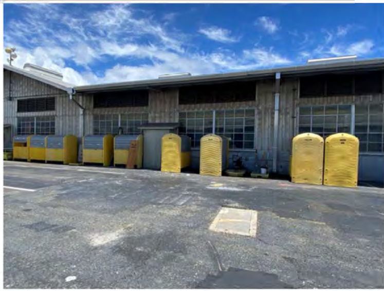
Photograph 31: Paint Storage area, with drums of paints stored inside of the yellow UltraTech® 9613 outdoor spill containment pallets, and Hazardous Material Storage on secondary containment.
