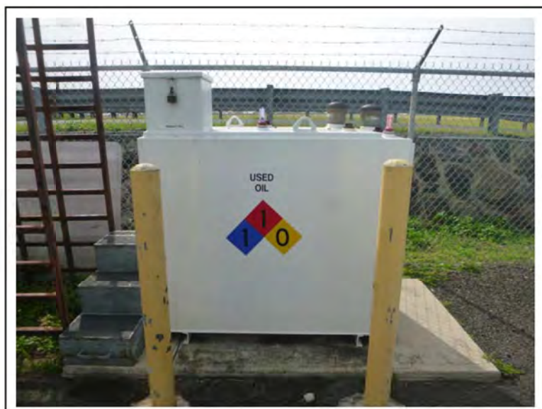
Photograph 11: 280-gallon used oil AST (EID 09372) near the Fueling Area.
