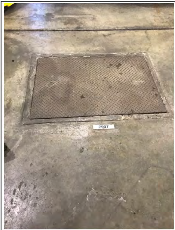
Photograph 6: 100-gallon oil water separator (3907) in the Maintenance Shop.
