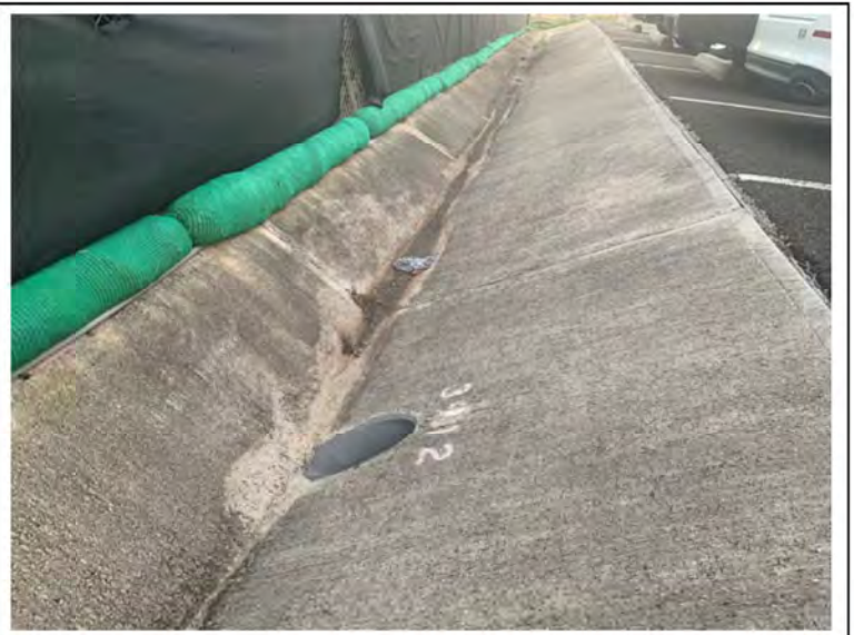
Photograph 50: Drain inlet EID 3912, an opening in the Concrete Channel.
