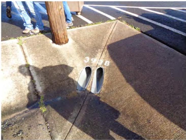
Photograph 49: Drain inlet EID 3908, an opening in the Concrete Channel.
