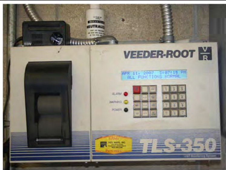
Photograph 21: Veeder-Root monitoring system for the underground storage tanks.
