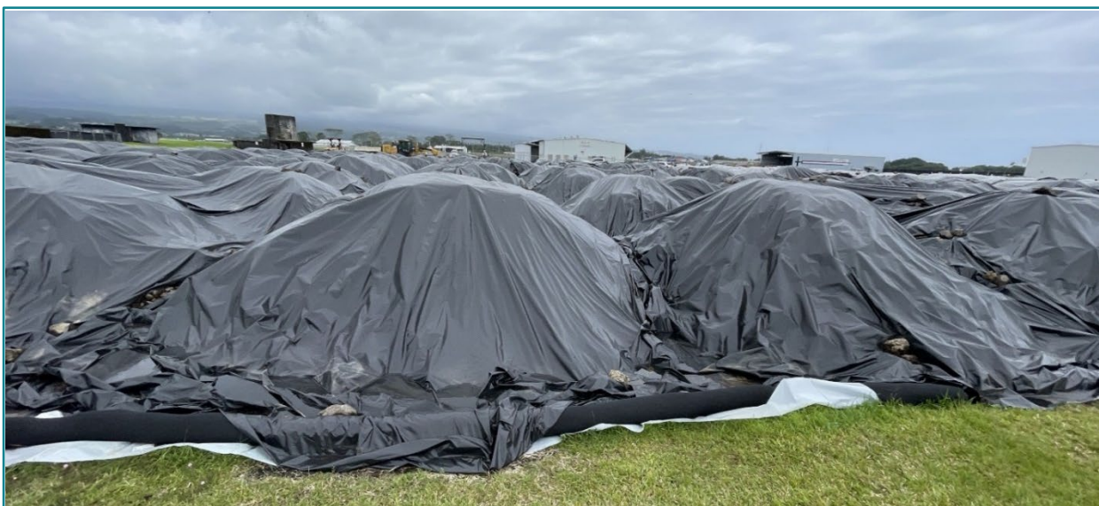
Properly Managed Soil Stockpiles are Constructed on a Liner with Berm and a Cover
