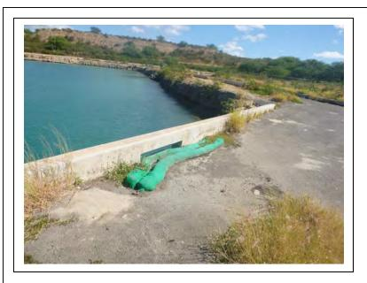
Photograph 35: Concrete edge protection and scour at the end of Pier 7.
