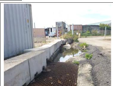
Photograph 8: SDD7615 Concrete barrier displaced.
