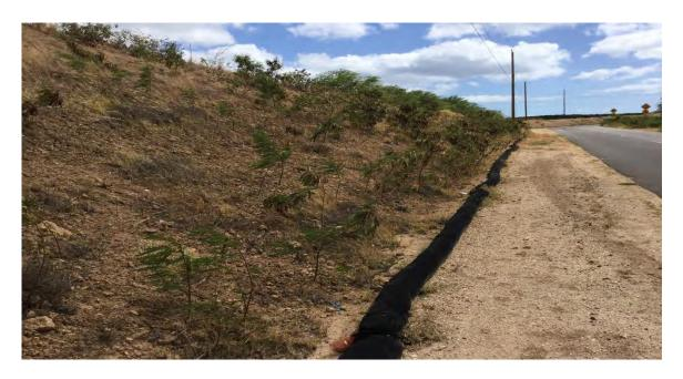
Figure 6 – Mauka slope of Stockpile 2B with biosock BMP looking west.
