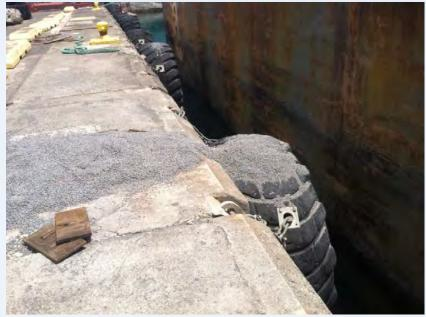
Uncontained materials over a trench drain and near pier's edge.
