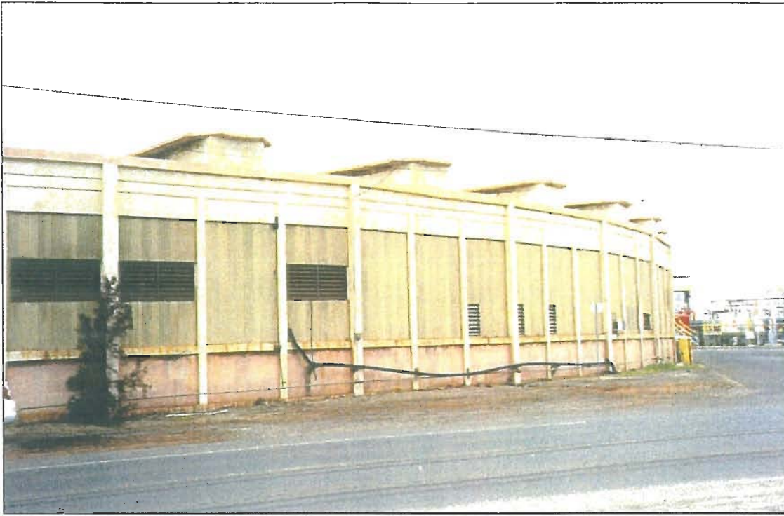
Photo 5. Site 1607 former Kahului Railroad roundhouse.
