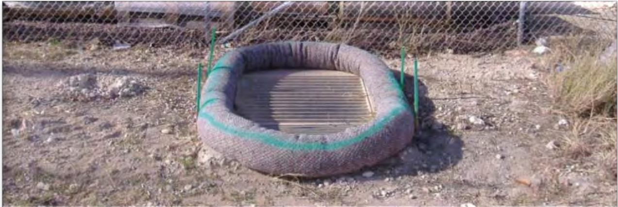
Drain Inlet Control, Barbers Point. January 2006.
