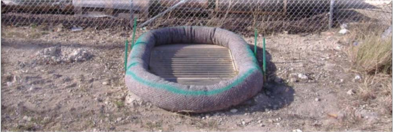
Drain Inlet Control, Barbers Point. January 2006.
