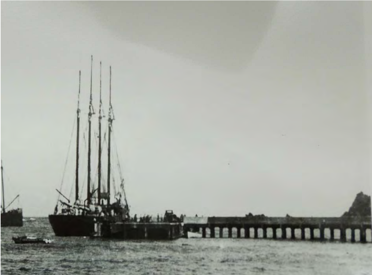
No structures on Pier yet.
