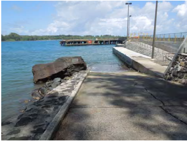
Photo 8. Hāna Pier Ramp Area
