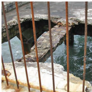
5. Topside view of pier deck hole in Photo 4.
