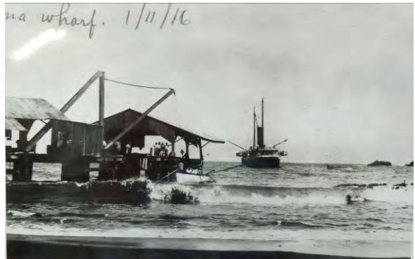
Photo 33. Vessel waiting off of old Wharf.
