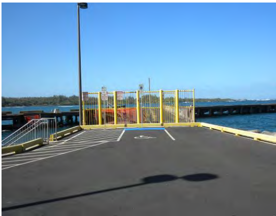
Photo 64. Entrance to pier 2-28-13
