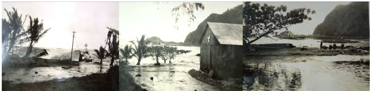
Photos 46-48. Aftermath of April 1, 1946 Tsunami on shore of Hāna Bay; Structure on Pier deck still intact.
