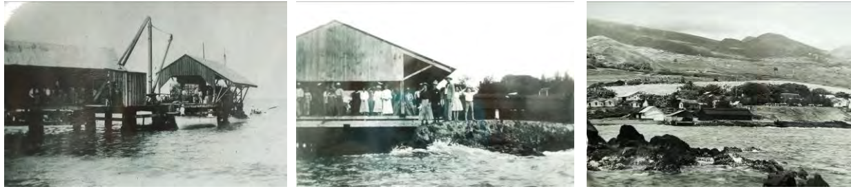
Photos 37-39. Old Wharf in Hāna Bay destroyed in the early 1900s.
