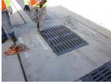
Photo 3.3.53 **PBMP 3.3** Pier 29 Inlet & Trench Drain Filters
