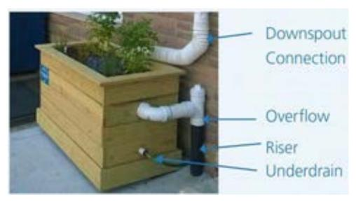
Figure 3-8 Downspout Planter Box<sup>5</sup>
