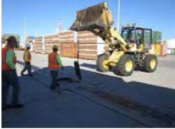
Photo 3.3.13 **PBMP 3.3** Pier 29 Inlet & Trench Drain Filters
