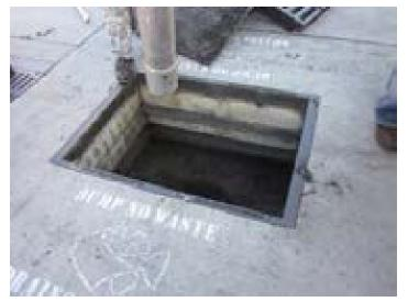
Photo 3.3.44 **PBMP 3.3** Pier 29 Inlet & Trench Drain Filters
