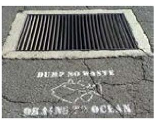
**Photo 8 Description:** Stenciling by all drain inlets prevents illicit discharges. These are maintained by DOT-Harbors personnel.
