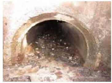
Photo 3.1.54 **PBMP 3.1** Pier 35 Grated Inlet Skimmer Box
