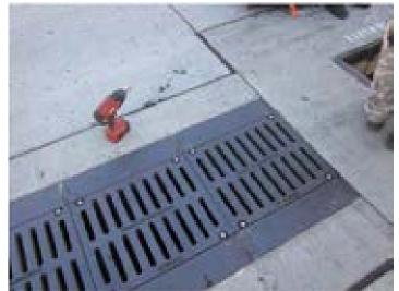
Photo 3.3.21 **PBMP 3.3** Pier 29 Inlet & Trench Drain Filters
