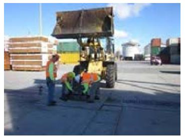
Photo 3.3.48 **PBMP 3.3** Pier 29 Inlet & Trench Drain Filters
