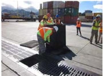
Photo 3.3.85 **PBMP 3.3** Pier 29 Inlet & Trench Drain Filters
