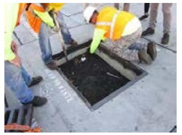
Photo 3.3.20 **PBMP 3.3** Pier 29 Inlet & Trench Drain Filters
