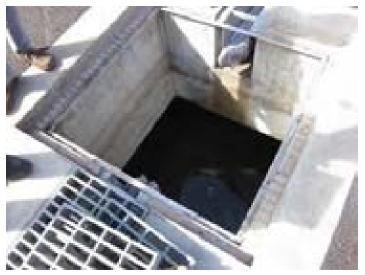
Photo 3.1.63 **PBMP 3.1** Pier 35 Trench Drain
