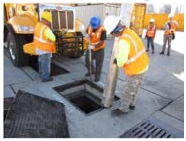
Photo 3.3.38 **PBMP 3.3** Pier 29 Inlet & Trench Drain Filters
