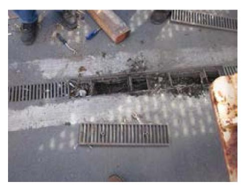
Photo 2 shows a close-up view of occluded filtration media and accumulated sediment within trench drain at Pier 31.
