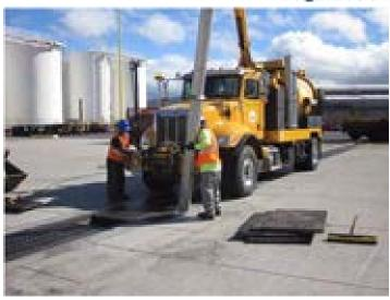
Photo 3.3.98 **PBMP 3.3** Pier 29 Inlet & Trench Drain Filters
