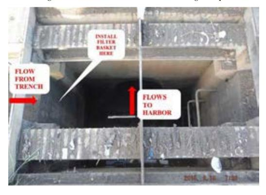
Figure 3-18 SDO8906 Trench Drain Discharge to Pipe
