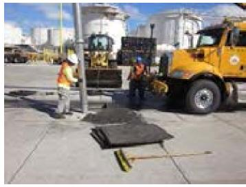
Photo 3.3.94 **PBMP 3.3** Pier 29 Inlet & Trench Drain Filters
