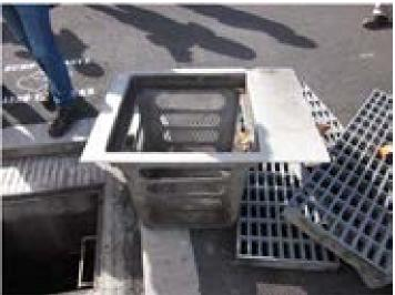
Photo 3.1.21 **PBMP 3.1** Pier 35 Grated Inlet Skimmer Box
