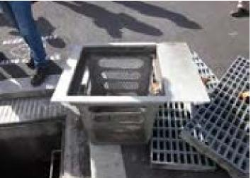
Photo 3.1.21 **PBMP 3.1** Pier 35 Grated Inlet Skimmer Box
