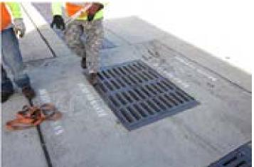
Photo 3.3.53 **PBMP 3.3** Pier 29 Inlet & Trench Drain Filters
