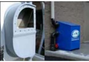
The existing BMPs in SDO4401, SDO4405, SDO4397, SDO4401, SDO4393, SDO4395, SDO4399 are effective at removing pollutants from runoff, but maintenance of the BMPs does not work. The design of the existing BMPs called for replacement of the absorbent pouches by pulling them out from the perforated housing pipe, but when the BMP is fully loaded with sediment, it is impossible to remove the pouches. Even after removing the accessible sediment from the BMP, the pouches were still not removable.
