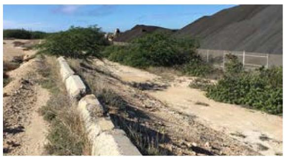
Figure 11: Pile butts on the perimeter of Stockpile 5 and drainage/retention basis along western slope.
