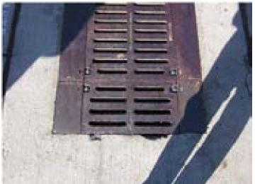
Photo 3.3.9 **PBMP 3.3** Pier 29 Inlet & Trench Drain Filters
