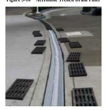
Figure 3-10 Accessible Trench Drain Filter
