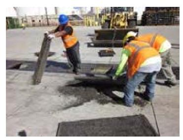
Photo 3.3.87 **PBMP 3.3** Pier 29 Inlet & Trench Drain Filters
