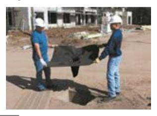
Figure 3-14 Ultra-Drain Guard Filter<sup>9</sup>
