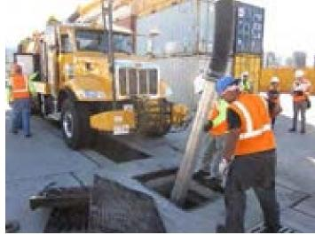
Photo 3.3.41 **PBMP 3.3** Pier 29 Inlet & Trench Drain Filters
