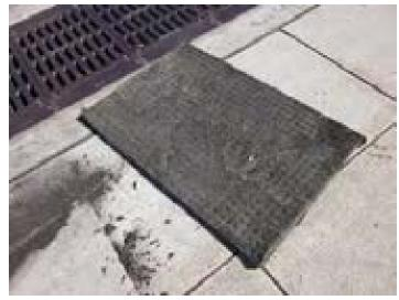
Photo 3.3.82 **PBMP 3.3** Pier 29 Inlet & Trench Drain Filters
