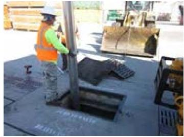
Photo 3.3.42 **PBMP 3.3** Pier 29 Inlet & Trench Drain Filters
