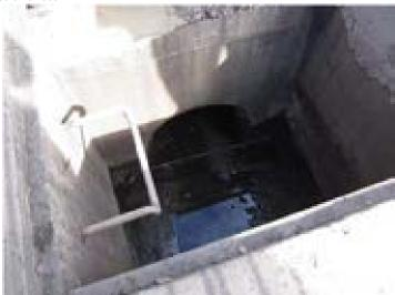
Photo 3.1.25 **PBMP 3.1** Pier 35 Grated Inlet Skimmer Box
