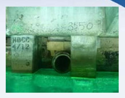
Designed to carry untreated stormwater directly into the Harbor
