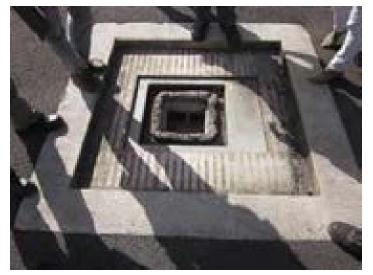
Photo 3.1.12 **PBMP 3.1** Pier 35 Grated Inlet Skimmer Box
