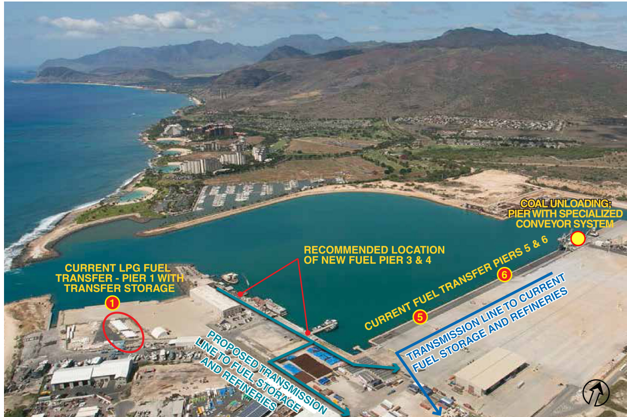
Figure 2. Fuel Pipelines, KBPH
