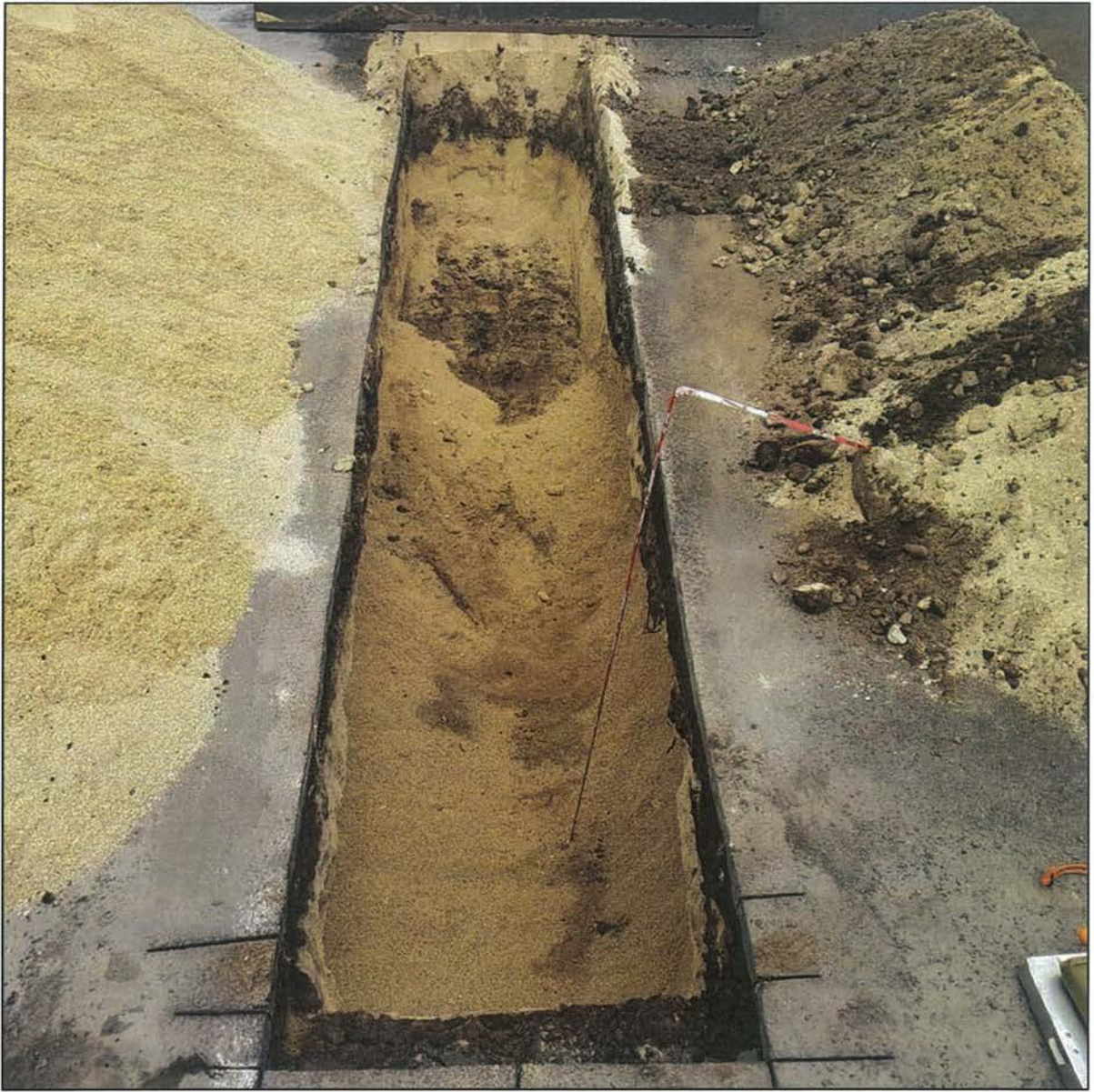
Figure 6: Photographic Overview of Stratigraphic Trench 1. View to North.
