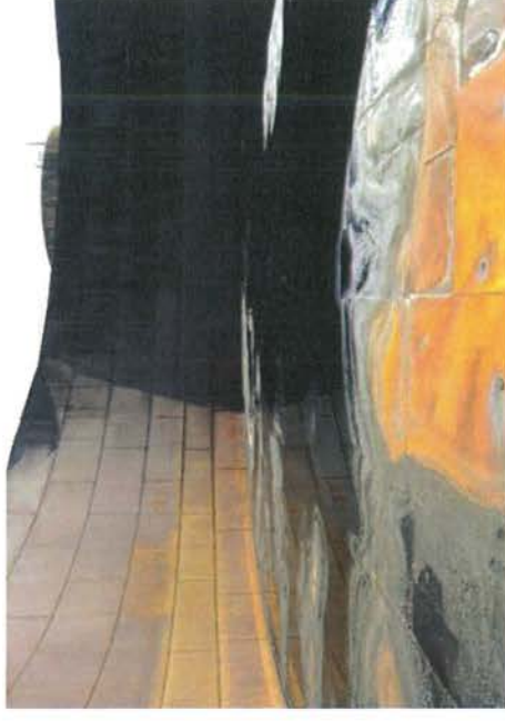
Figure 6: Interior of Molasses Storage Tank (3)
