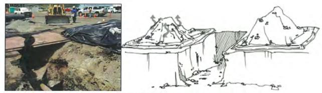
Oil might seep from the side of an excavation and cause an oil sheen. It may be necessary to manage the oily water.
