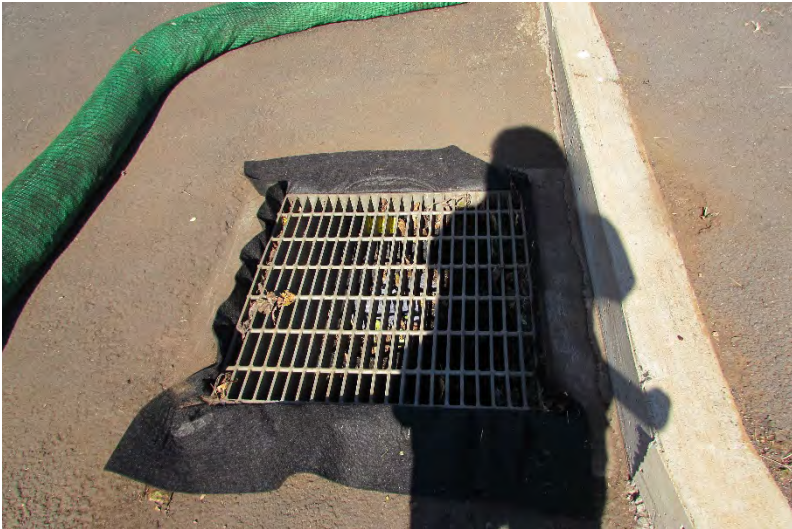
HWY-M Photo 5.2.118 Grated Drain Inlet
