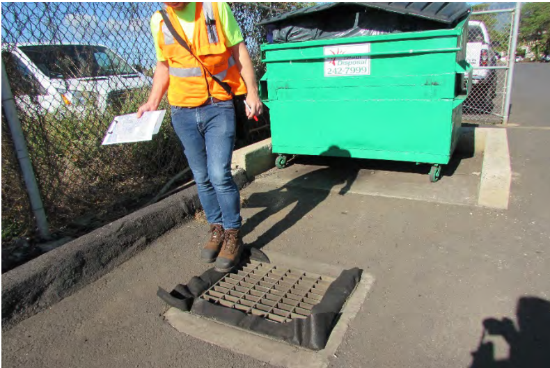
HWY-M Photo 5.2.31 Grated Drain Inlet/Dry Well
