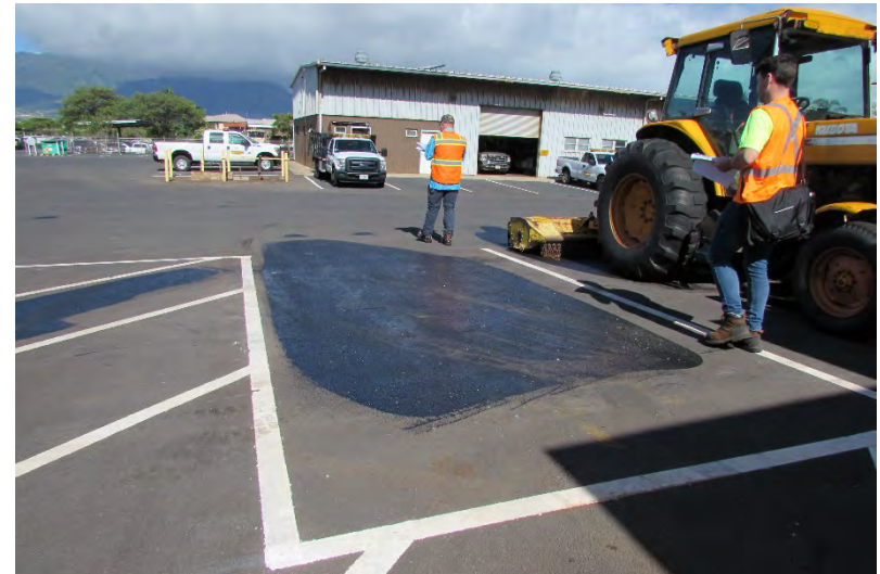
HWY-M Photo 5.2.143 Equipment Parking Area Asphalt Seal
