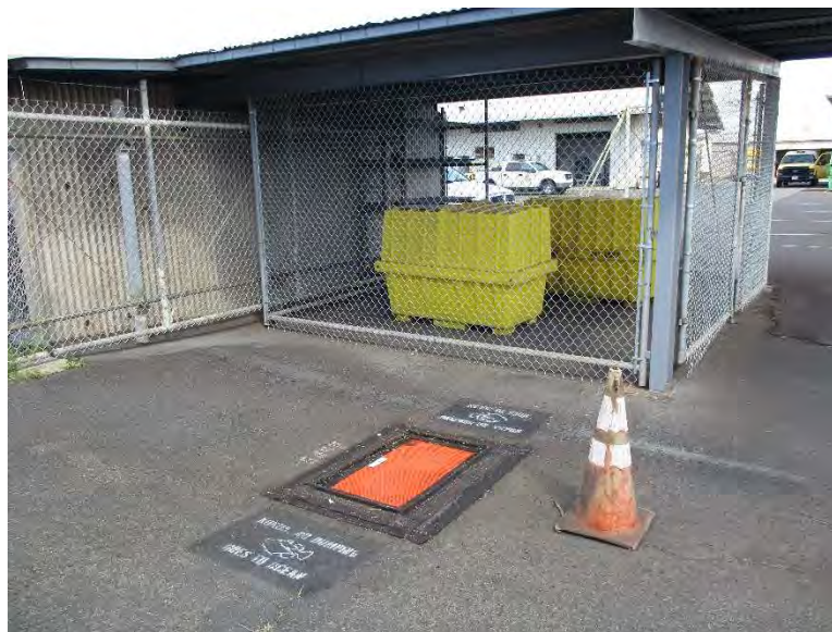
Figure 5. GR8 Guard Drain Protector Mat at Drain Inlet EID 5499.
