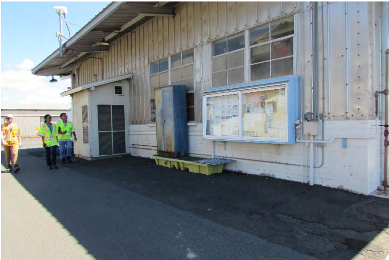
AIR-EE Photo 2.1.167 Chemical Storage Cabinet on Secondary Containment
