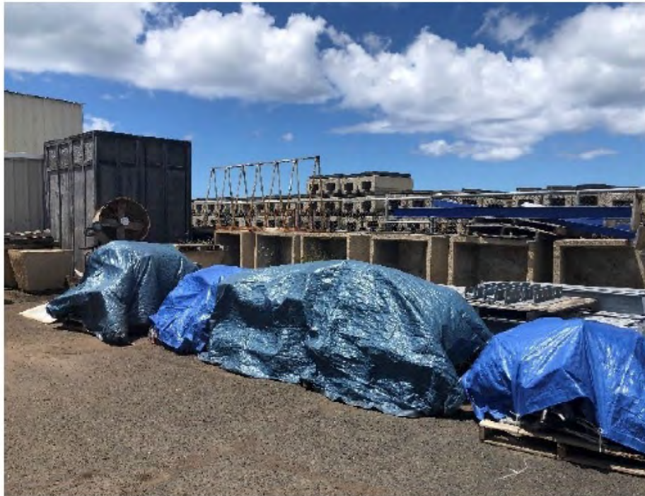
Figure 1. Metal materials (already stored on dunnage) covered with tarp.
