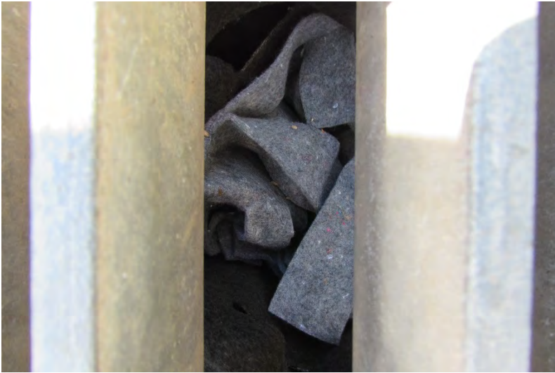
HWY-O Photo 6.1.117 Storm Drain Inlet With BMP
