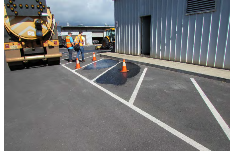
HWY-M Photo 5.2.141 Equipment Parking Area Asphalt Seal
