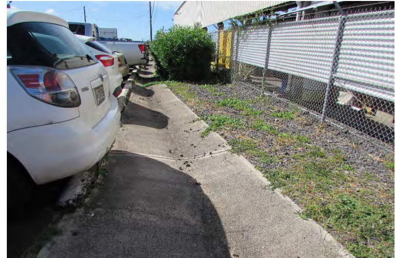
AIR-EE Photo 2.1.12 Concrete Channel near Employee Parking Area
