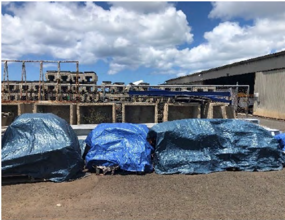
Figure 2. Another view of the metal materials covered and on dunnage.
