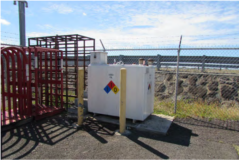
AIR-EE Photo 2.1.41 Used Oil AST
