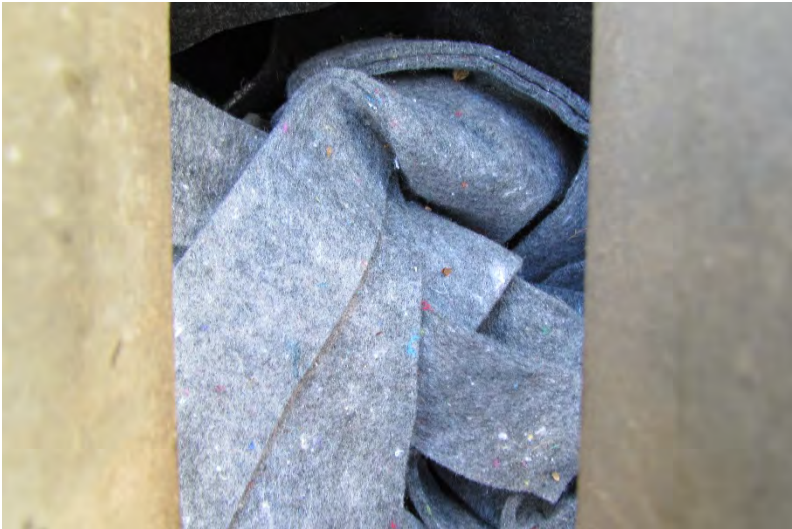
HWY-O Photo 6.1.115 Storm Drain Inlet With BMP
