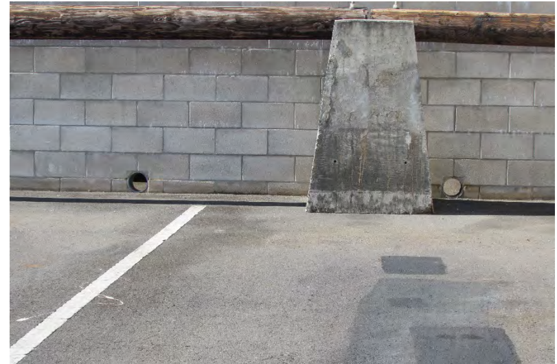
HWY-O Photo 6.1.54 Openings in South CMU Wall
