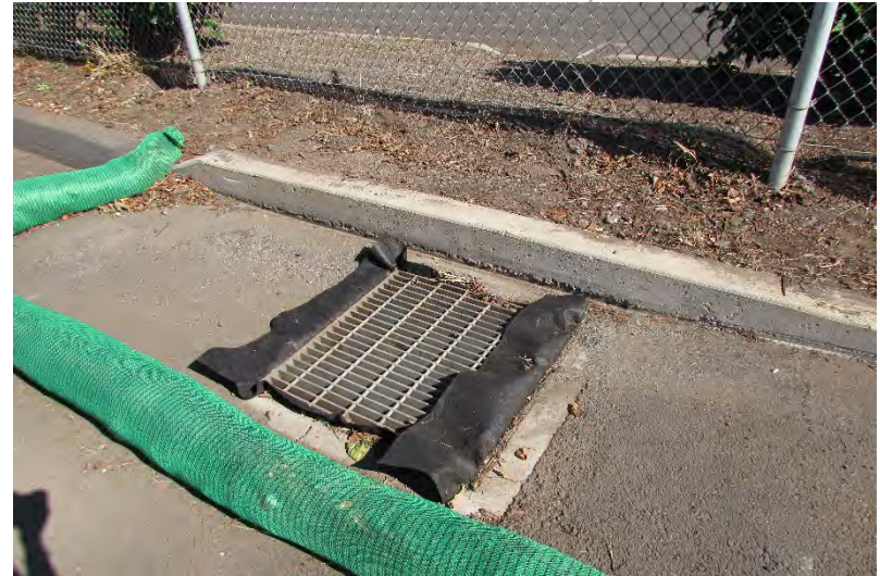
HWY-M Photo 5.2.106 Grated Drain Inlet
