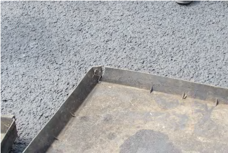
HWY-O Photo 6.2.15 Drip Pan in Disrepair
