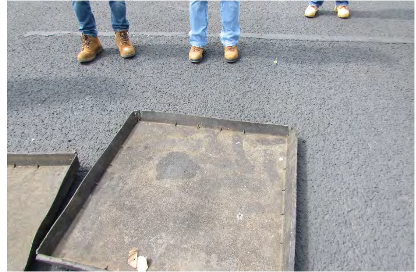
HWY-O Photo 6.2.14 Drip Pan in Disrepair
