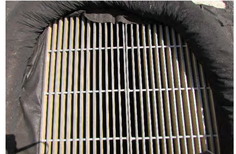
HWY-O Photo 6.2.66 Drain Inlet with BMP (Southern)
