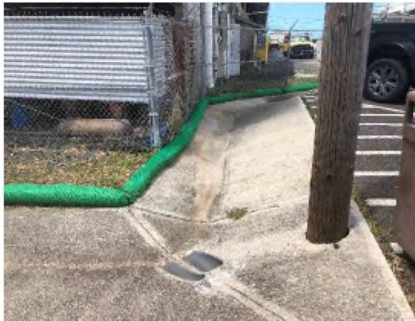
Figure 1. Debris cleaned out and filter sock placed along the concrete channel.
