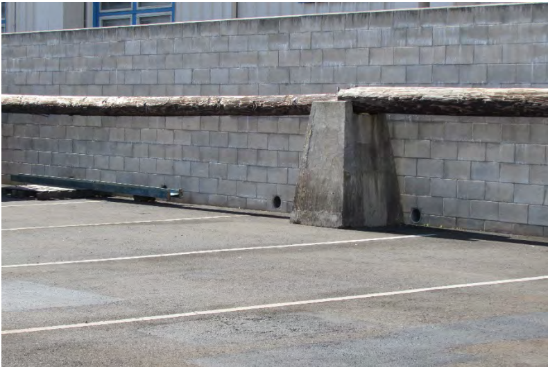
HWY-O Photo 6.1.55 Openings in South CMU Wall
