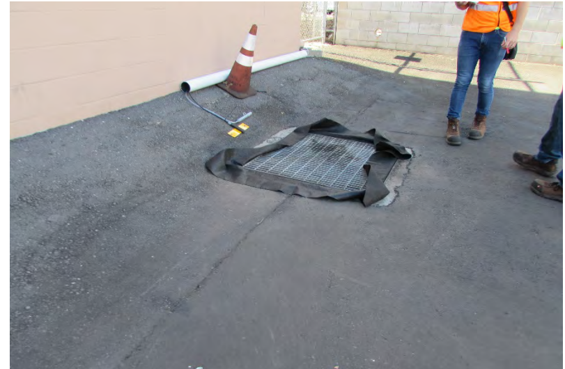
HWY-O Photo 6.1.34 Sampling Point Storm Drain Inlet with BMP
