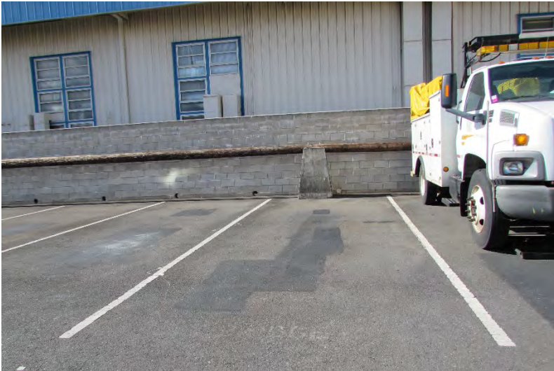
HWY-O Photo 6.1.53 Openings in South CMU Wall
