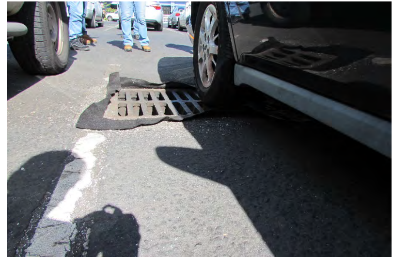
HWY-O Photo 6.1.124 Storm Drain Inlet With BMP
