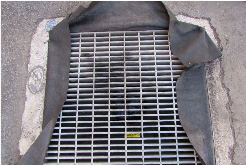
HWY-O Photo 6.1.35 Storm Drain Inlet with BMP
