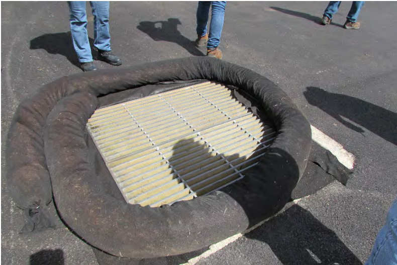
HWY-O Photo 6.2.65 Drain Inlet with BMP (Southern)
