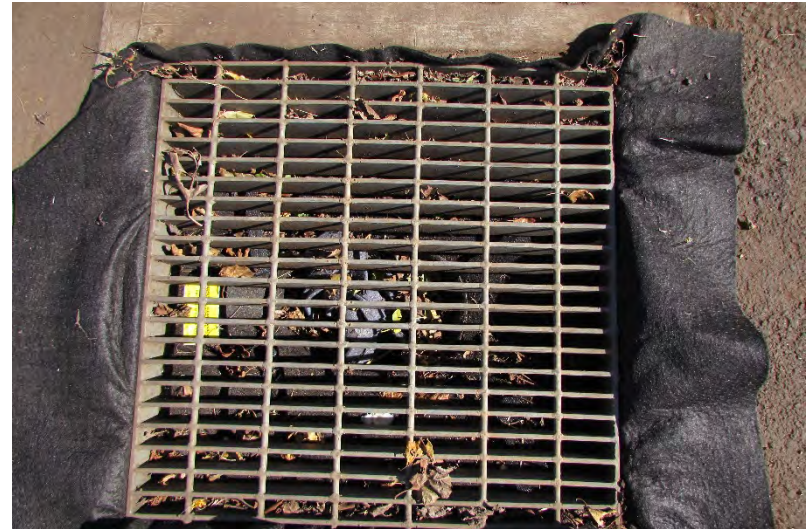
HWY-M Photo 5.2.119 Grated Drain Inlet
