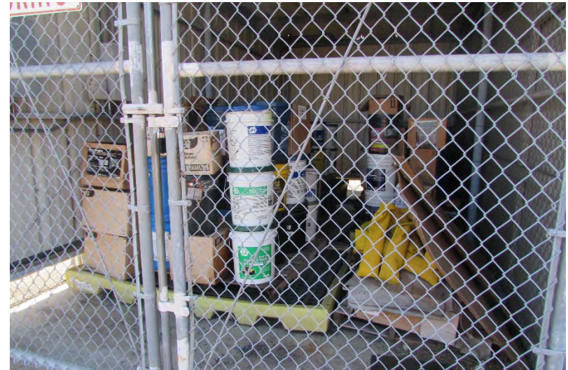
AIR-EE Photo 2.1.56 Covered Material Storage on Secondary Containment
