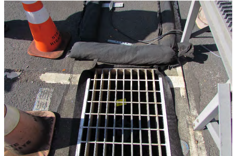
HWY-O Photo 6.1.116 Storm Drain Inlet With BMP
