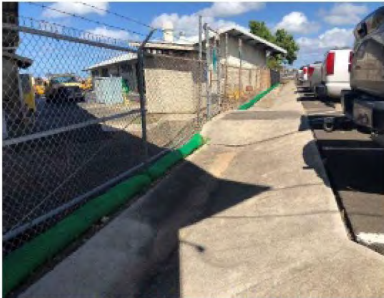
Figure 3. Another view of the debris cleaned out and filter sock placed along the concrete channel.
