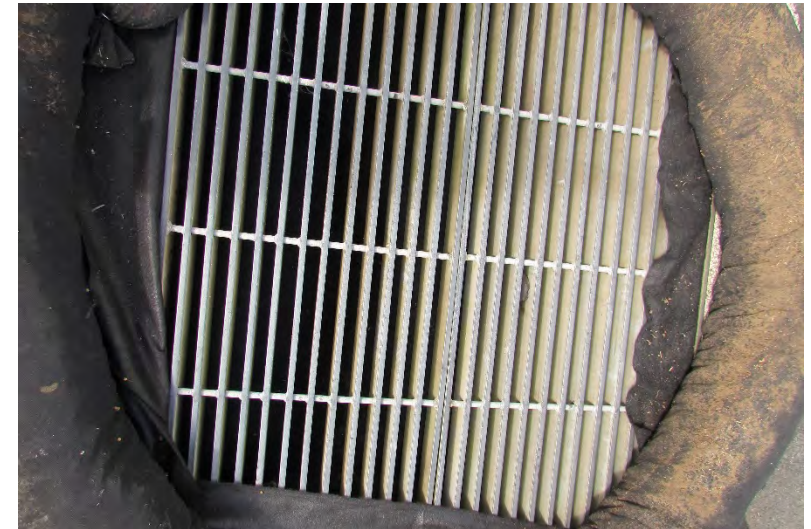
HWY-O Photo 6.2.70 Drain Inlet with BMP (Outside Vehicle Shed)
