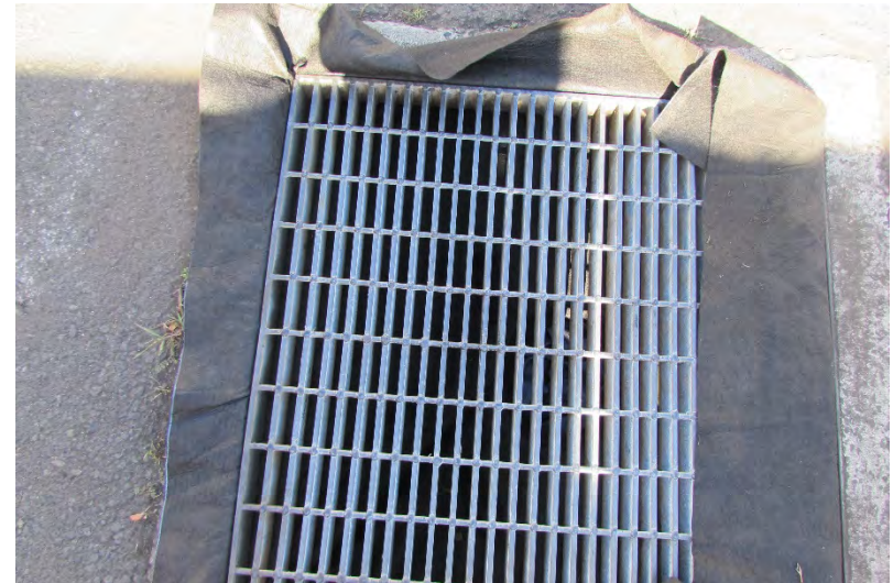
HWY-O Photo 6.1.28 Storm Drain Inlet with BMP
