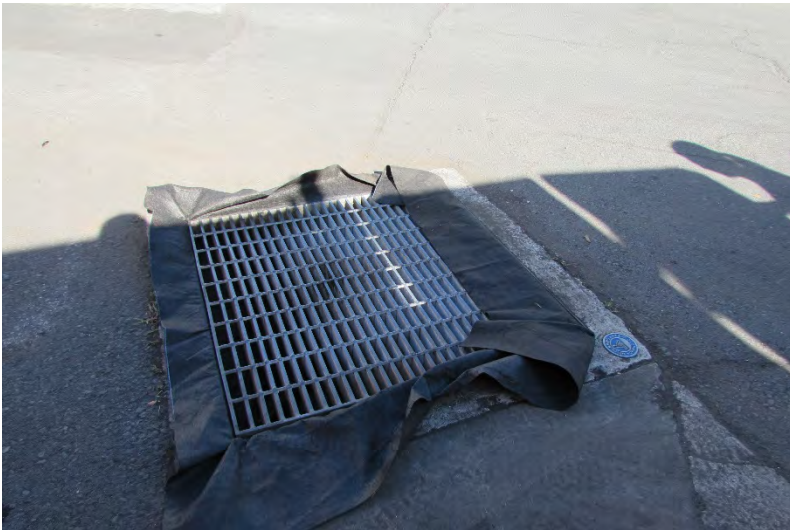
HWY-O Photo 6.1.27 Storm Drain Inlet with BMP
