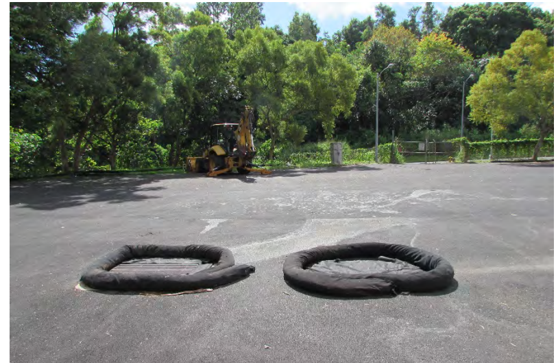
HWY-O Photo 6.2.32 Drain Inlets with BMPs
