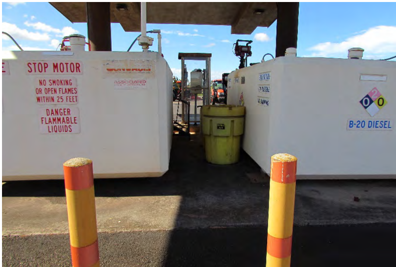
HWY-M Photo 5.2.136 Fueling Area ASTs and Spill Kit
