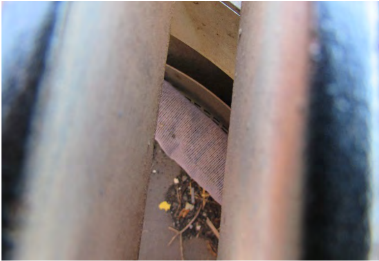
AIR-EE Photo 2.1.69 Storm Drain 5500 (With Safe Drain)
