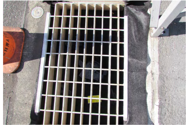
HWY-O Photo 6.1.114 Storm Drain Inlet With BMP
