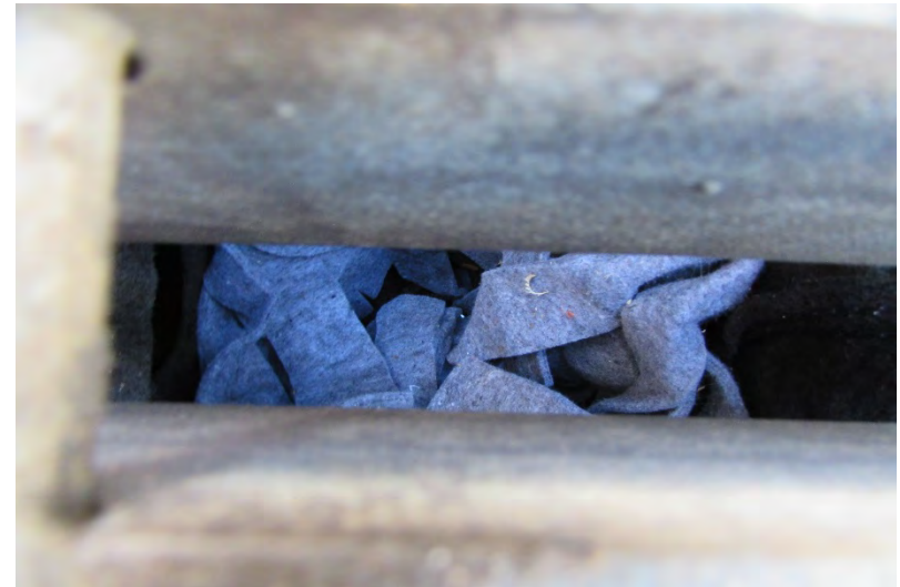
HWY-O Photo 6.1.36 Storm Drain Inlet with BMP
