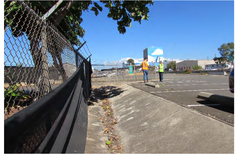
AIR-EE Photo 2.1.22 Concrete Channel near Employee Parking Area
