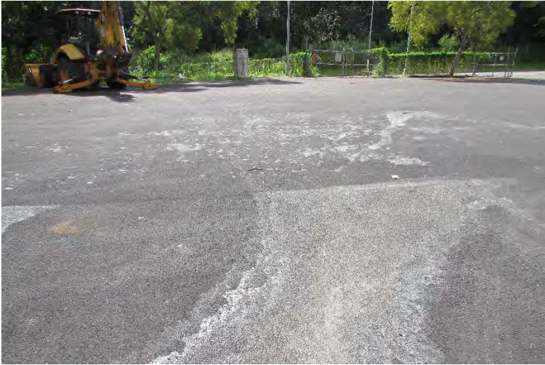
HWY-O Photo 6.2.37 White Residue on AC Pavement
