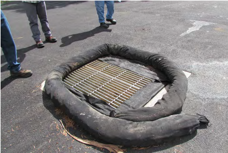
HWY-O Photo 6.2.33 Drain Inlets with BMPs
