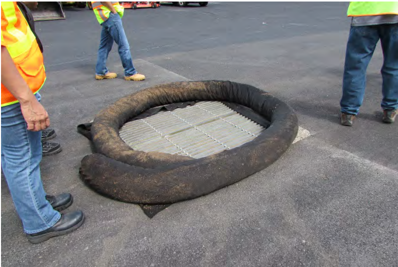
HWY-O Photo 6.2.69 Drain Inlet with BMP (Outside Vehicle Shed)
