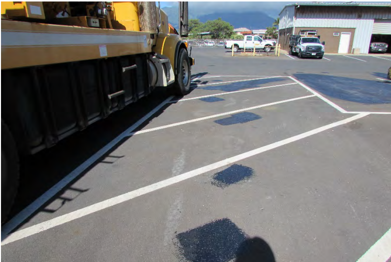
HWY-M Photo 5.2.142 Equipment Parking Area Asphalt Seal
