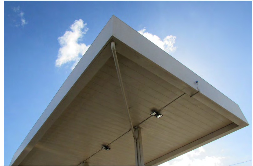
HWY-O Photo 6.1.106 Fuel Station Roof Drainage
