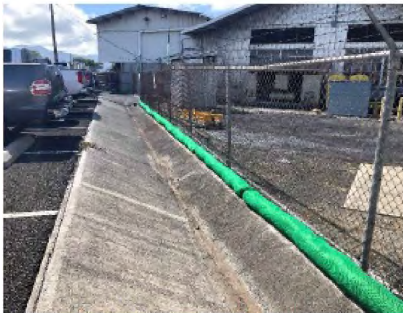
Figure 4. Another view of the debris cleaned out and filter sock placed along the concrete channel.
