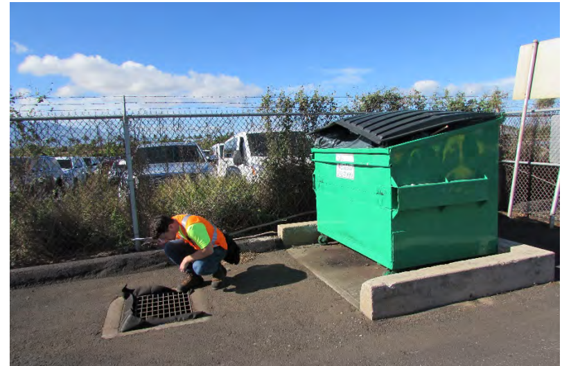
HWY-M Photo 5.2.28 Grated Drain Inlet/Dry Well
