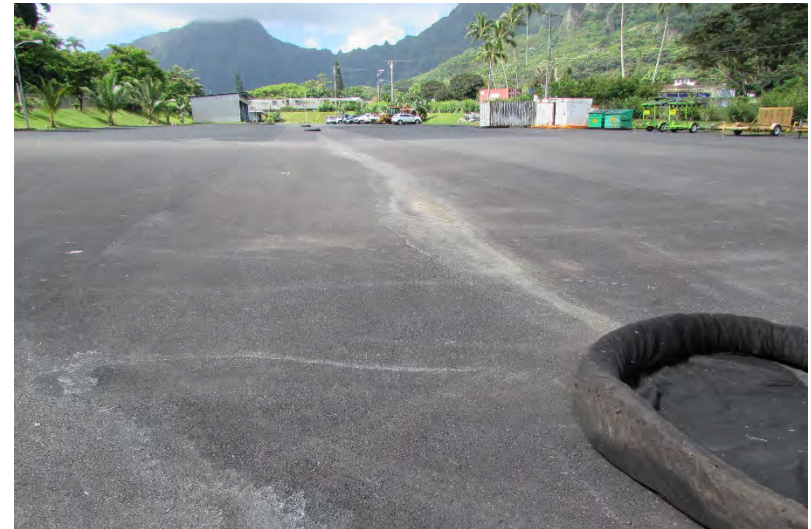
HWY-O Photo 6.2.36 White Residue on AC Pavement
