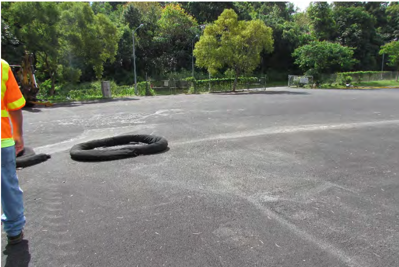
HWY-O Photo 6.2.31 Drain Inlets with BMPs
