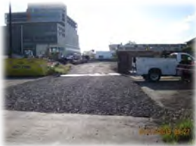
Stabilized construction entrance.
