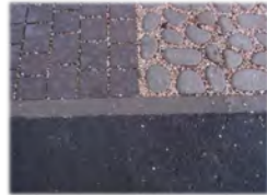
Install Permeable Pavers
