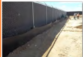
Properly installed silt fence
