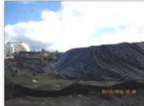
Properly contained stockpile.
