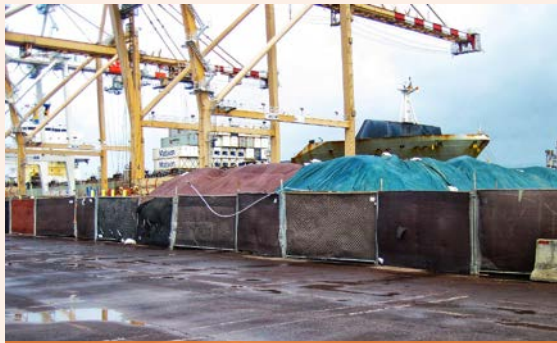
Properly covered and contained stockpile.
