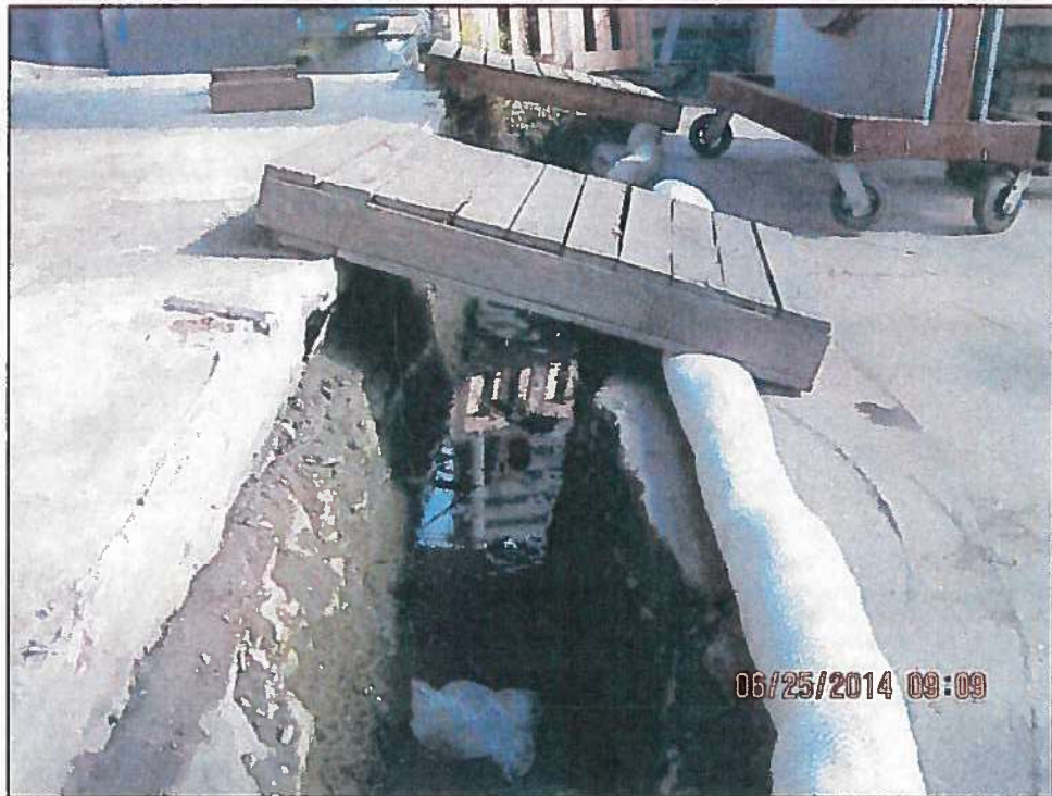
Photo 5: Litter scattered in the trench drain, bermed with biosocks (facing north-northwest).
