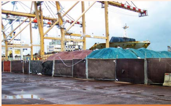
Properly covered and contained stockpile.
