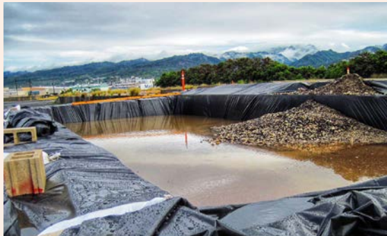
Concrete washout containment.
