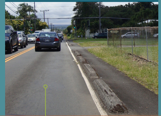
Example of extruded curbing. See page 4-36 for cautions related to extruded curbs.
