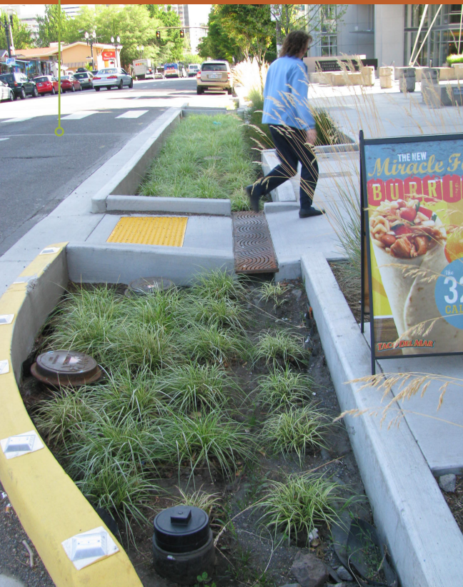
Stormwater infiltration system on a green street in Portland, OR. ( www.pedbikemages.org/LauraSandt )
