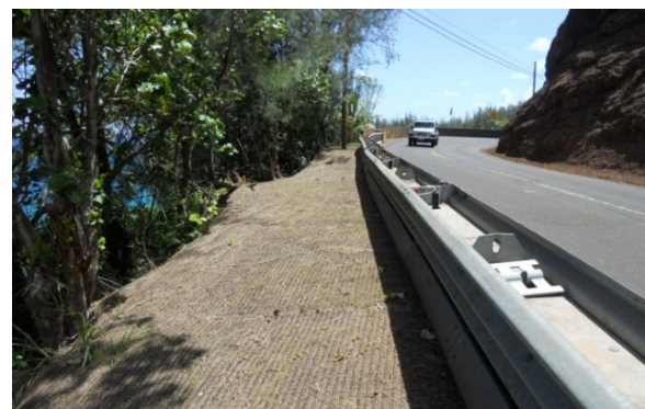
Landslide protection, Kuhio Highway, Lumahai, Kauai.
