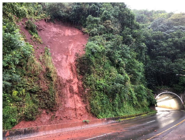
Bulk of the debris is removed at the landslide location at the Kailua bound direction. The slope along the Honolulu bound direction needs to be stabilized before it can be reopened.
