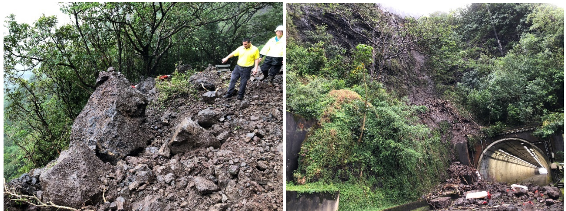
Damage to Pali Highway as a result of multiple landslides on February 18, 2019. Reconstruction of the roadway with the soil nails occurred from April 2018 to April 2019. Large boulders at risk of falling down to the Pali Highway. Two separate landslides affected both Kailua-bound and Honolulu-bound traffic.
