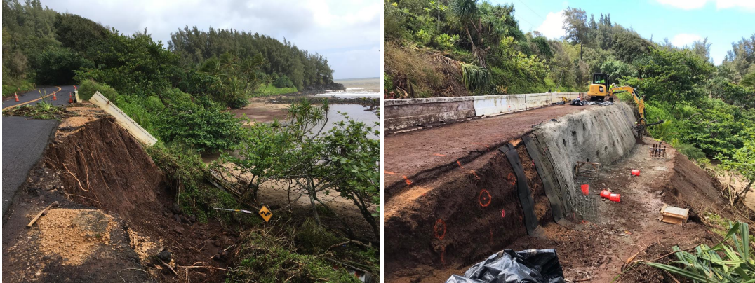
Damage to Kuhio Highway as a result of heavy rains in April 2018. Reconstruction of the roadway with the soil nails occurred from April 2018 to April 2019.
