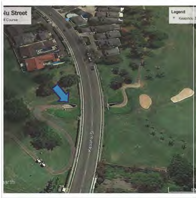
Kealahou Street Underpass (typical golf course installation)
