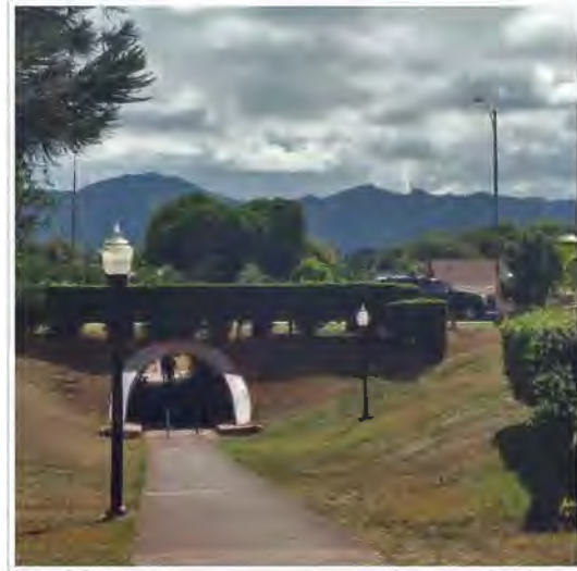
Kamehameha Highway Underpass (pedestrian can be seen at end of underpass)
