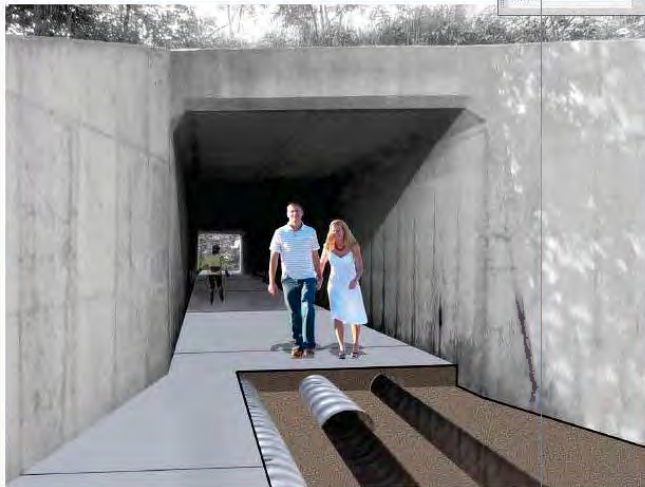
Highway 30 Underpass concept Mount Vernon, Iowa DOT: Note drainage culverts beneath walkway and general dimensions of 10.4' x 10'
