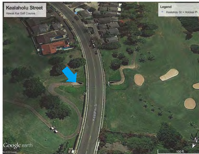
Kealahou Street Underpass (Typical golf course application) Hawaii Kai
