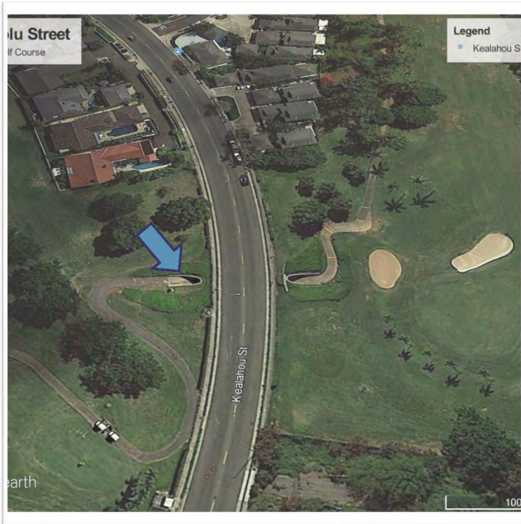
Kealahou Street Underpass (typical golf course installation)
