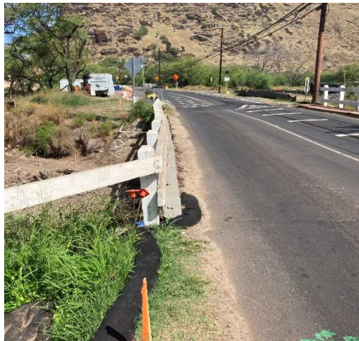
Figure 5.3. Makaha Bridge No. 3
