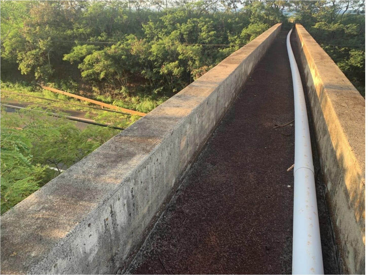
Image 3. Solid parapet and flume channel. Facing southwest.
