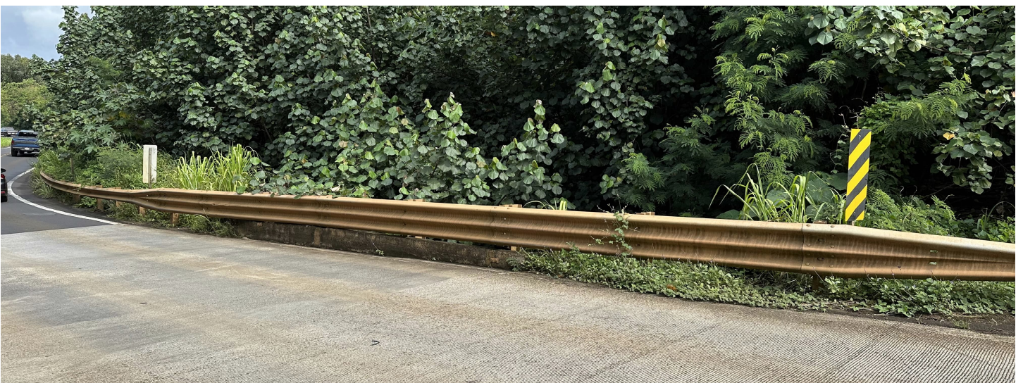
Image 3. View of raised deck and three beam railings, facing northwest.
