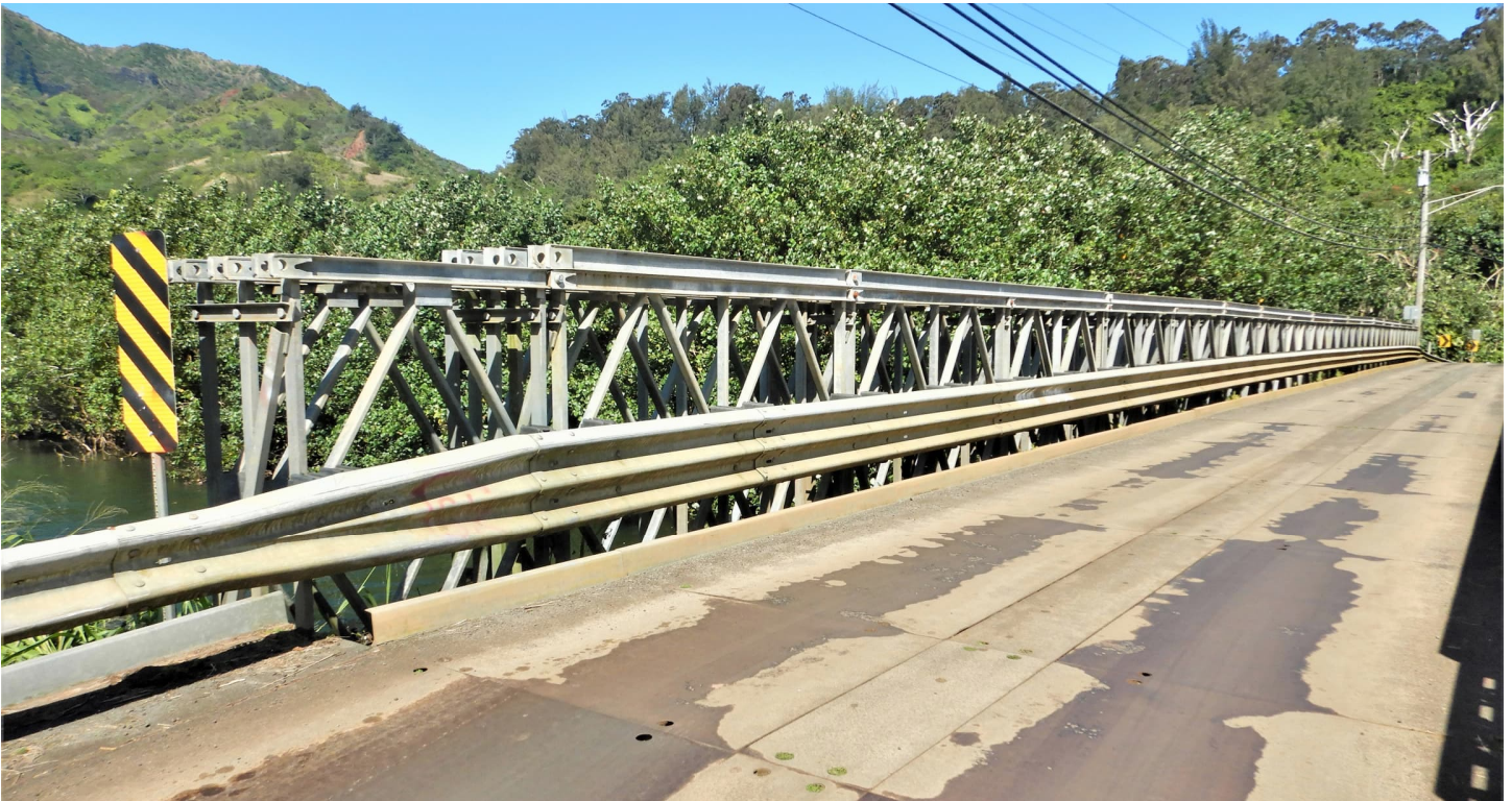
Image 4. Bridge deck and ACROW structure, facing southwest.
