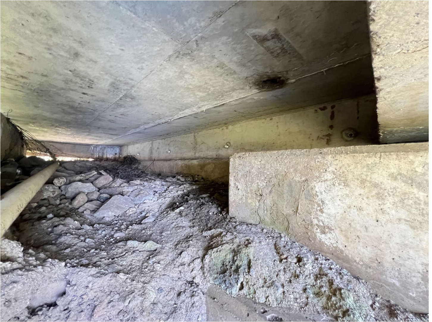
Figure 3. Waipa Stream Bridge, detail of abutment.
