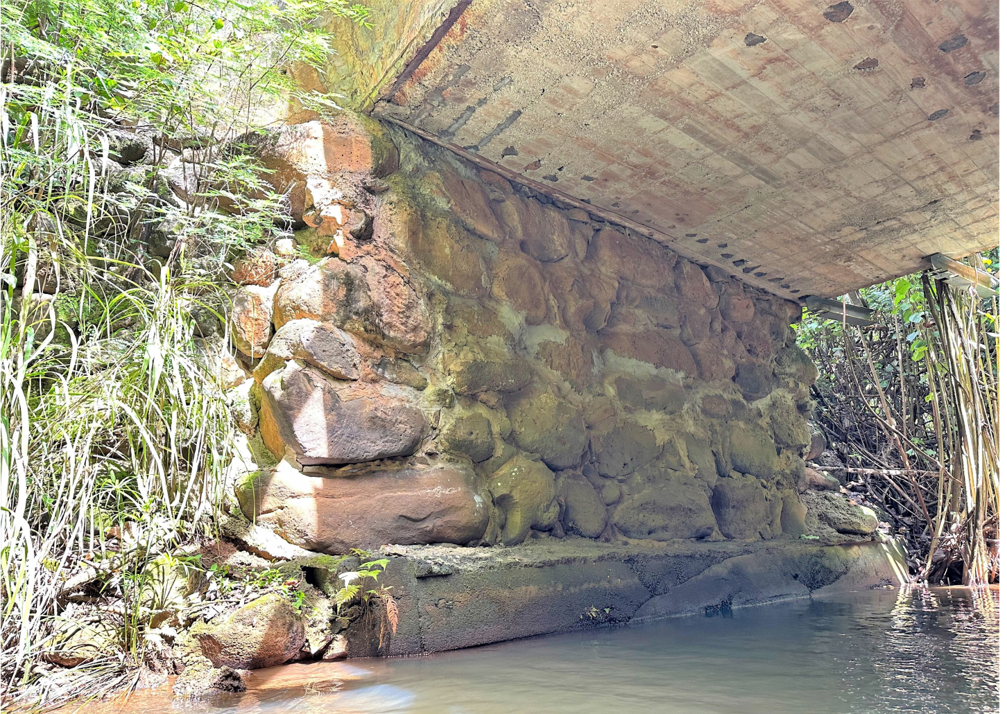
Image 2. Detail of patched CRM abutment.
