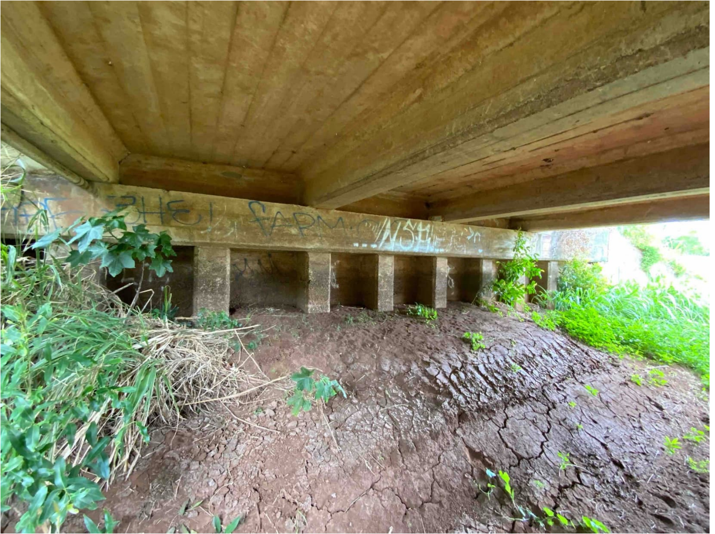
Figure 2. Kuilima-Oio Stream Bridge view of abutment and bridge deck.
