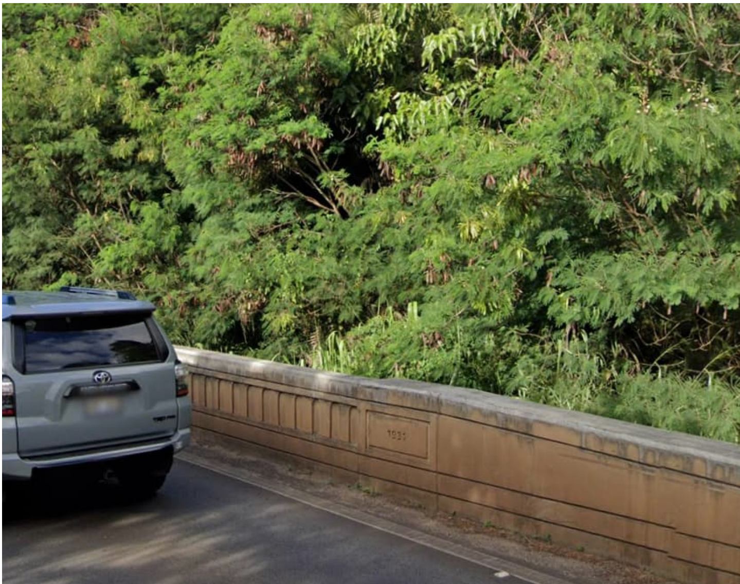
Image 4. Southeast replacement parapet end post with 1931 construction date, facing east. Source: Google Maps, July 2019.
