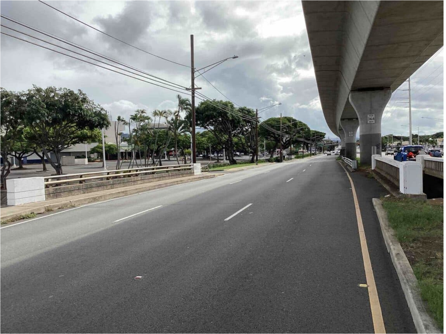
Image 2. Roadway facing east. Note the original parapet (right) and altered parapet (left) from road widening.
