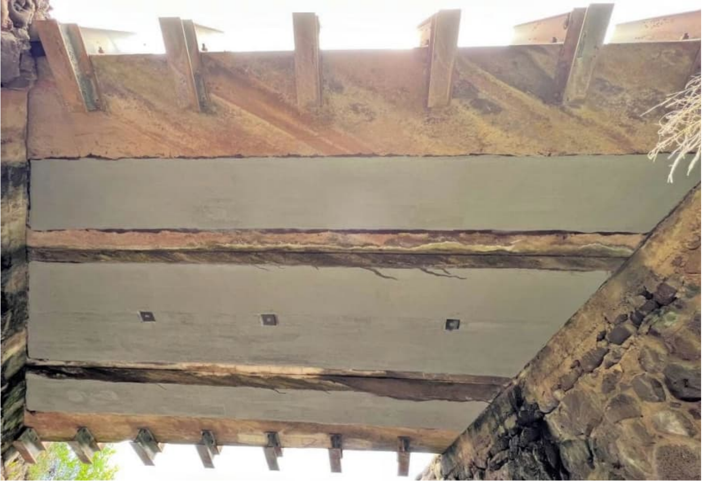
Image 3. View of bridge deck underside and CRM abutment.
