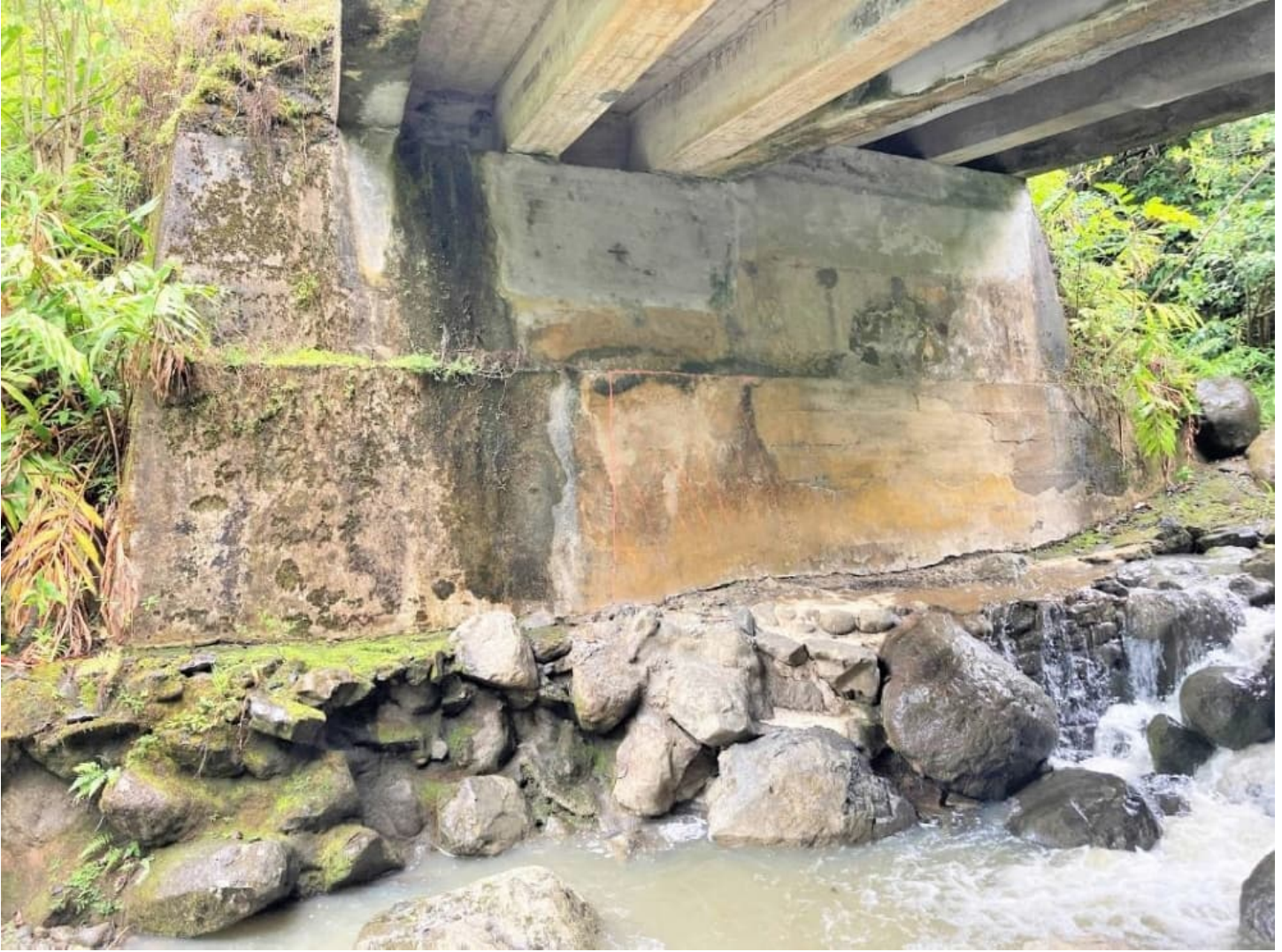
Image 6. View of southeast abutment and deck girders, facing south. Note the different girder depths indicating construction in 1911 (mauka) and 1940 (makai).
