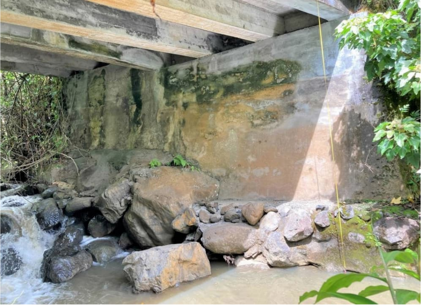
Image 5. View of northwest abutment and deck girders, facing north. Note the different girder depths indicating construction in 1911 (mauka) and 1940 (makai).
