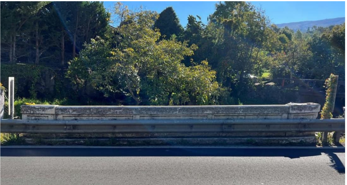
Image 2. View of west parapet with thrie beam.
