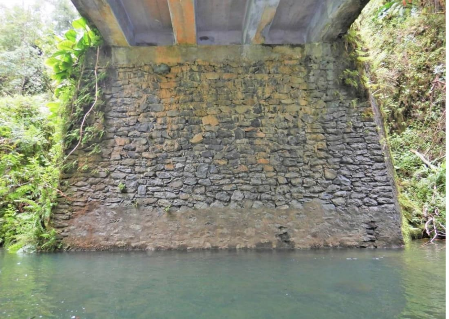
Image 5. View of southeast CRM abutment and deck girders, facing southwest.
