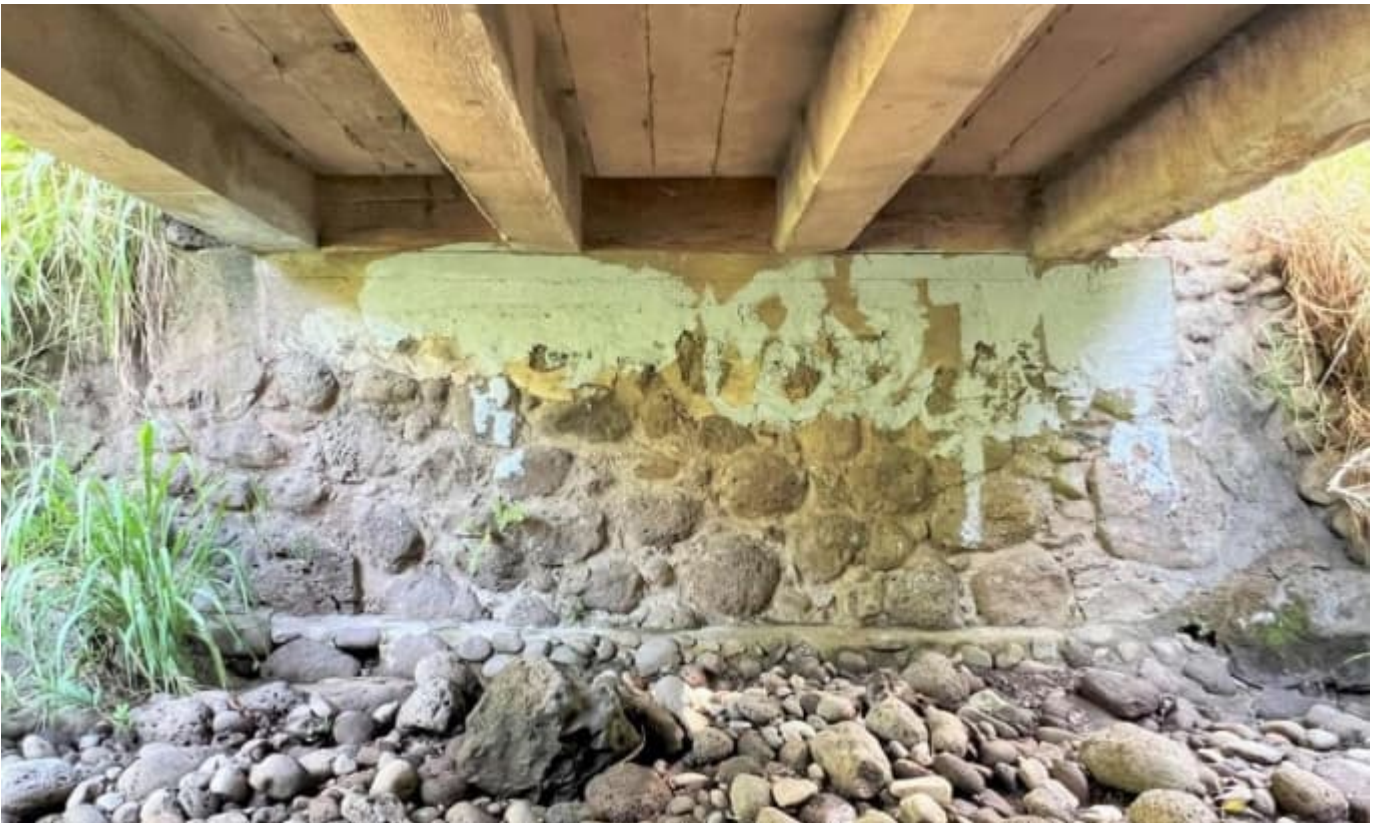
Image 2. Detail of CRM abutment and deck girders.
