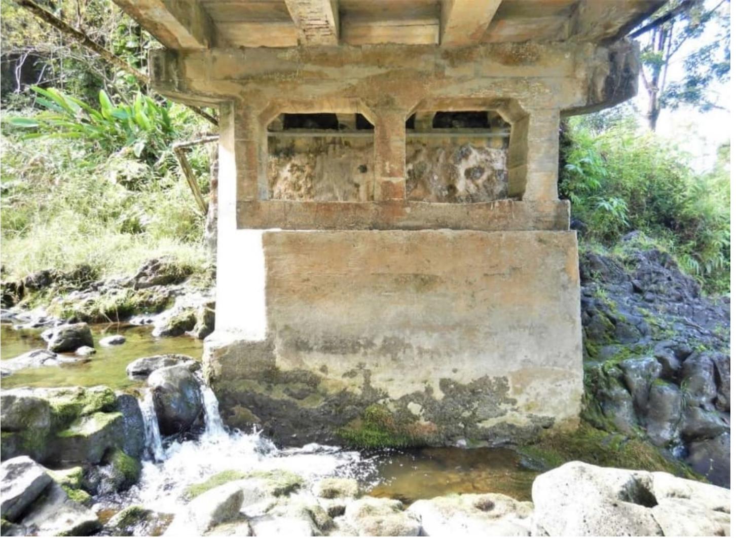
Image 5. Pier and deck girders, facing west.
