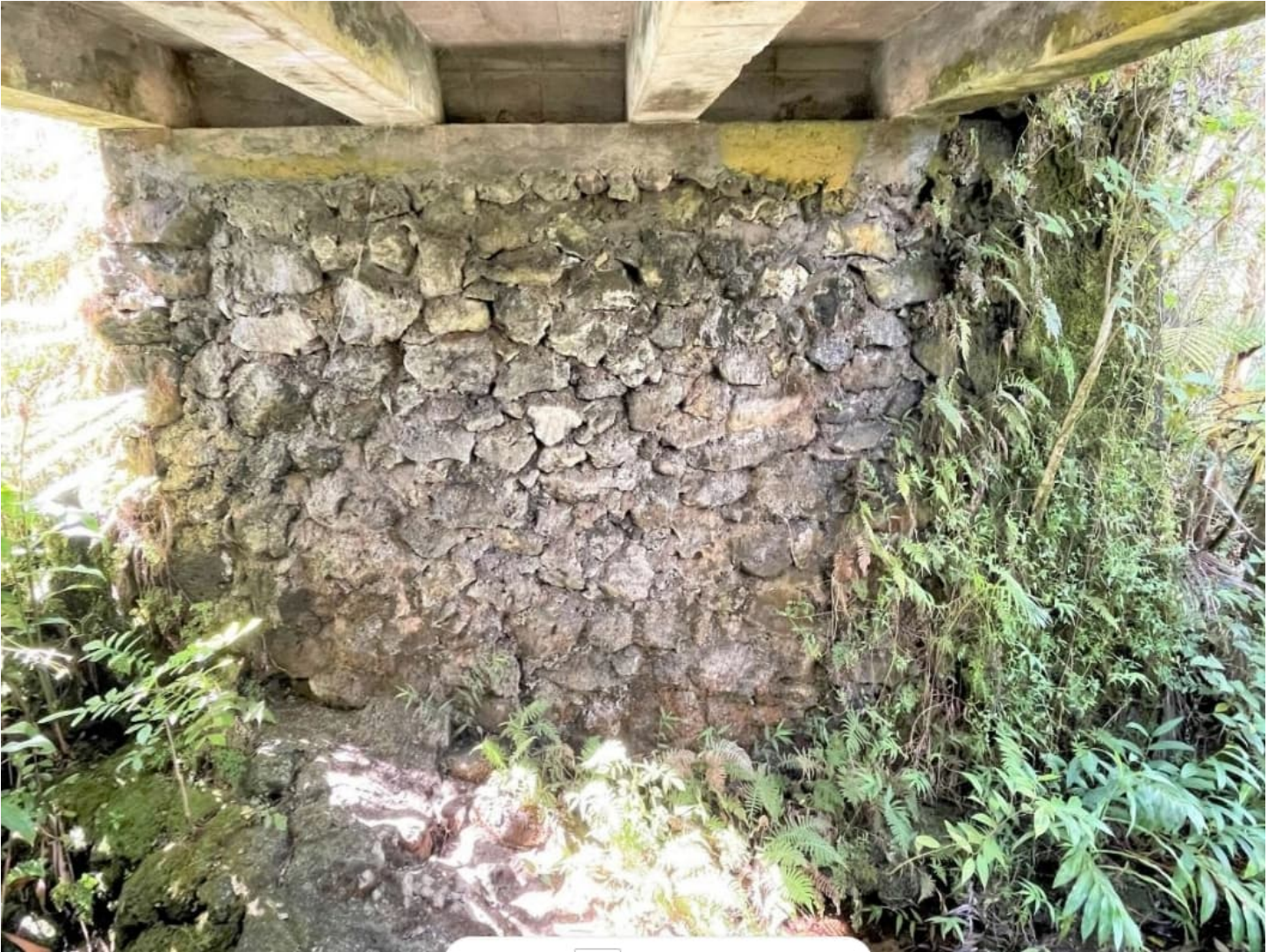
Image 3. West CRM abutment and deck girders, facing west.
