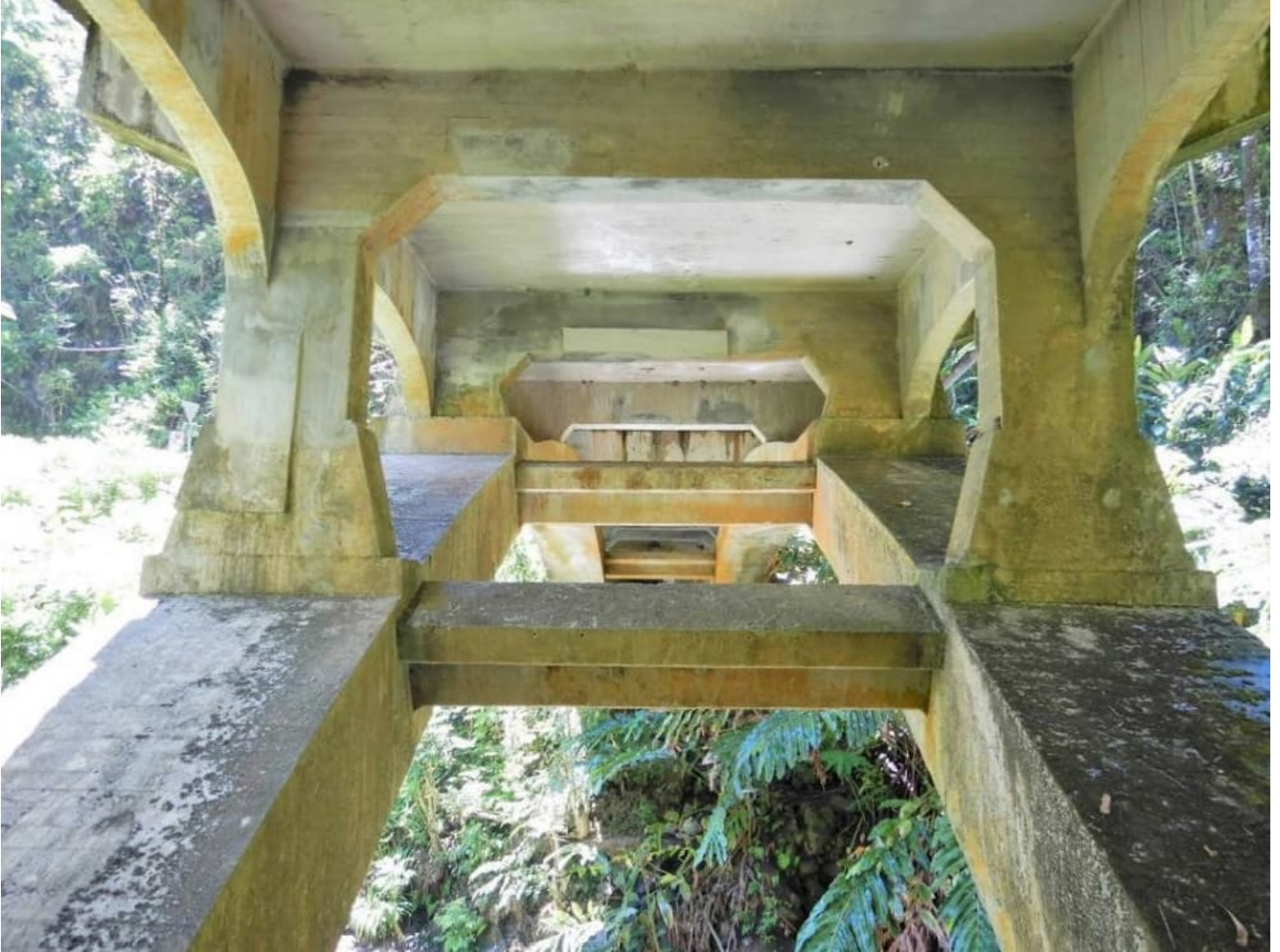
Image 4. View of open spandrel arch and support girders, facing southeast.
