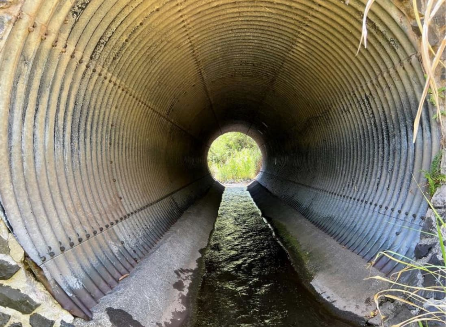
Image 3. Detail of culvert cell.
