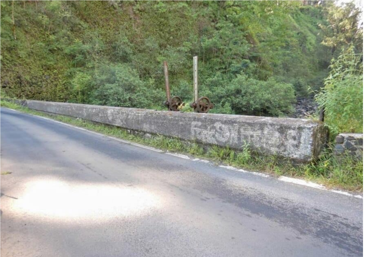
Image 3. View of south parapet/truss, facing southeast. Note East Maui Irrigation system sluice pulleys in foreground.
