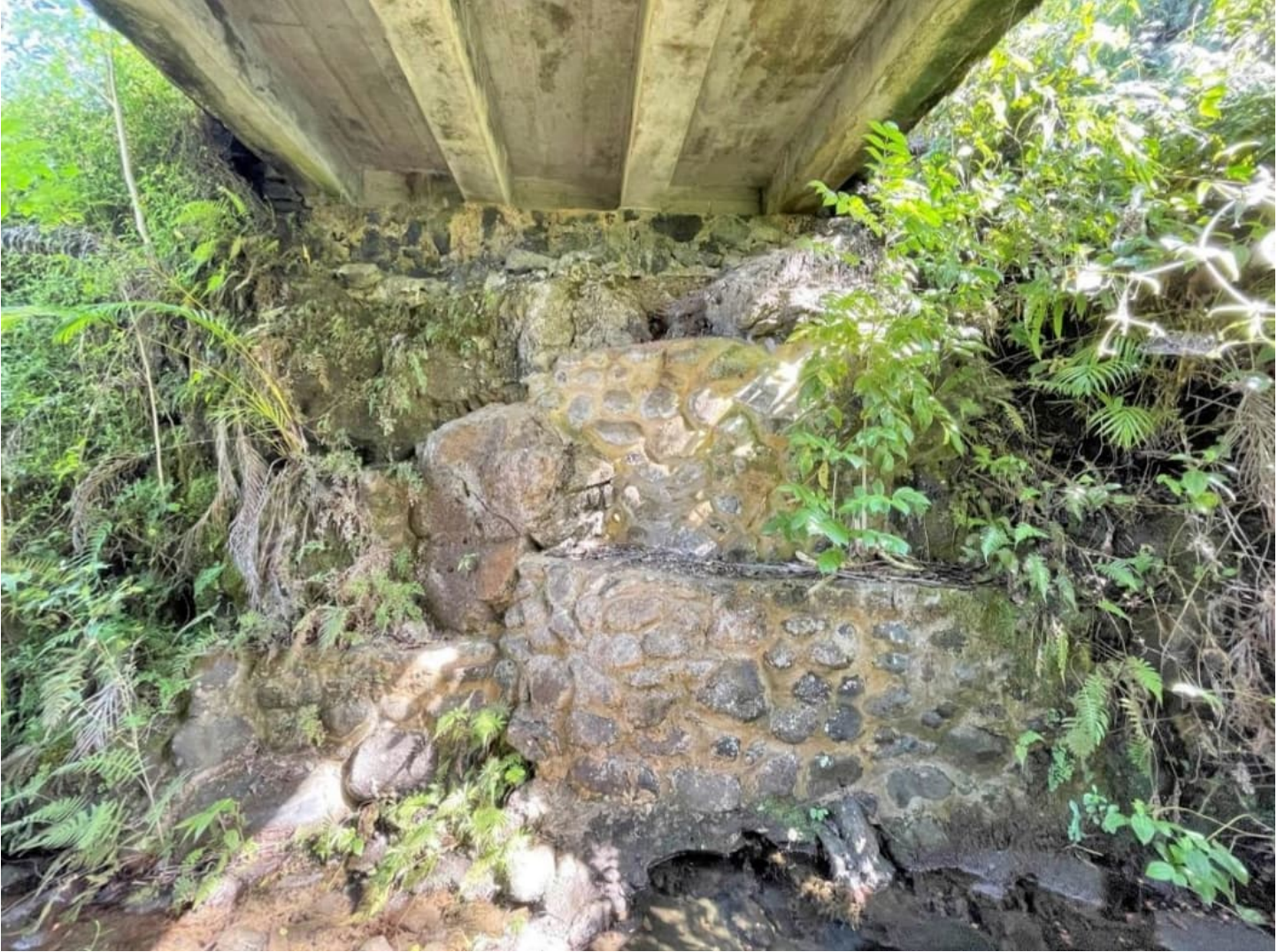
Image 4. East abutment and deck girders, facing east.
