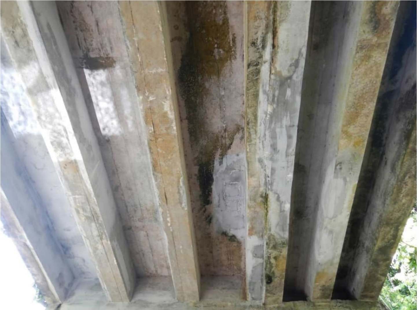
Image 6. Detail of deck girders, facing southeast. Note irregular girder width marking 1911 construction (right) and 1940 widening (left).
