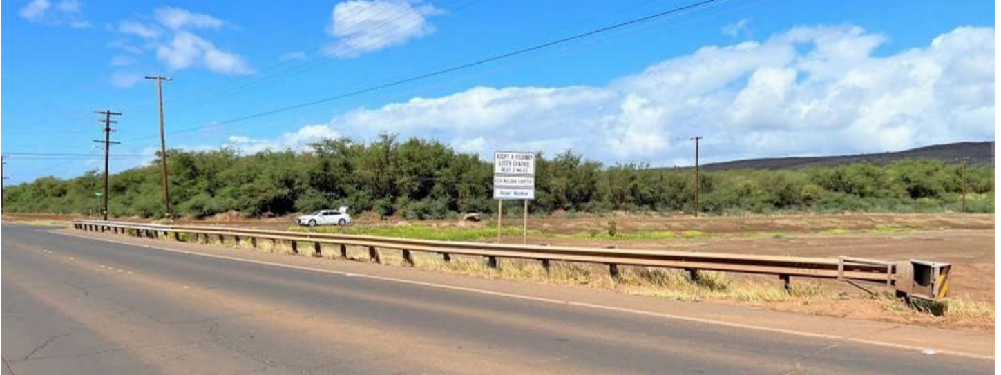
Image 3. View of northeast three beam railing and general setting of culvert.
