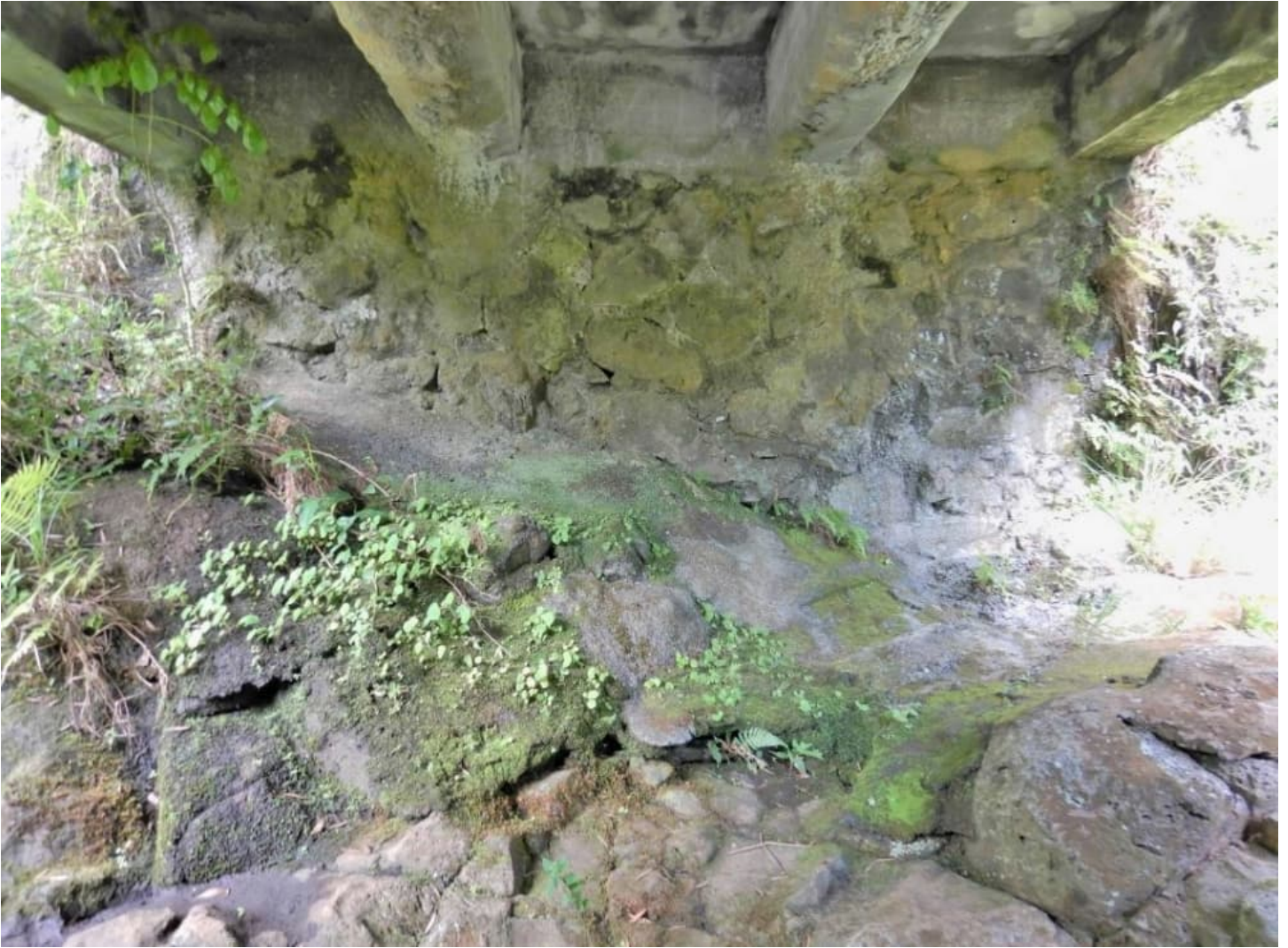
Image 5. View of northwest CRM abutment and deck girders, facing northwest.
