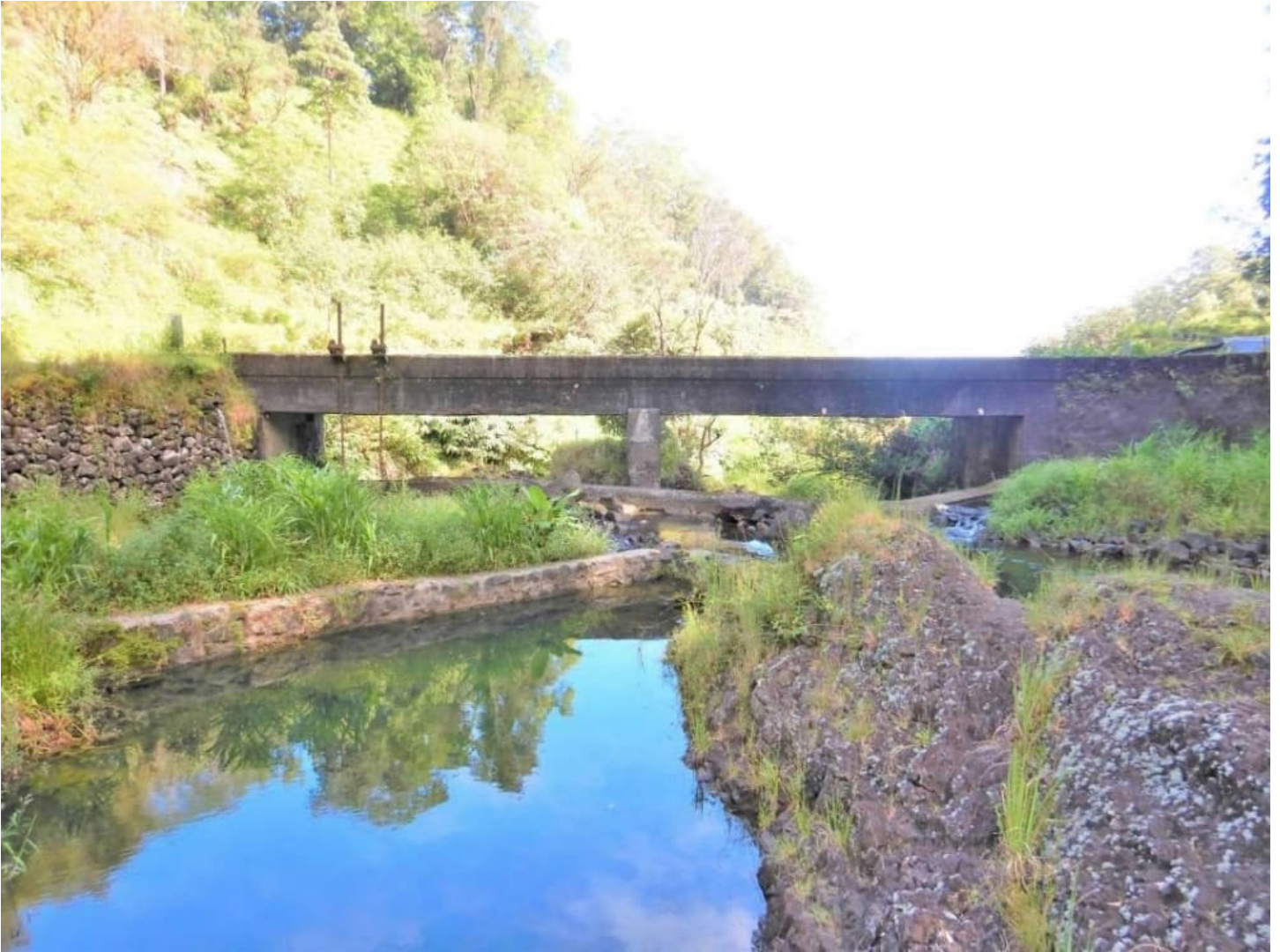
Image 1. General view of bridge, facing north. Note pulleys and sluice gate on the left for the East Maui Irrigation System.
