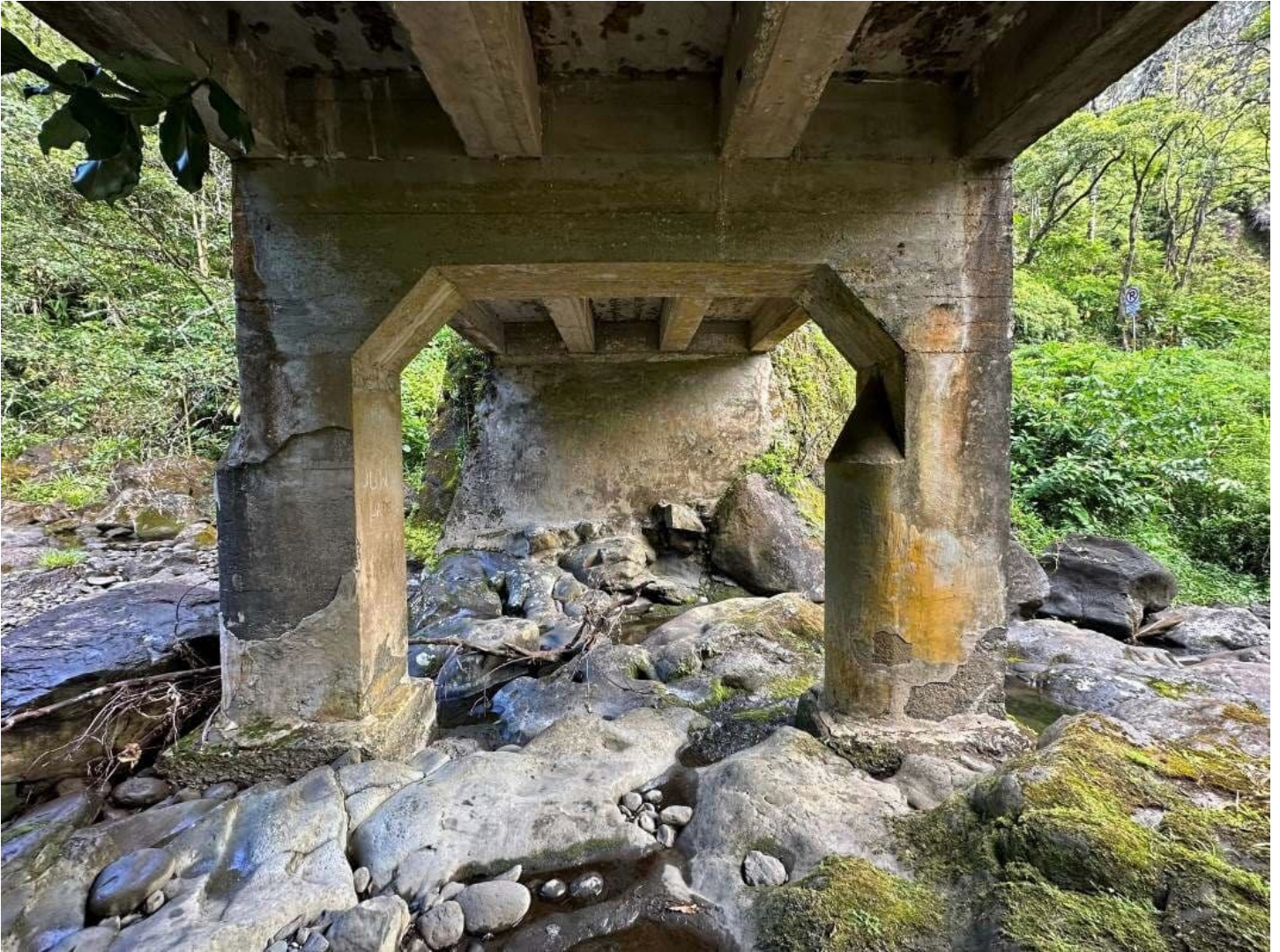
Image 6. View of pier, western abutment, and deck girders, facing west.
