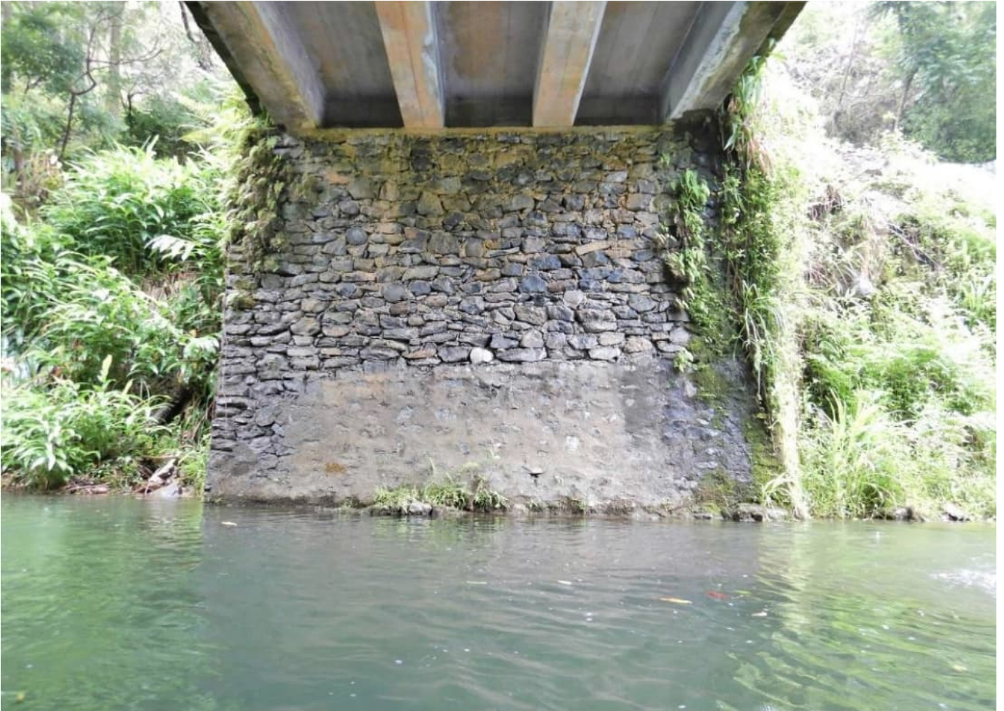
Image 4. View of northwest CRM abutment and deck girders, facing northwest.
