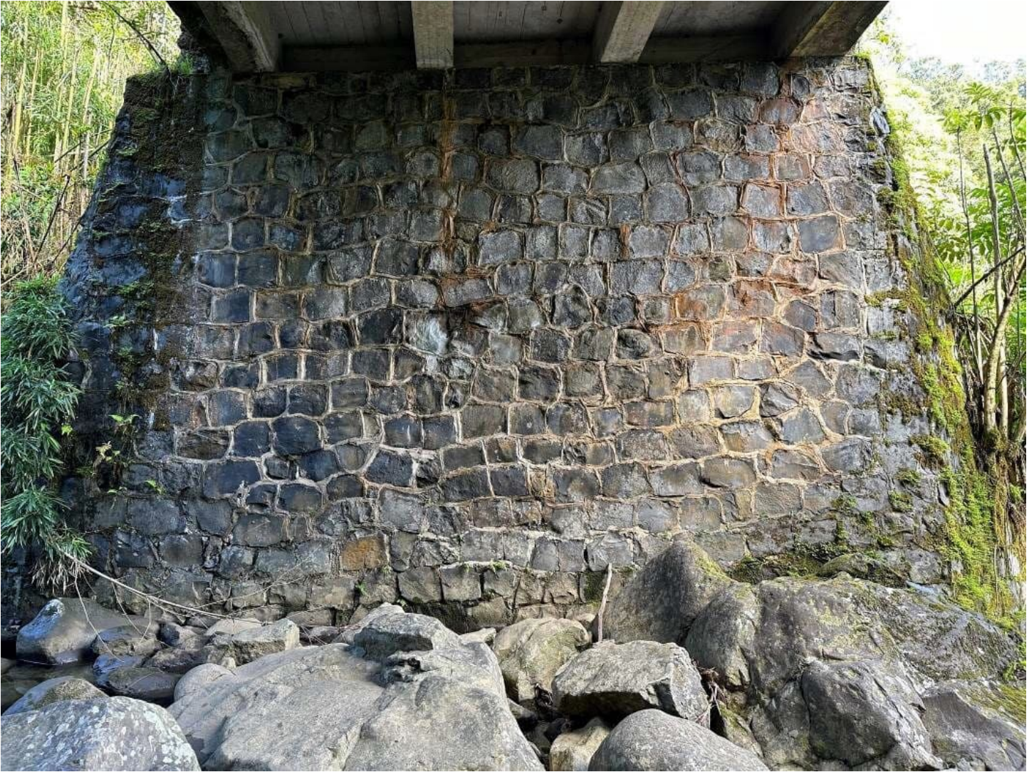
Image 7. View of CRM abutment, facing northwest.
