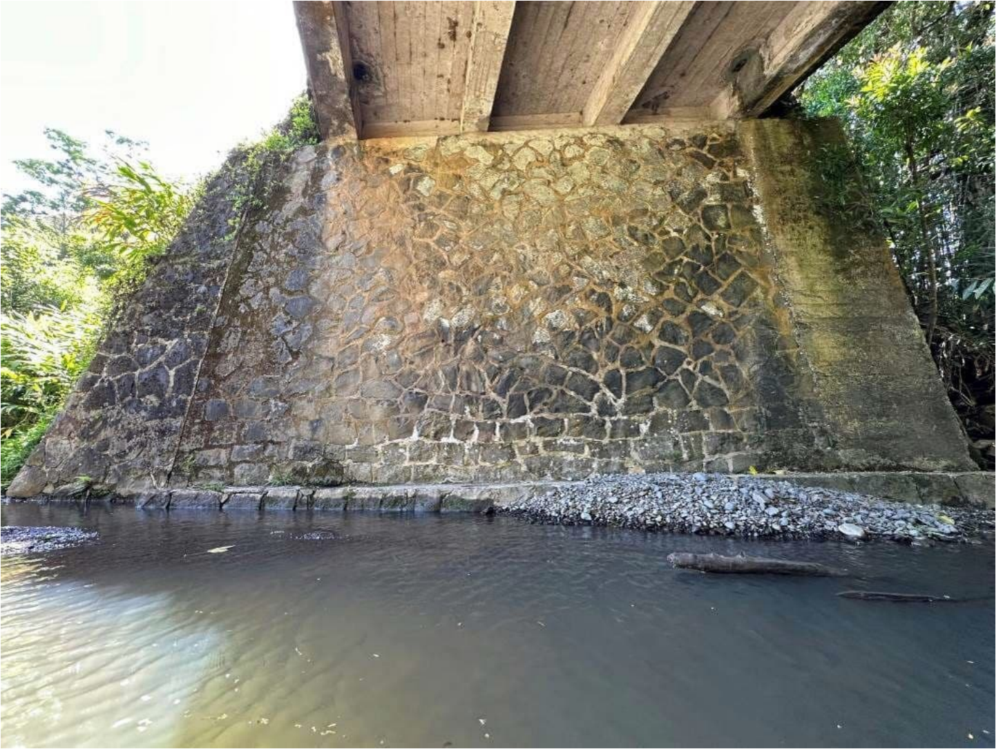
Image 9. View of southeast abutment and CRM wall.
