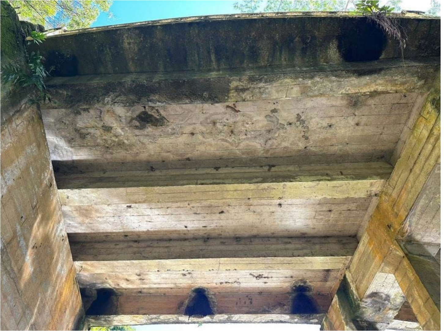
Image 6. Detail of northwest abutment, bridge girders, and pier.
