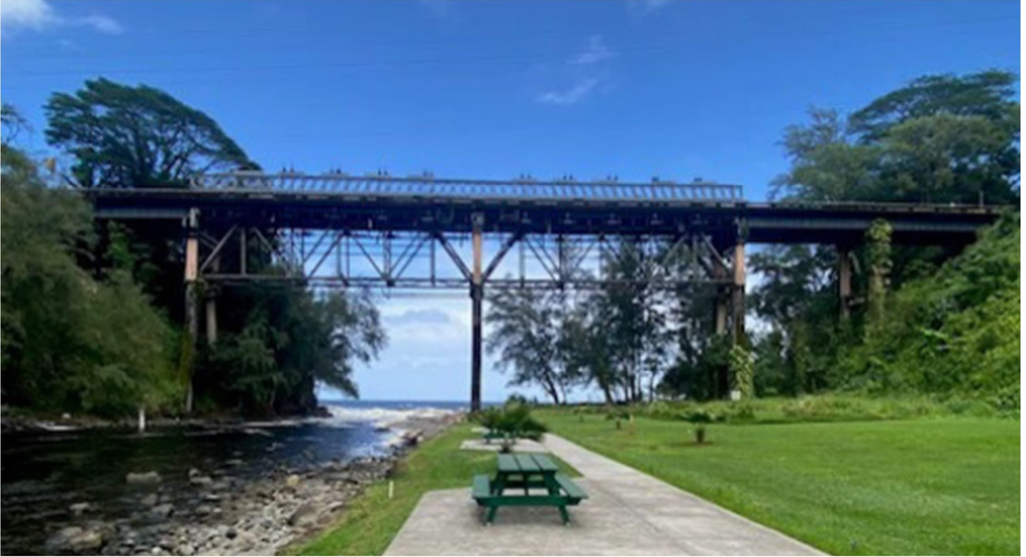
Image 1. General view of bridge, facing northeast. Temporary trusses visible while bridge undergoes repair work.
