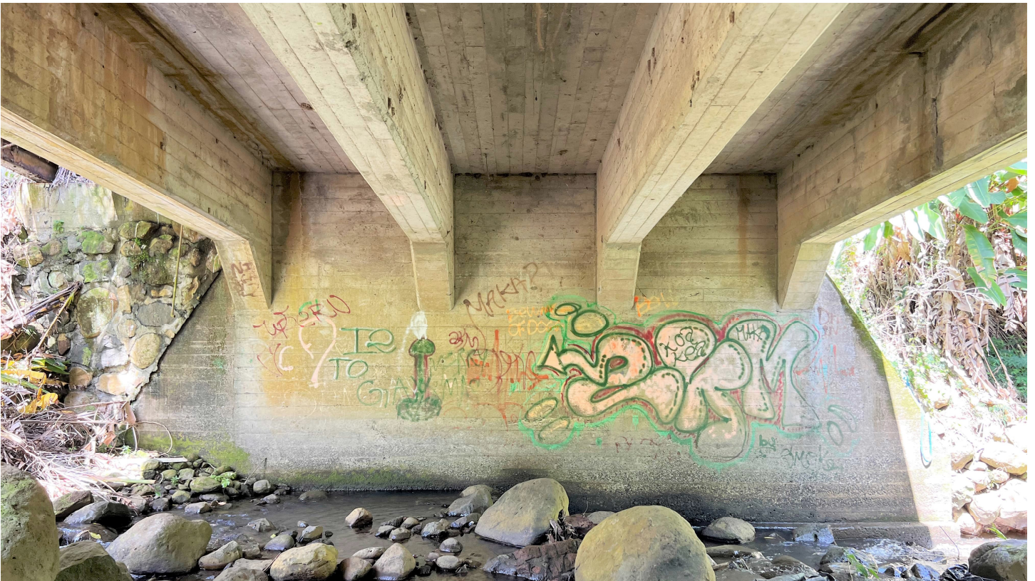
Image 2. West abutment and girder structure.
