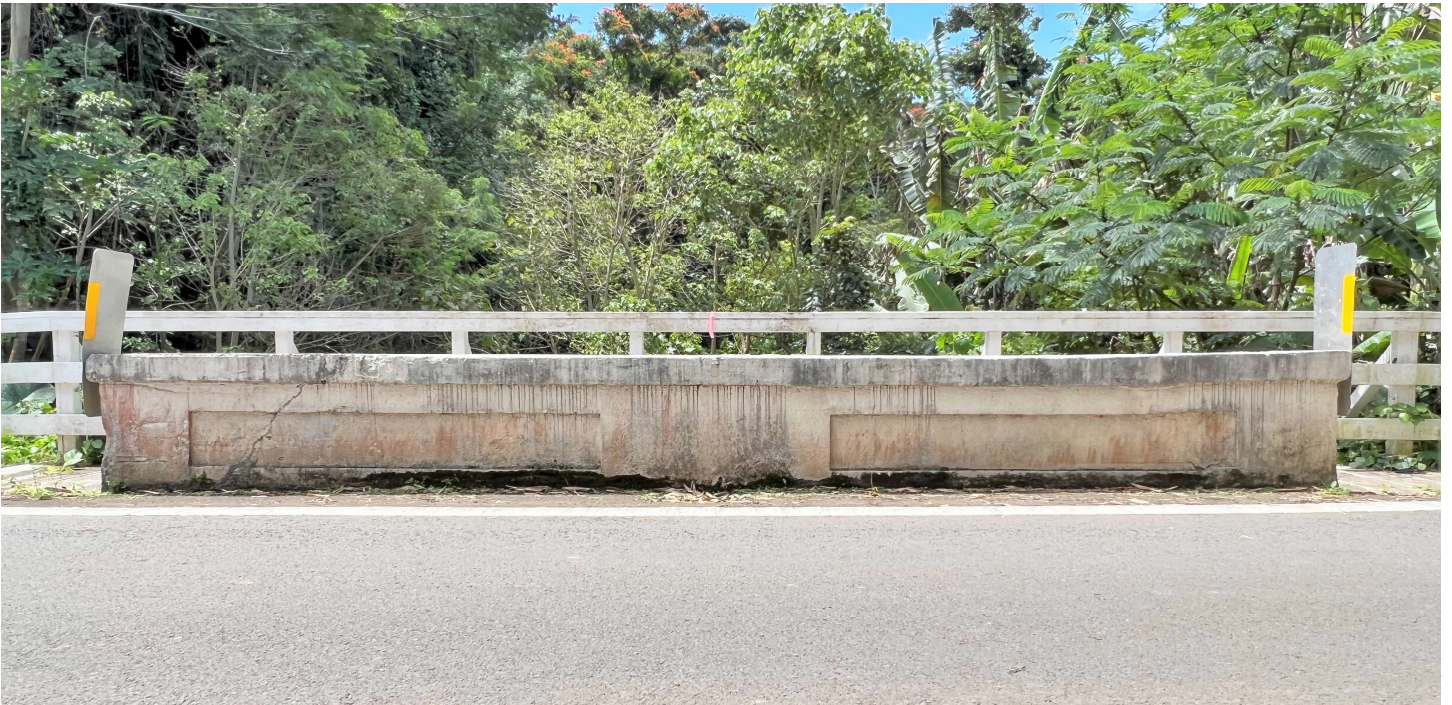
Image 4. Detail of concrete solid parapet and wooden walkway railing, facing north.
