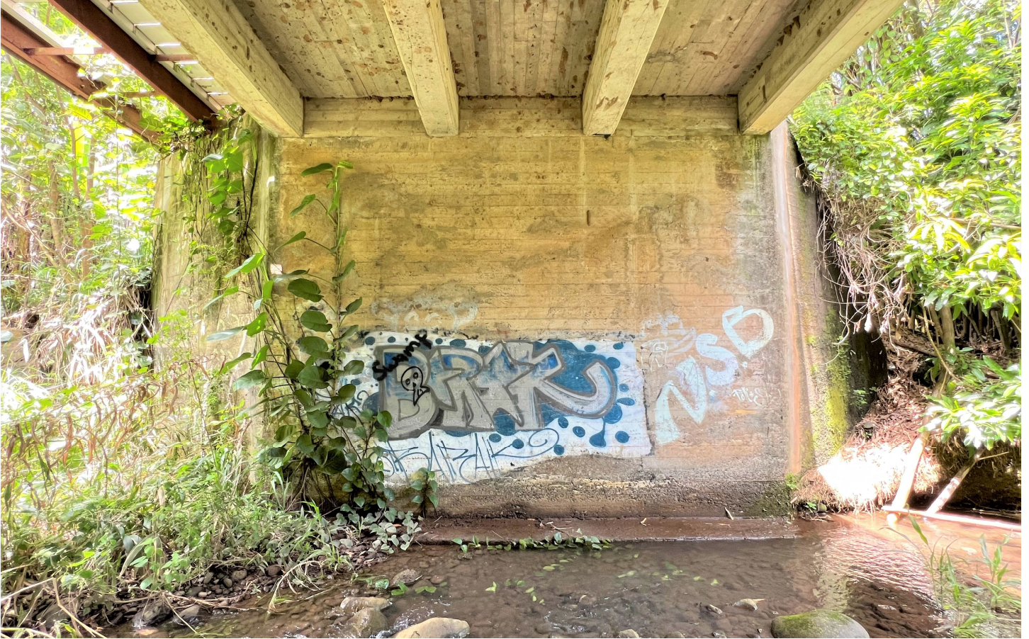
Image 3. Detail of west abutment and deck girders.
