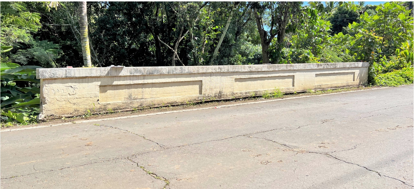
Image 4. Concrete solid parapet, facing northeast.
