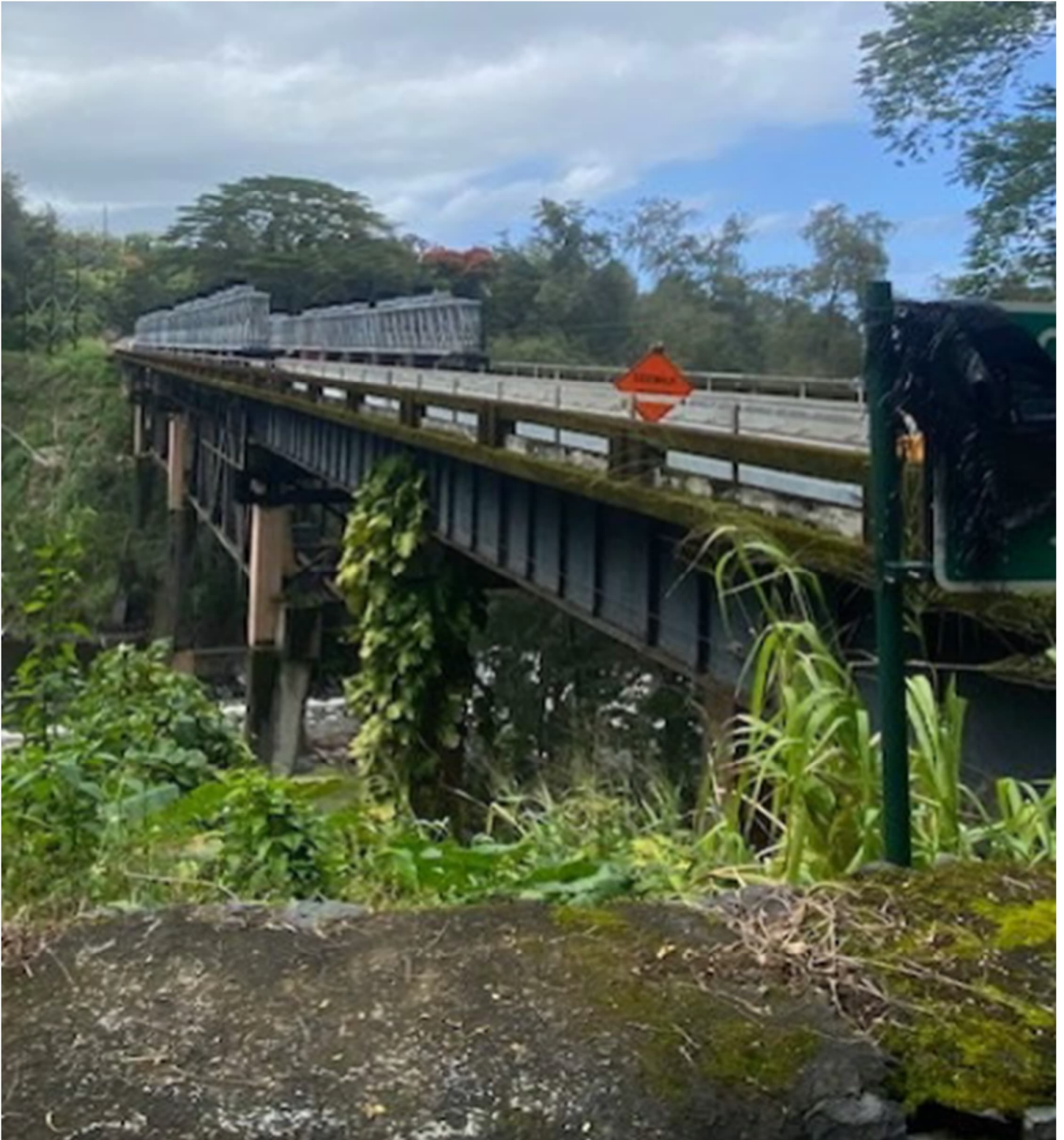
Image 3. View of bridge deck, railings, and piers, facing northwest. Temporary trusses visible while bridge undergoes repair work.
