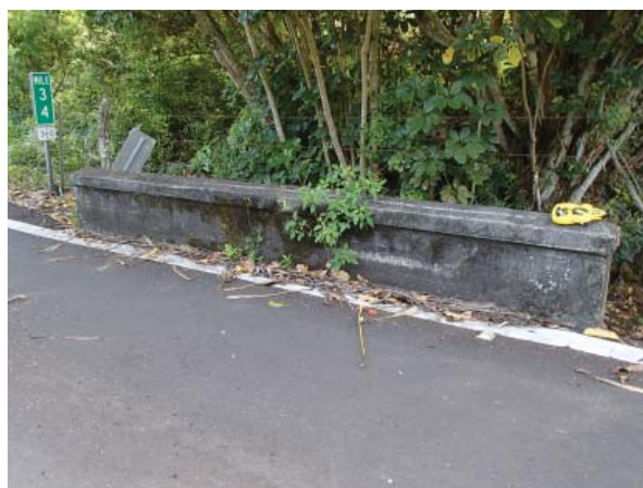
Solid parapet Courtesy of NOEI
