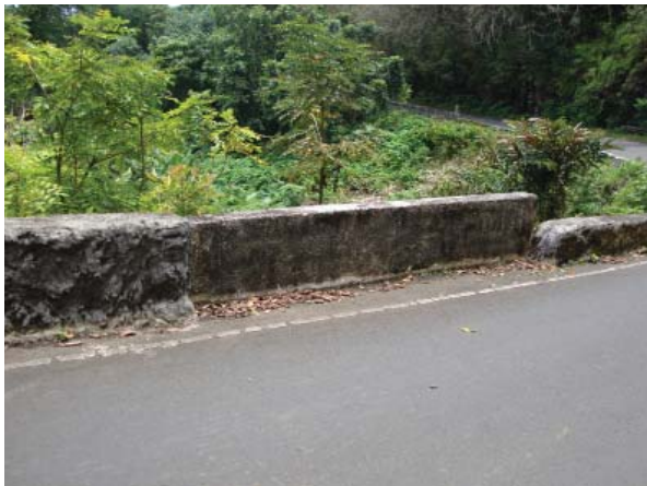
Solid concrete parapet, downstream side Courtesy of FAI
