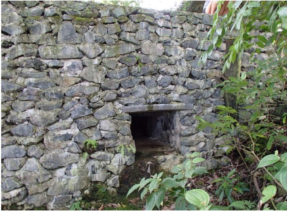
View of downstream CRM headwall / parapet.
