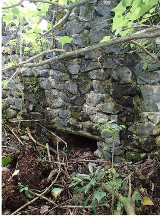
View of downstream CRM headwall / parapet.
