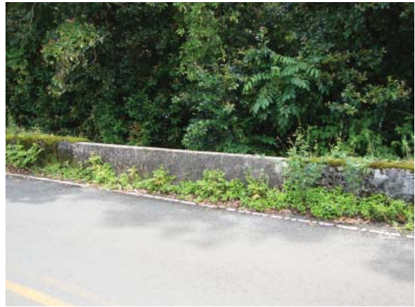
Solid concrete parapet, upstream side Courtesy of FAI
