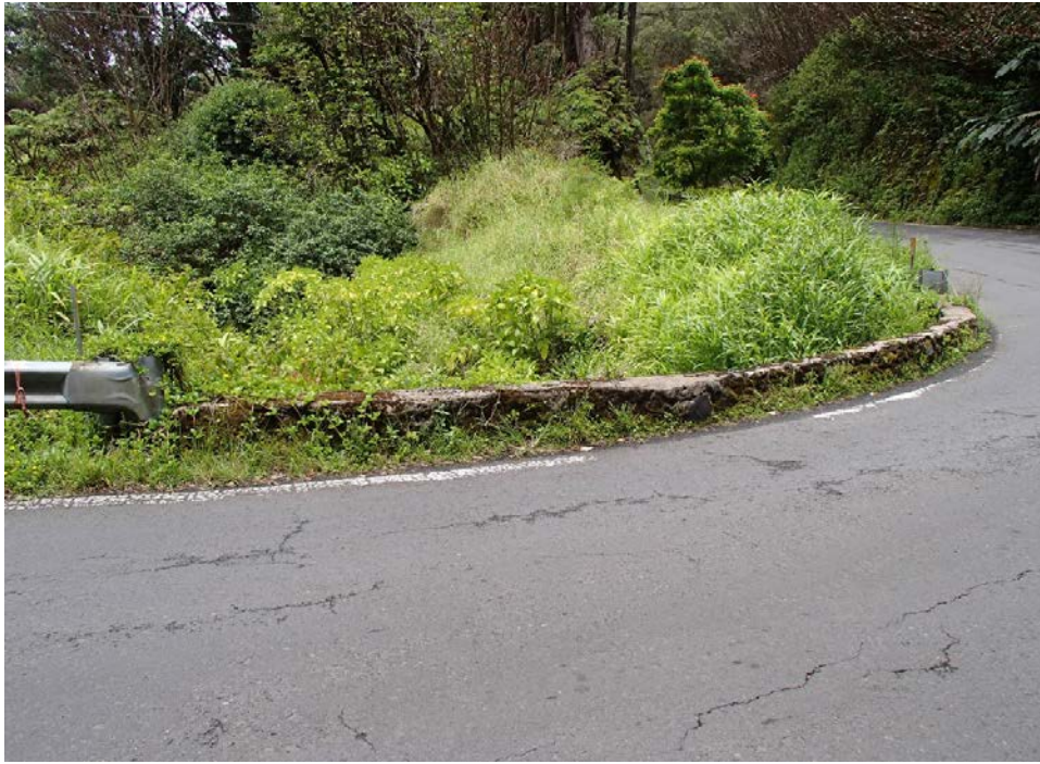
View of downstream CRM parapet.
