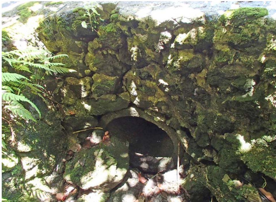
View of upstream CRM headwall / parapet and 24" diameter RCP inlet.
