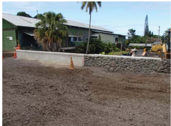
Solid concrete parapet, downstream side, and approach wall Courtesy of NOEI
