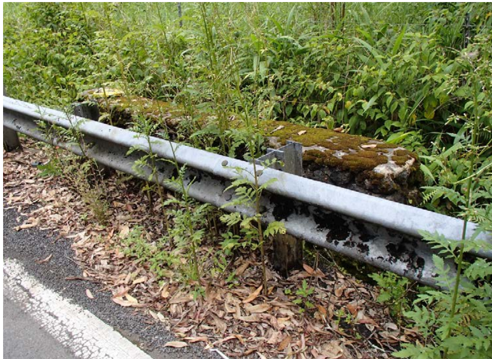
View of upstream CRM parapet with continuous metal guardrail in-front.
