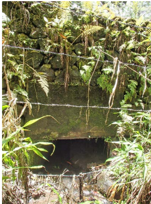
View of CRM parapet and concrete headwall at upstream side.
