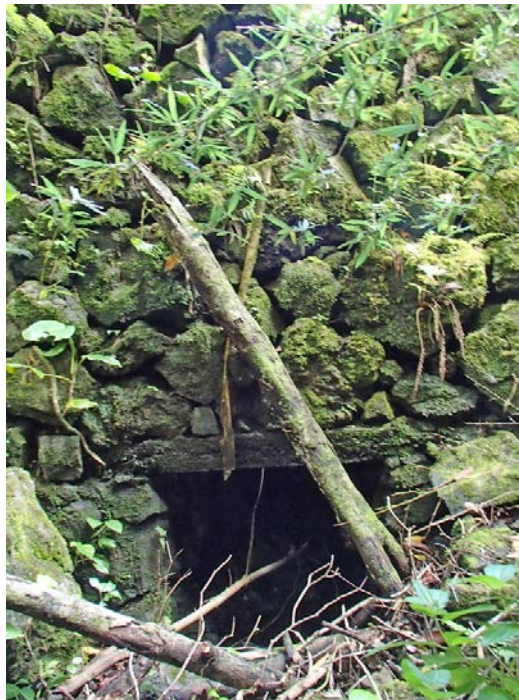
View of CRM headwall / parapet at upstream side.
