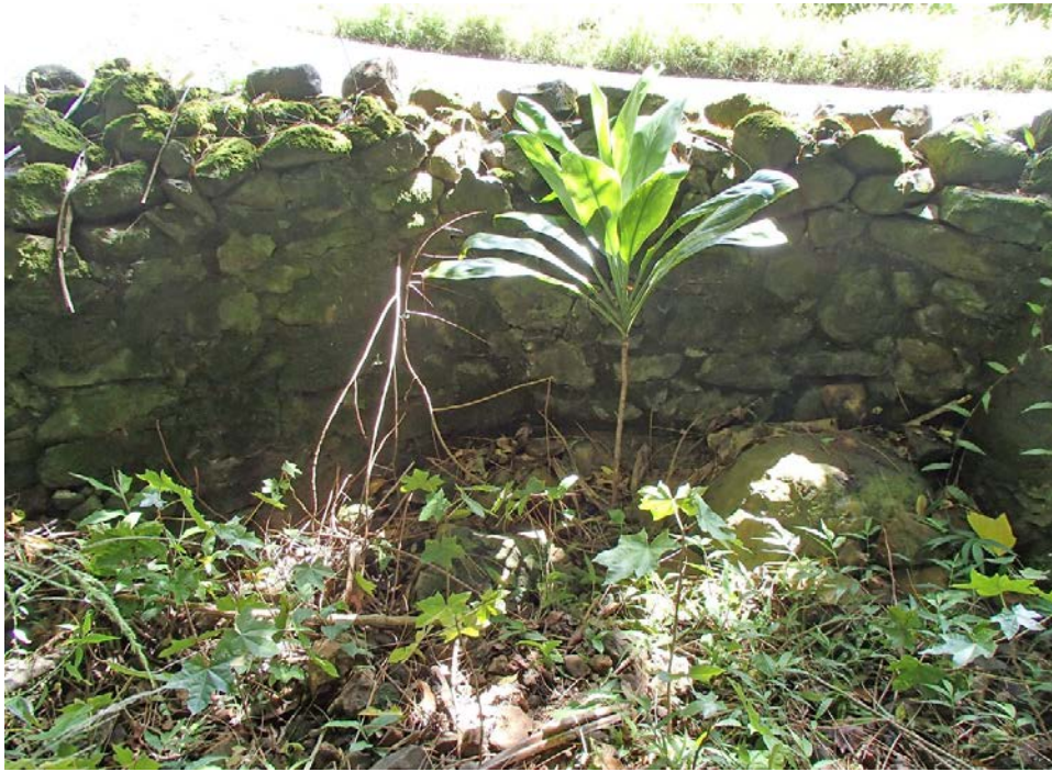
Upstream elevation of CRM parapet. Note: Nothing could be seen per description on as-builts.
