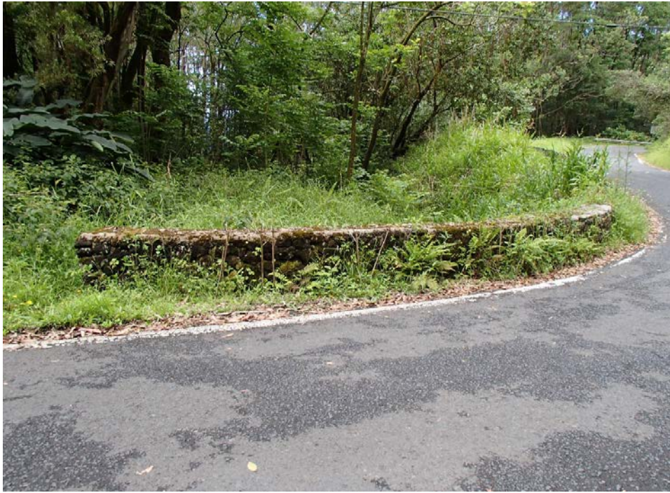
View of downstream CRM parapet.
