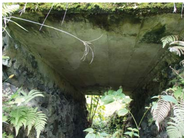
CRM abutments Courtesy of NOEI
