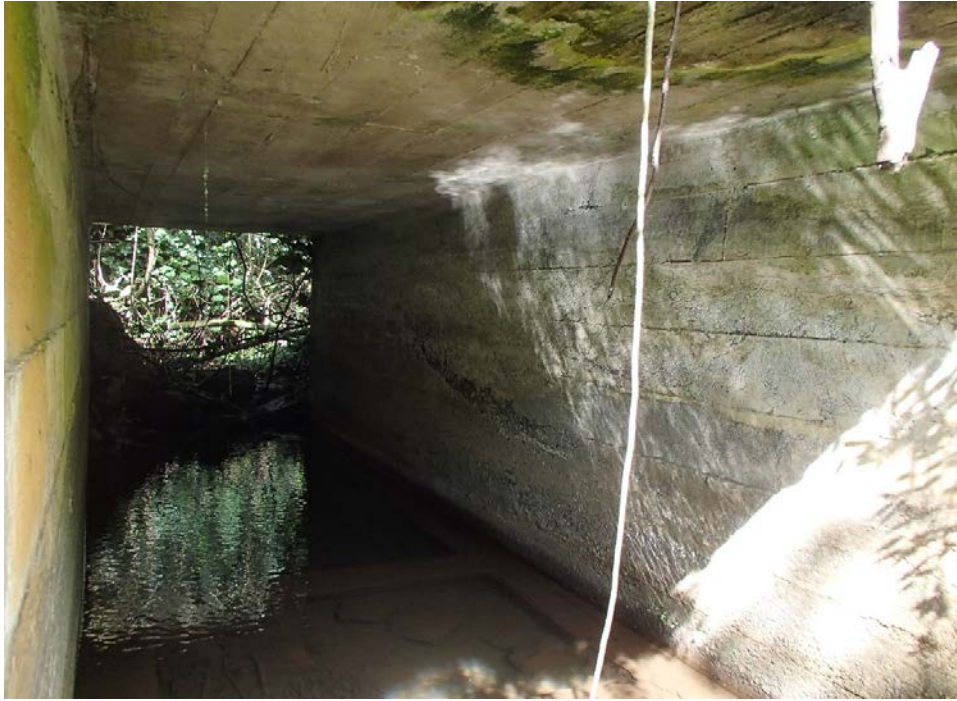
Upstream view through concrete box culvert.
