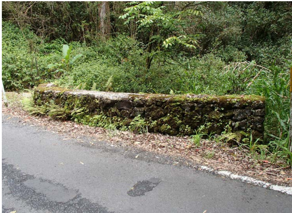
View of upstream CRM parapet.
