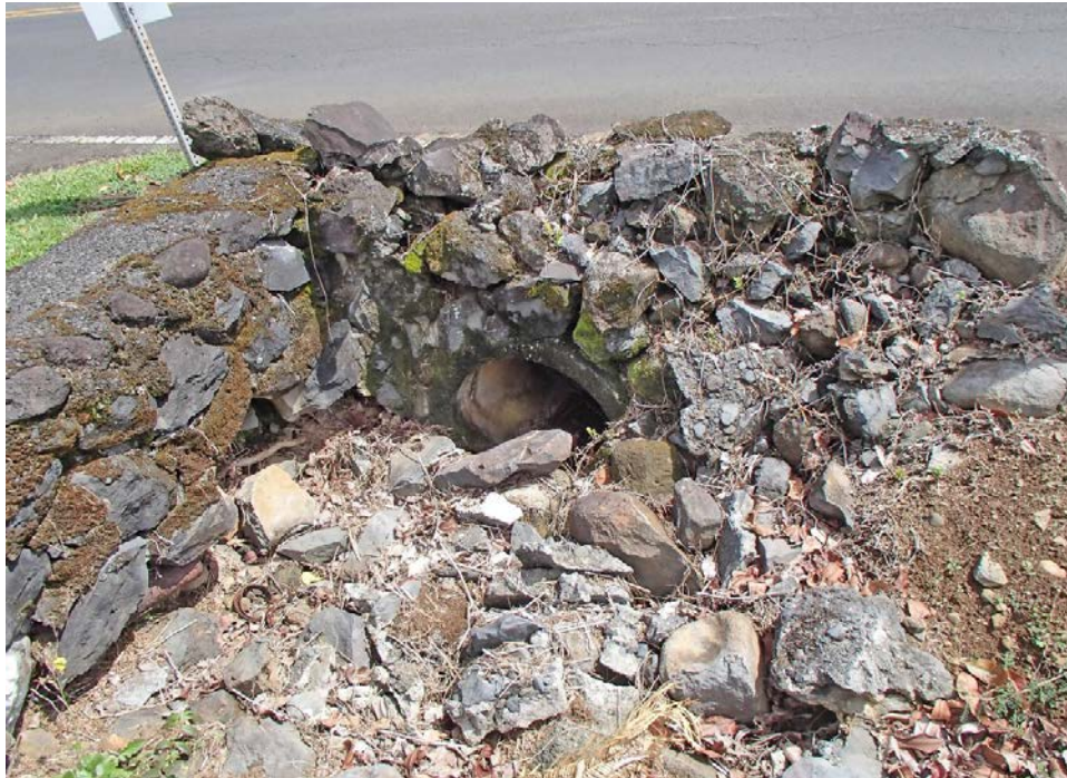
24" diameter RCP inlet at upstream side. Upstream / Hana corner of CRM parapet is damaged.
