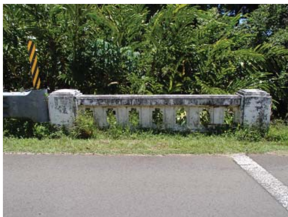
Greek cross parapet, downstream side Courtesy of NOEI
