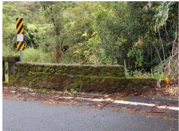
Exemplary CRM approach wall, Bridge #38 Heleleikeoha Stream Bridge Courtesy of NOEI
