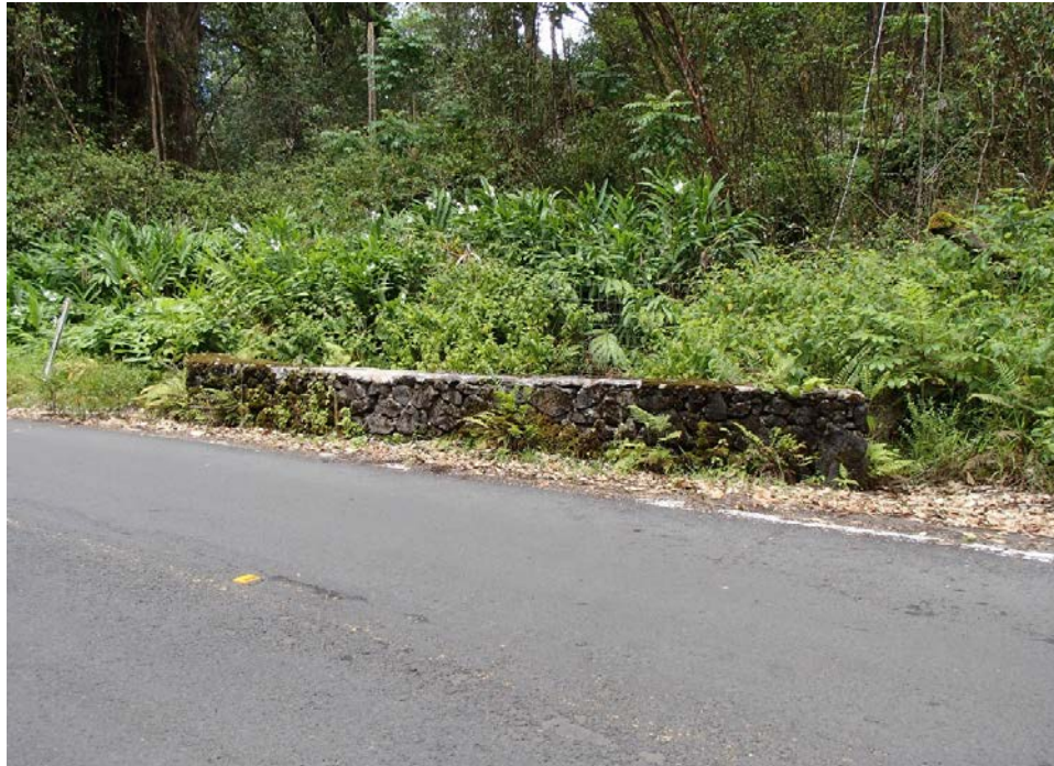
View of upstream CRM parapet.
