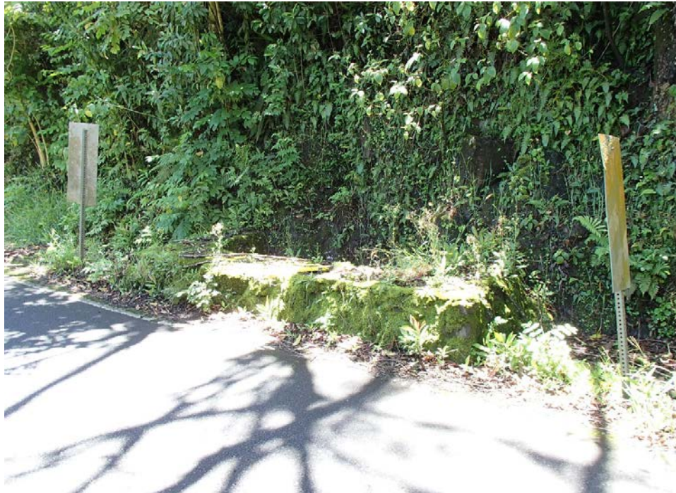
View of upstream CRM parapet.
