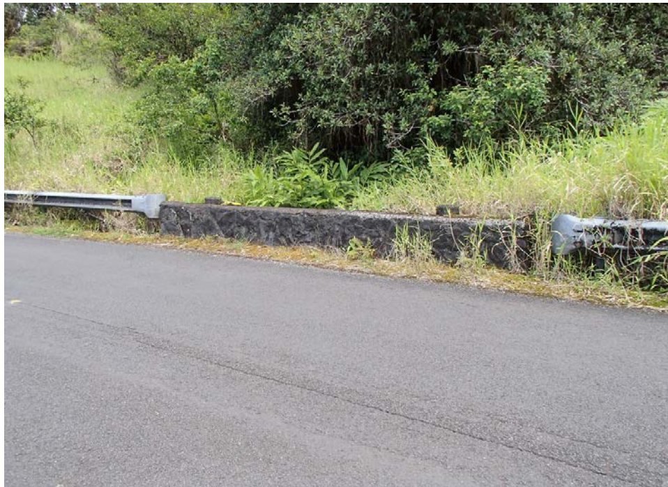
View of upstream CRM parapet.
