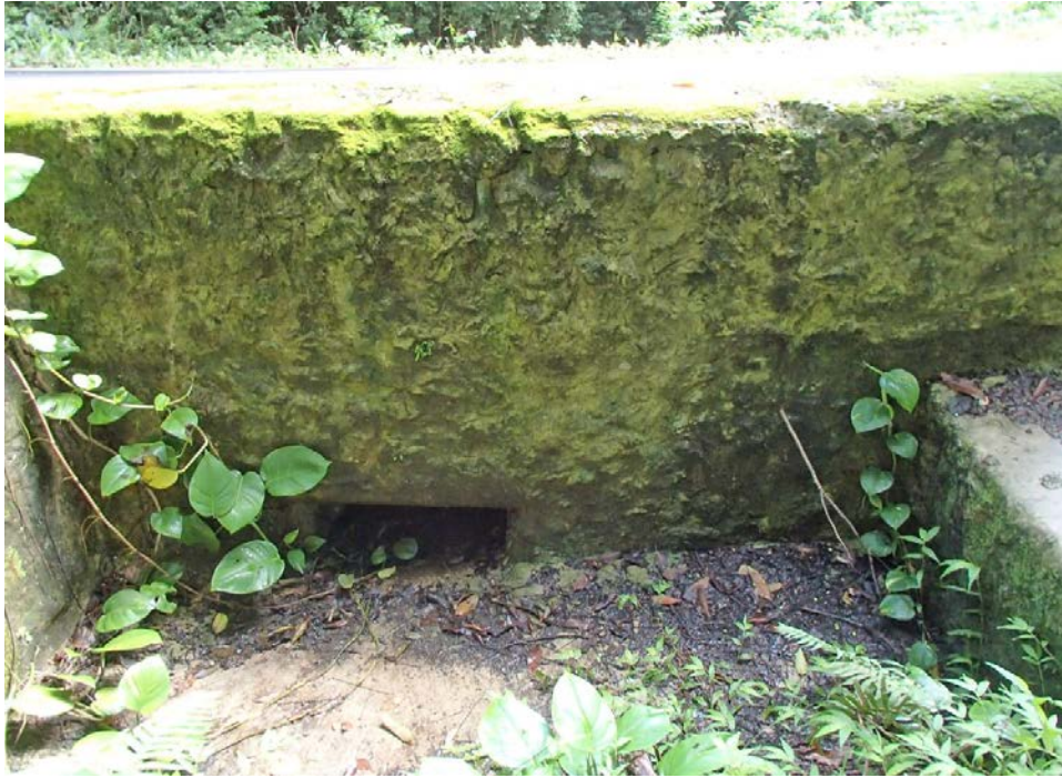
View of upstream CRM headwall / parapet and culvert inlet.
