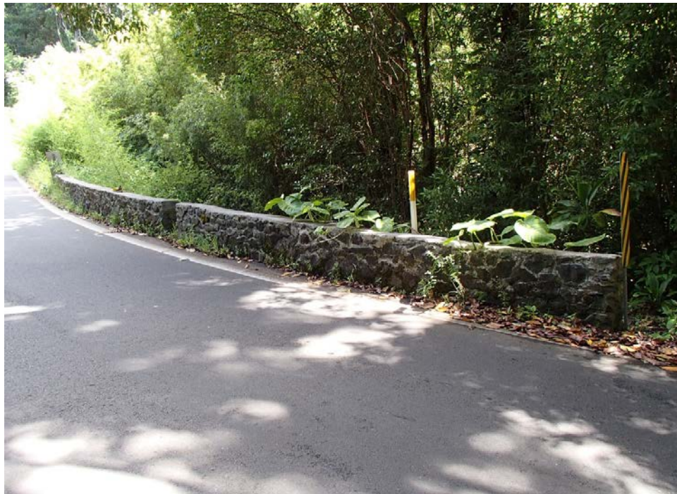
View of upstream CRM parapet.
