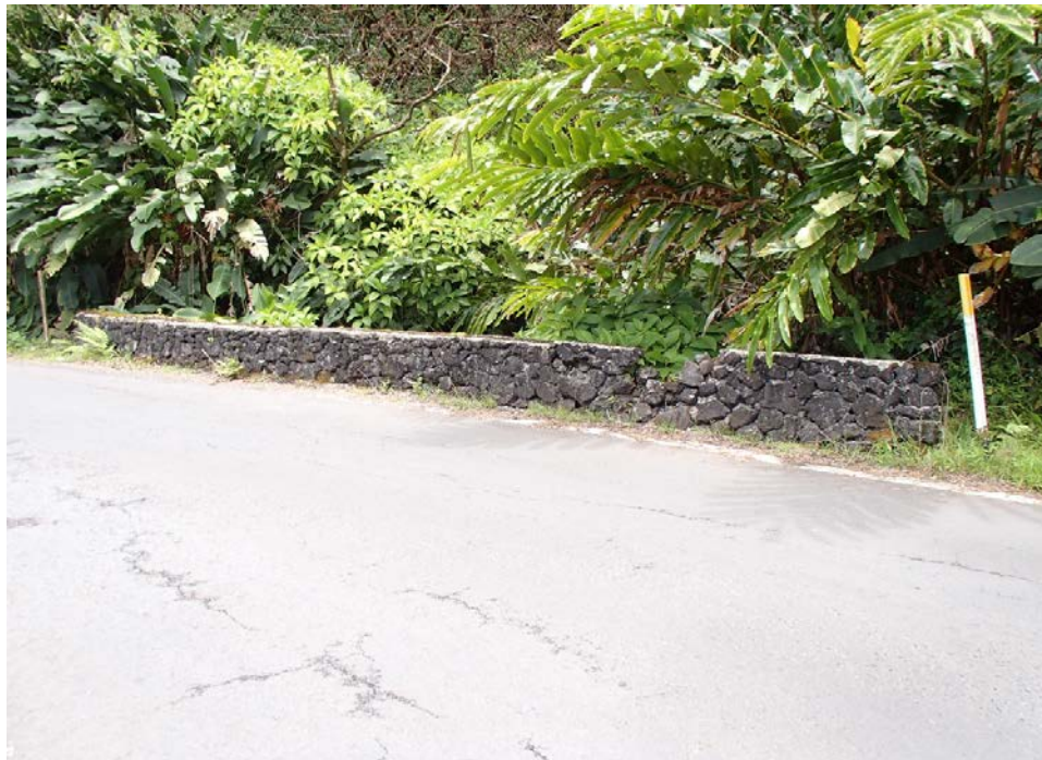
View of upstream CRM parapet.
