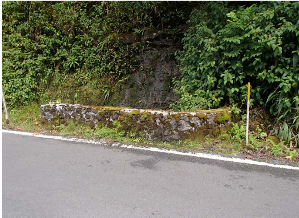
View of upstream CRM parapet.
