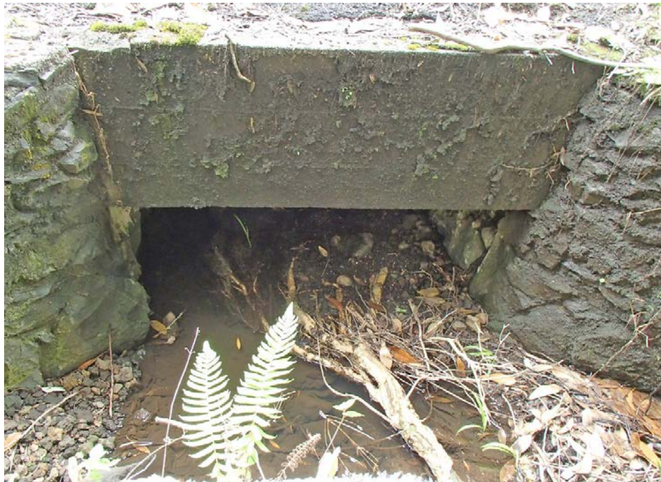
View of upstream concrete culvert headwall and CRM wingwalls.
