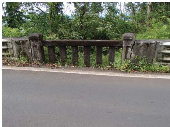
Concrete open railings with inset panels at end caps, downstream side Courtesy of NOEI
