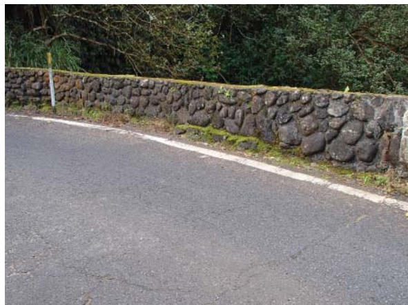
Exemplary CRM approach wall, Bridge #19 Kopiliula Stream Bridge Courtesy of NOEI
