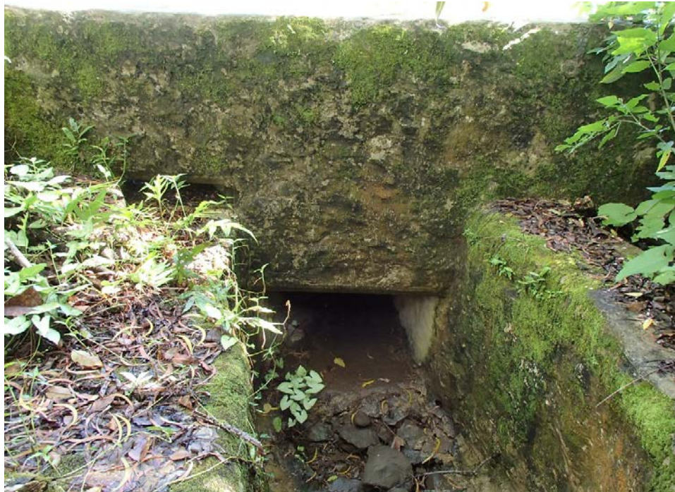
Backside view of upstream CRM headwall / parapet.
