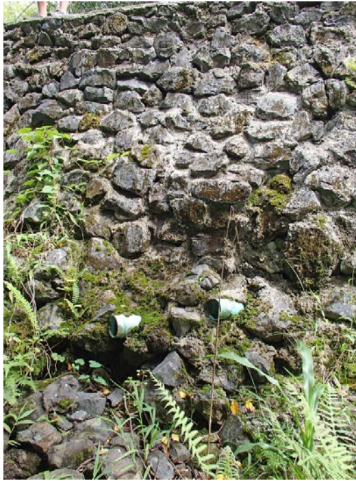
2 - 4" diameter pipe outlets at downstream side.
