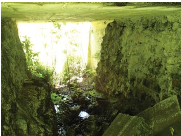
CRM abutment, Kahului and Hana sides Courtesy of FAI
