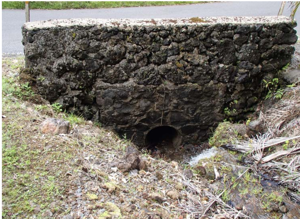
24" diameter RCP inlet at upstream side.
