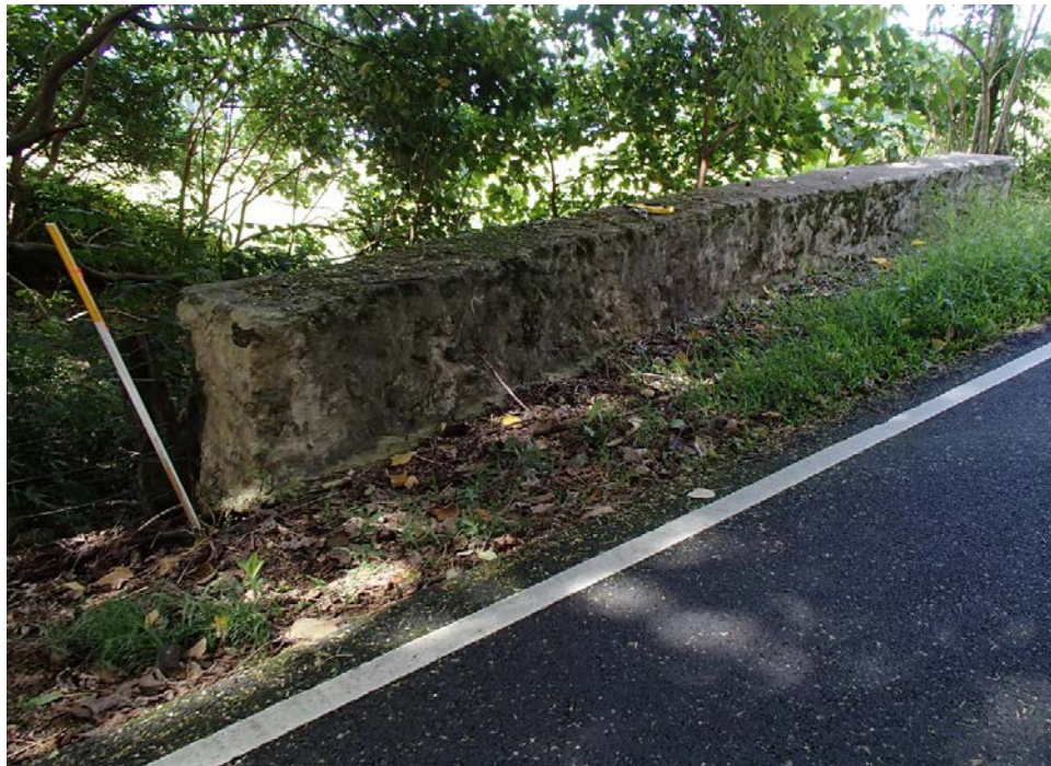
View of downstream CRM parapet.
