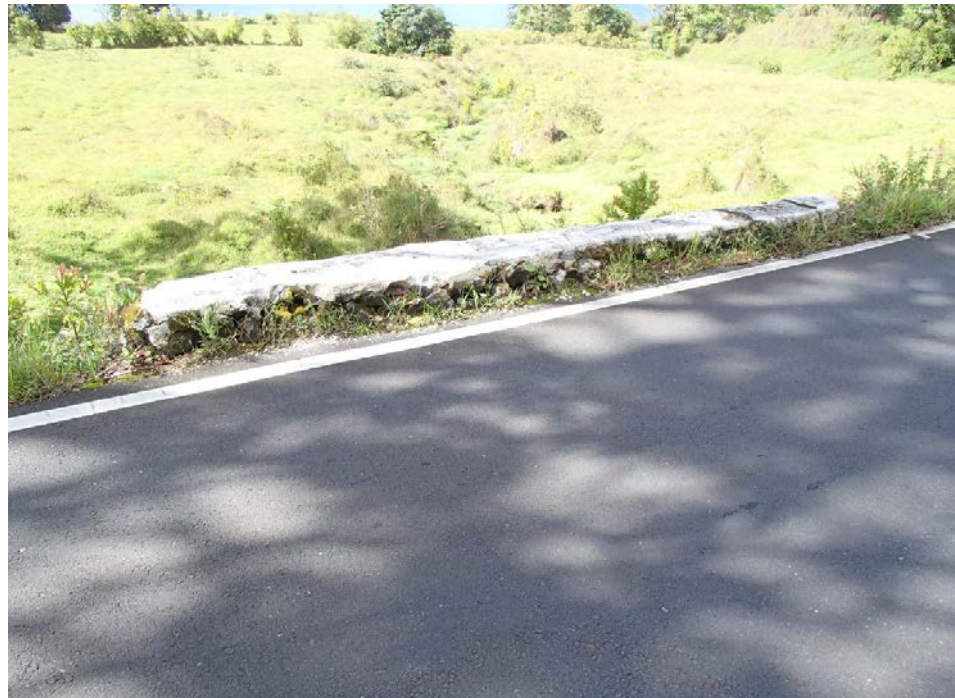
View of downstream CRM parapet.
