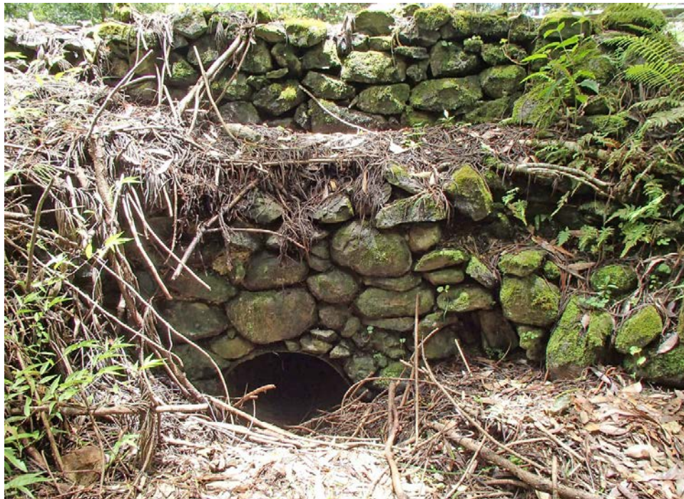
View of upstream CRM headwall / parapet and 30" diameter CMP inlet.
