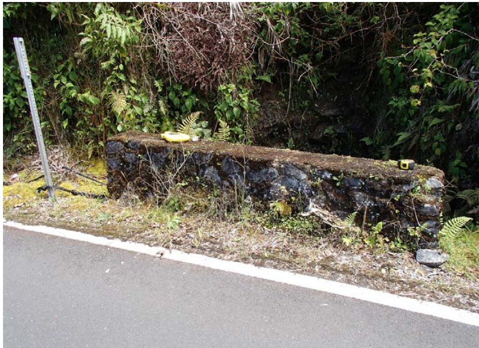
View of upstream CRM parapet.
