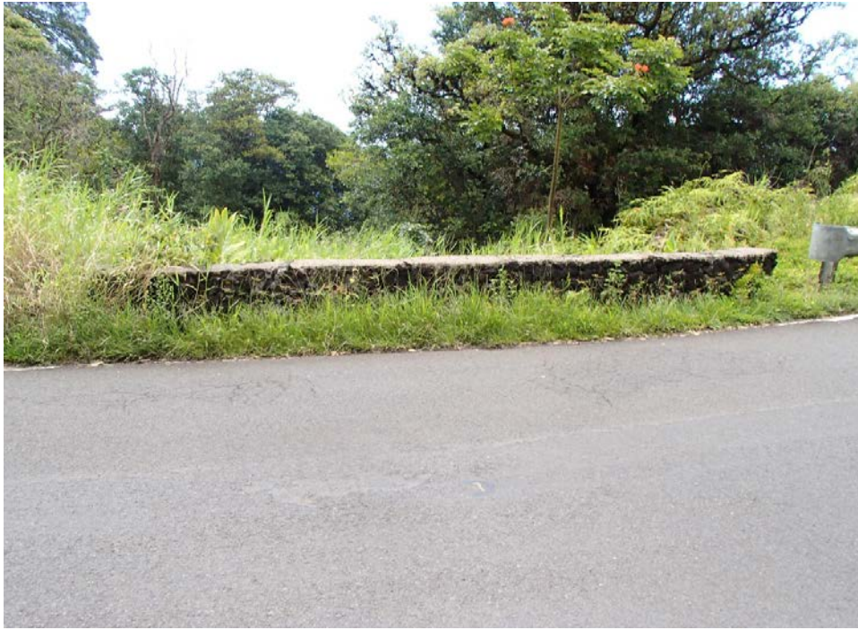
View of downstream CRM parapet.
