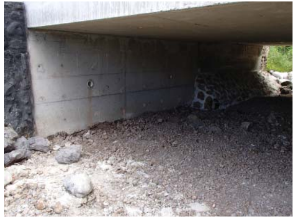
Concrete abutment, Hana side Courtesy of NOEI
