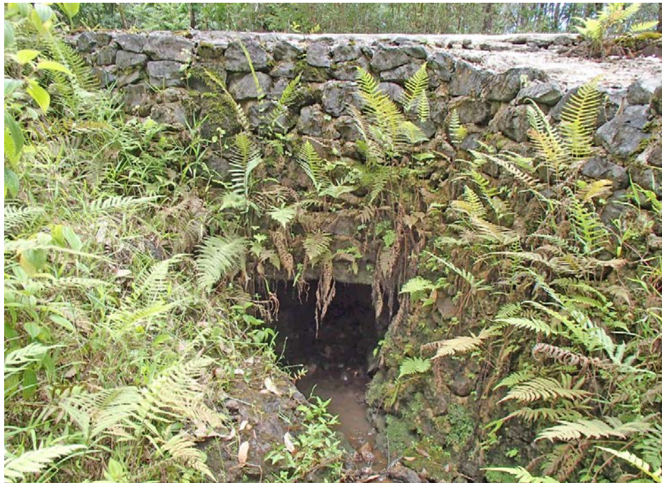
View of upstream CRM headwall / parapet.
