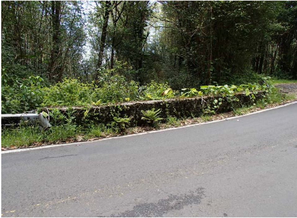
View of downstream CRM parapet.
