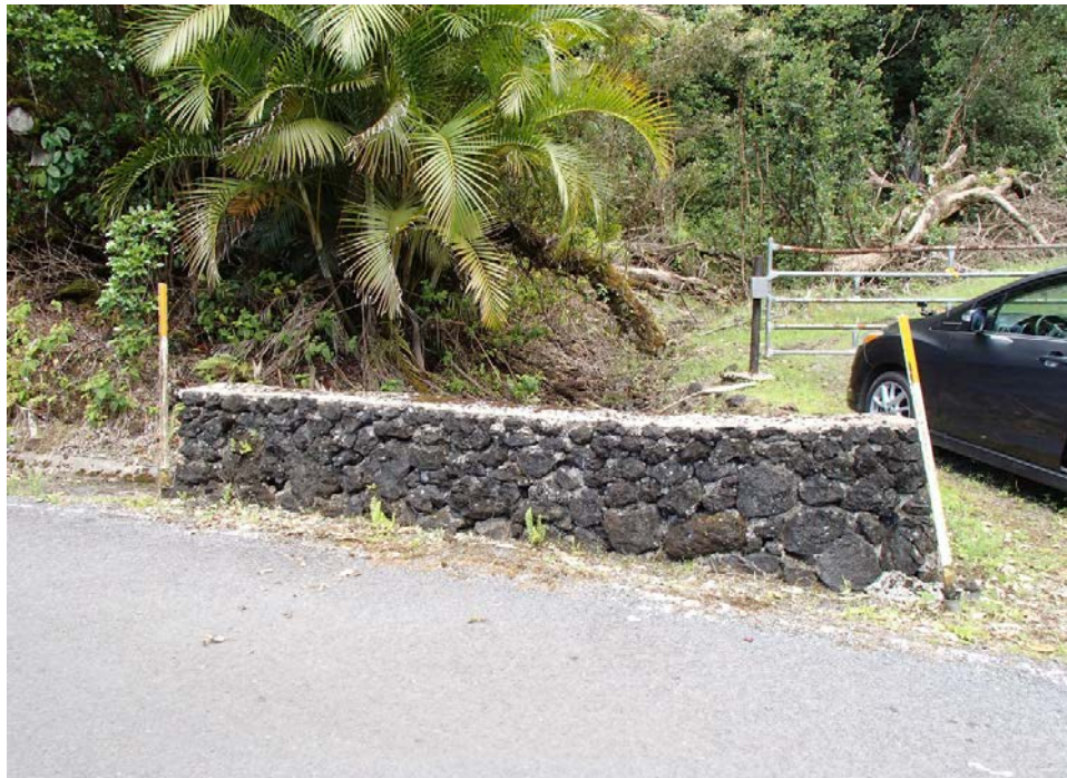
View of upstream CRM parapet.
