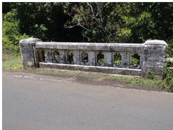
Greek cross parapet, upstream side Courtesy of NOEI
