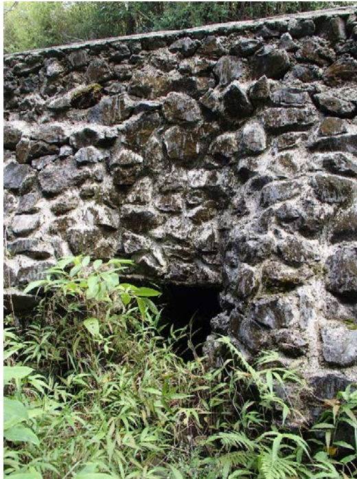
View of CRM headwall / parapet at downstream side.
