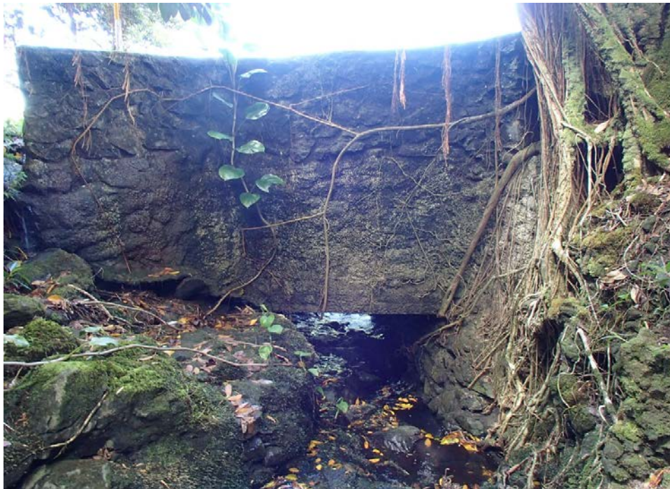
View of upstream CRM headwall / parapet and wingwalls.
