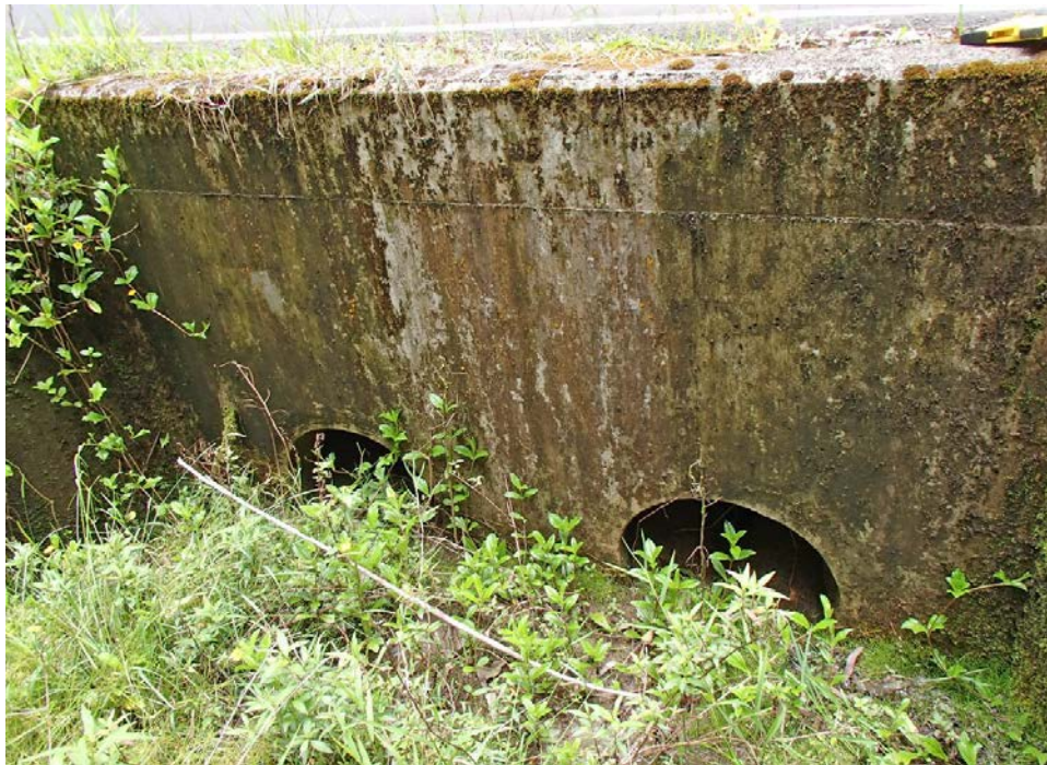
2 - 24" diameter RCP inlets at upstream side.
