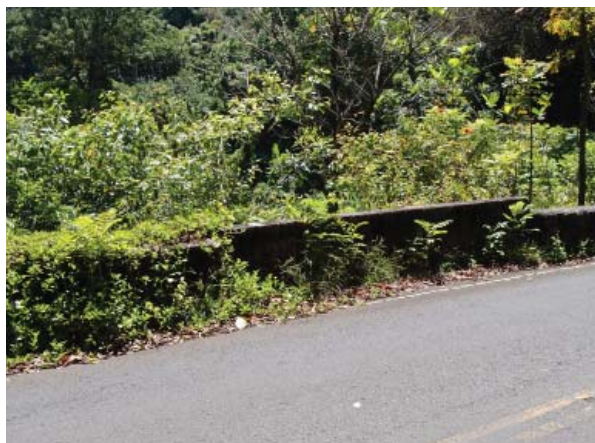
Solid concrete parapet, downstream side Courtesy of NOEI
