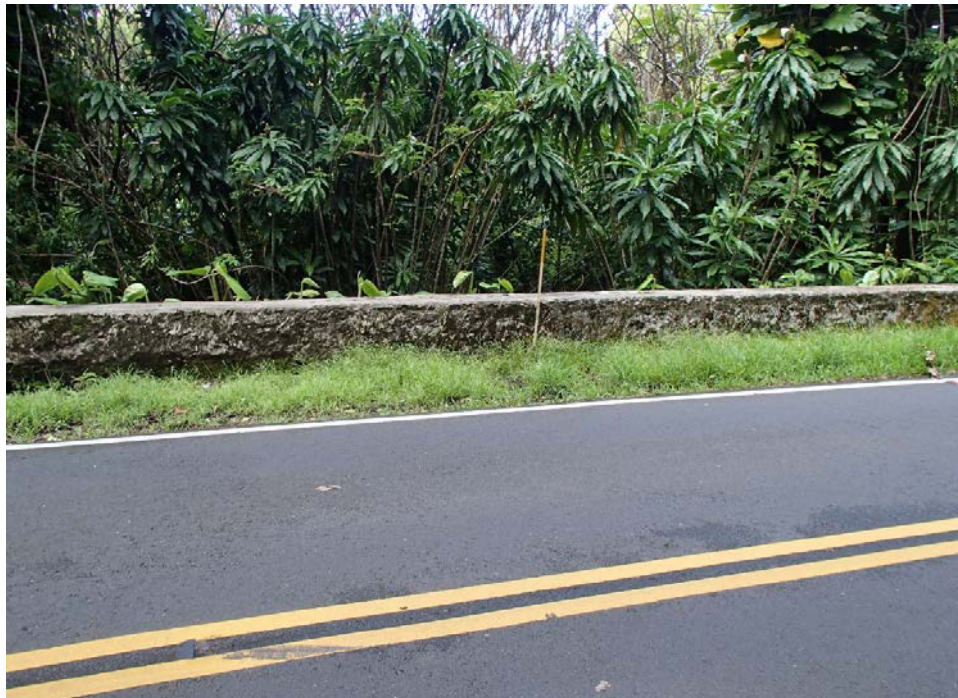
View of downstream CRM parapet.
