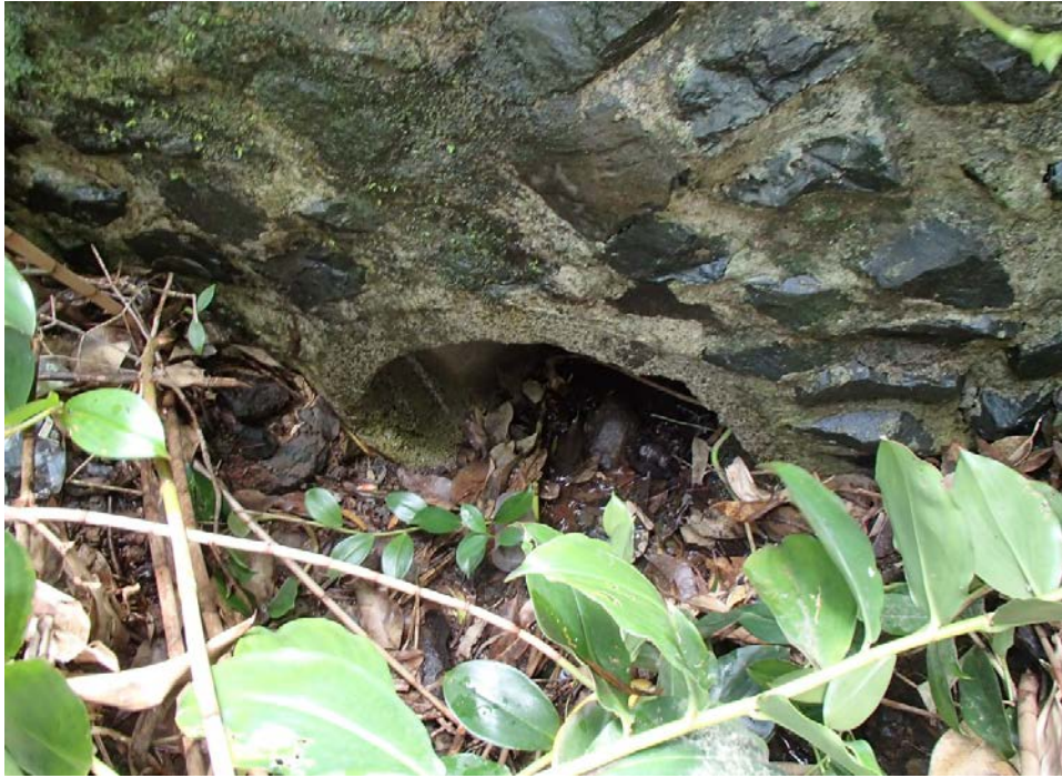
24" diameter RCP inlet at upstream side.
