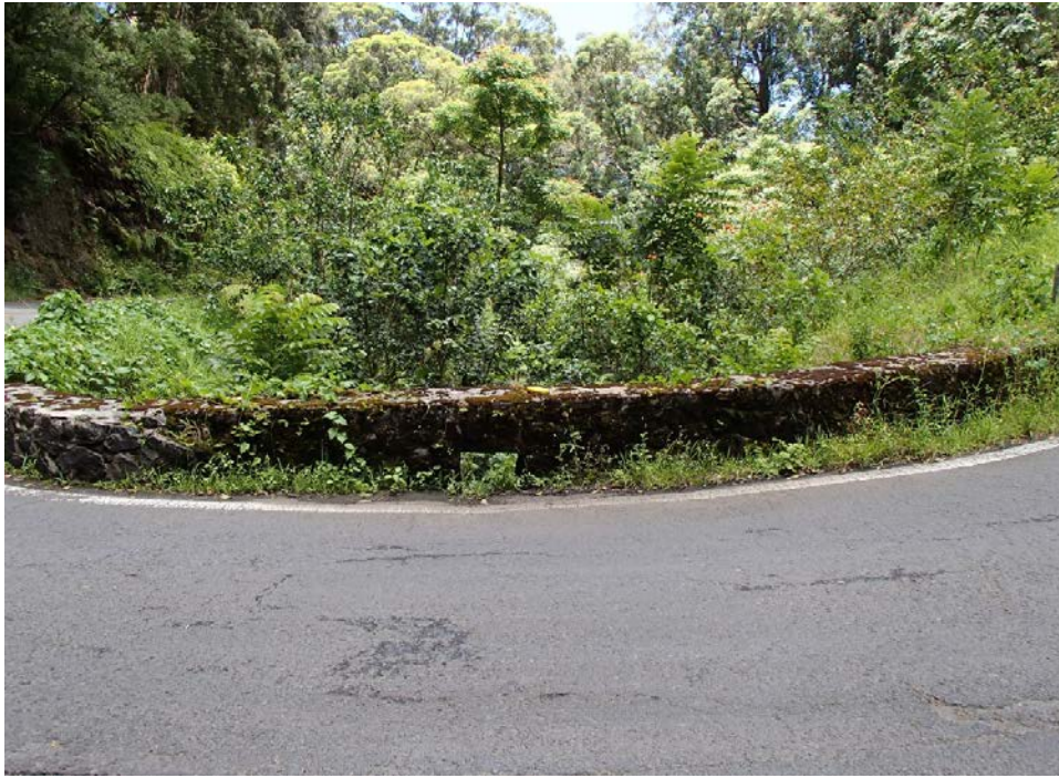
View of downstream CRM parapet.
