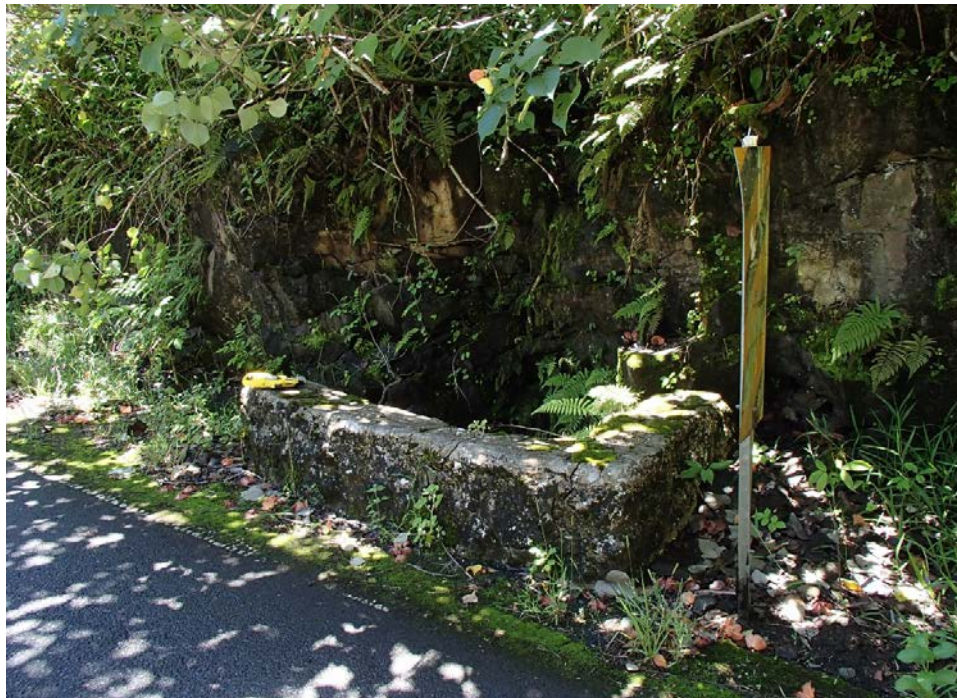
View of upstream CRM parapet.
