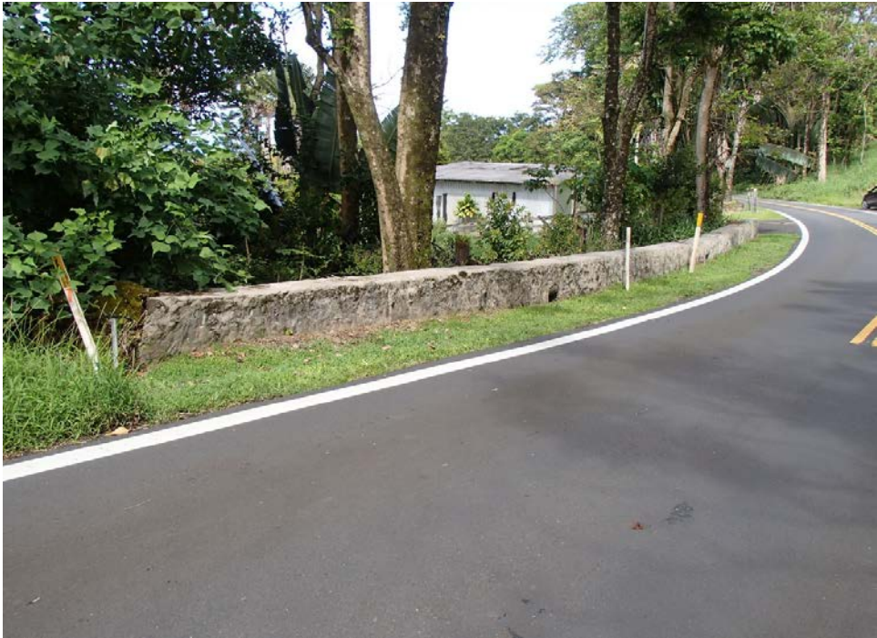
View of downstream CRM parapet.
