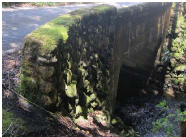
Exemplary CRM approach wall, East Hanawi Culvert Courtesy of FAI
