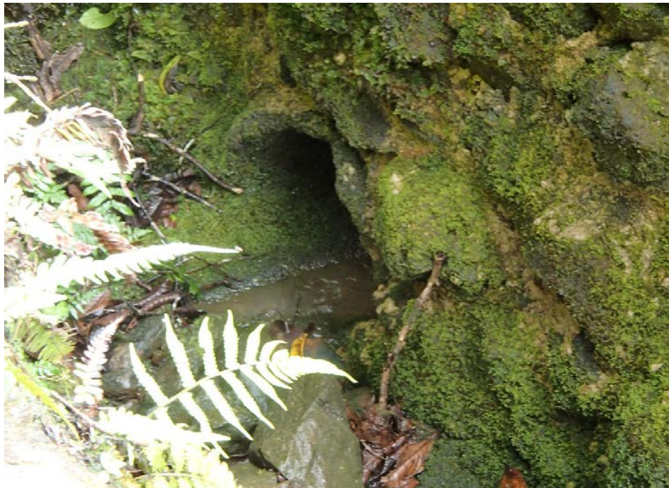
24" diameter RCP inlet at the upstream side.
