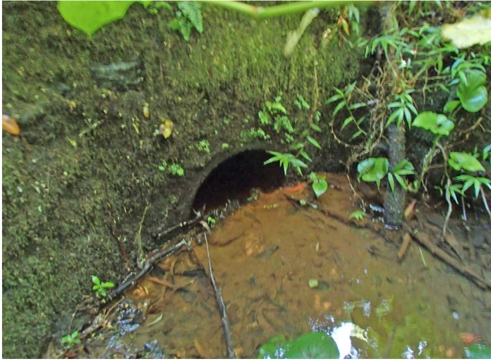
24" diameter RCP inlet at upstream side.
