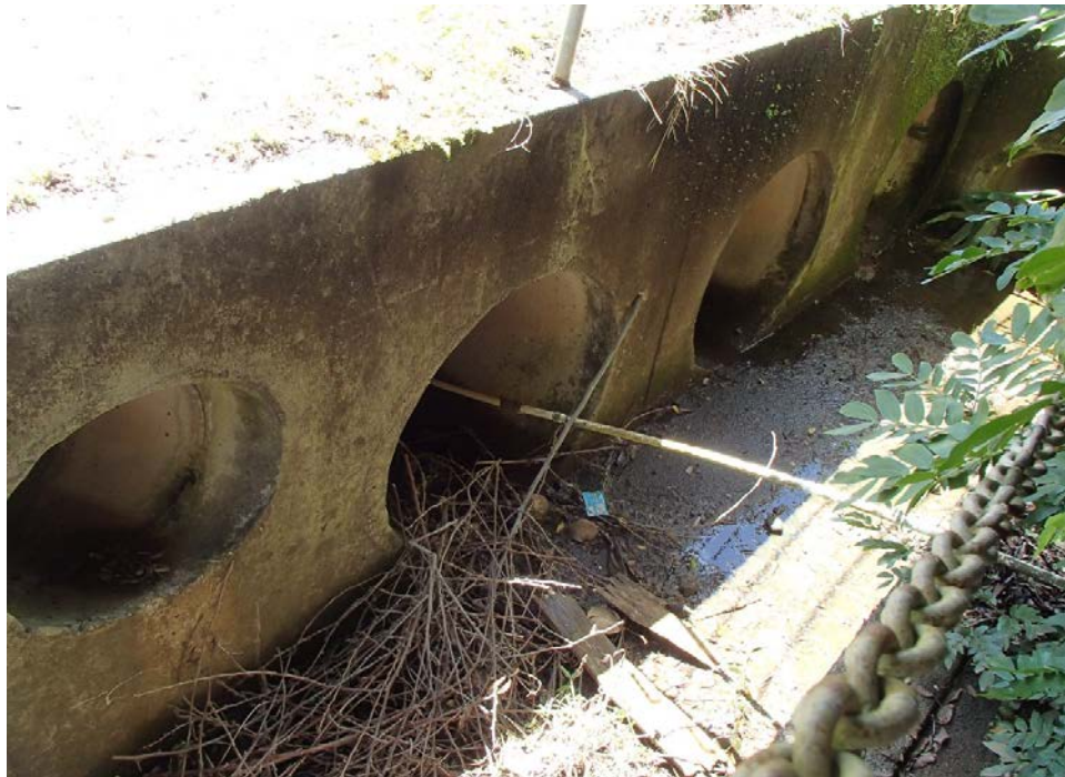
3 - 42" diameter and 1 - 24" diameter RCP inlets at upstream side.
