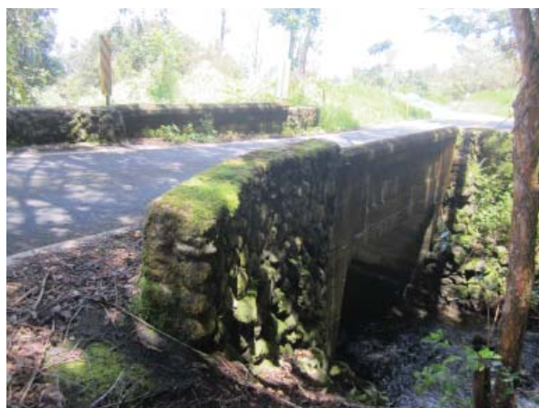
Upstream CRM approach wall, Kahului side Courtesy of FAI
