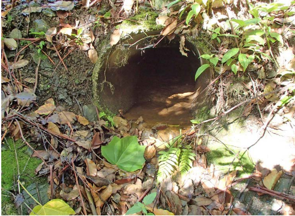
24" diameter RCP outlet at downstream side.
