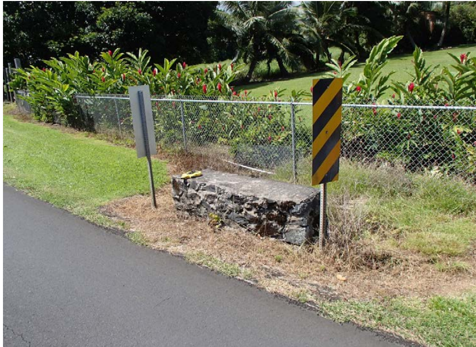
View of upstream CRM parapet.
