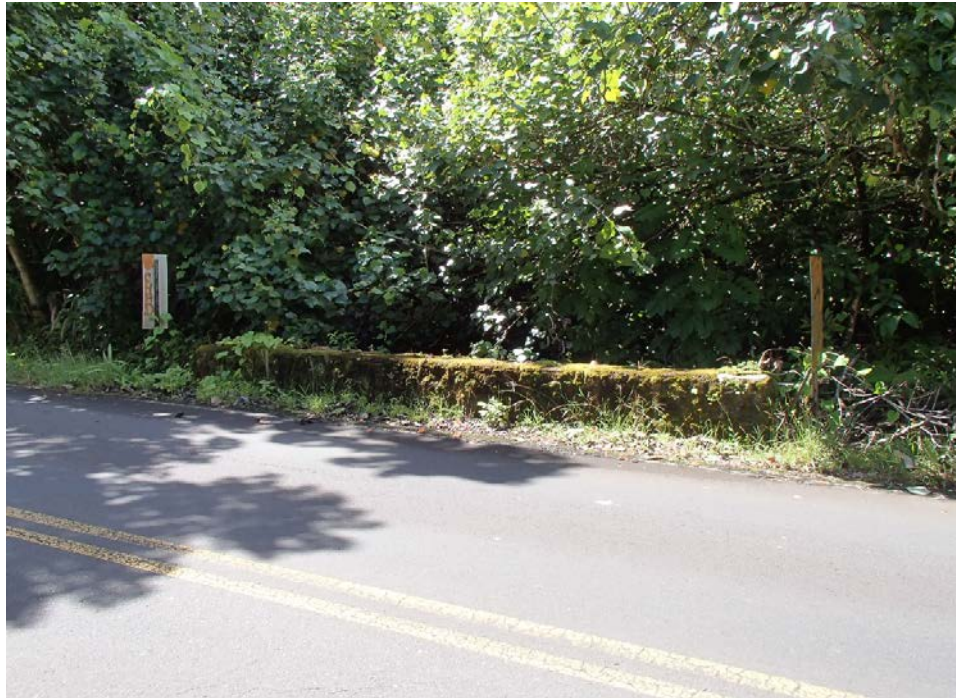
View of upstream CRM parapet.
