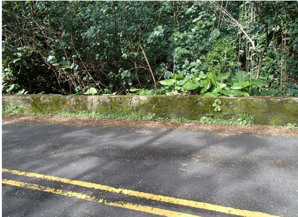
View of upstream CRM parapet.
