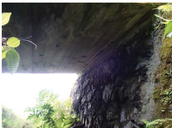
CRM abutment, Hana side Courtesy of NOEI
