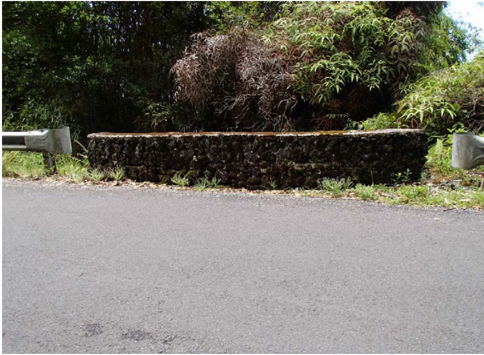
View of downstream CRM parapet.
