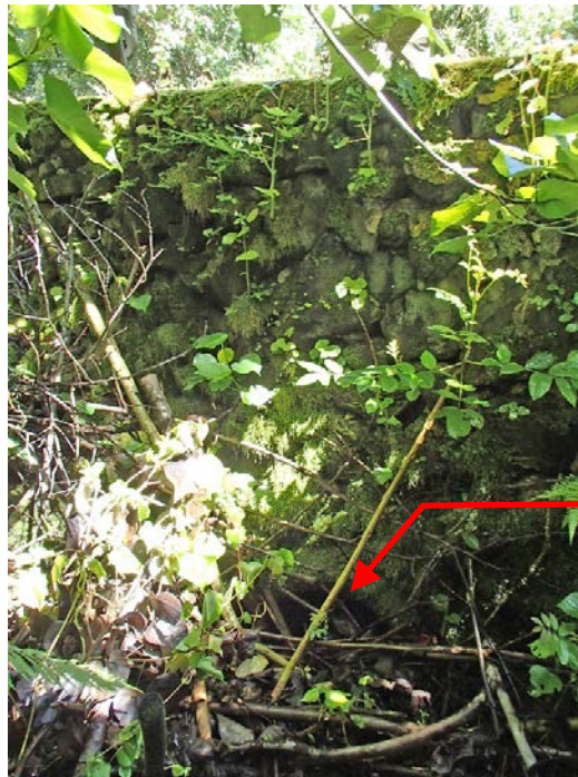
View of upstream CRM headwall / parapet and 24" diameter RCP inlet.
