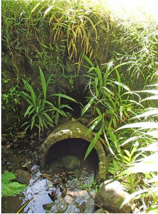
24" diameter RCP inlet at upstream side.
