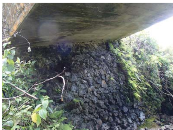
CRM abutment, Kahului side Courtesy of NOEI
