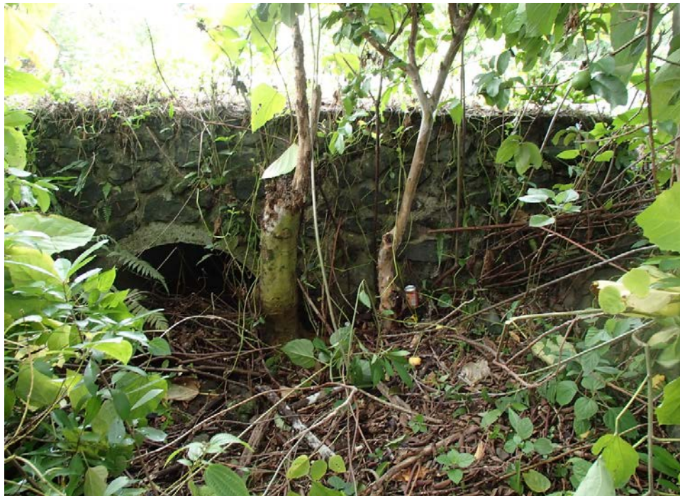
1 - 36" diameter and 1 - 24" diameter RCP outlets in downstream CRM headwall. 24" outlet is filled with debris.
