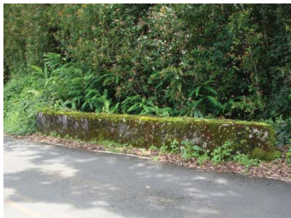
Solid concrete parapet, upstream side Courtesy of NOEI
