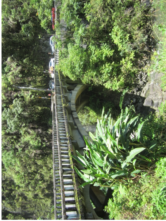
# 16 WAIKANI open spandrel concrete arch
