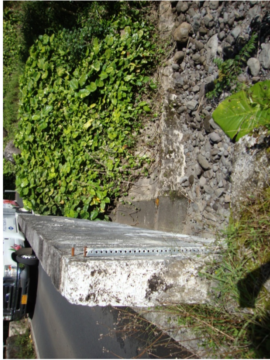
# 10 KOLEA-PUNALAU missing reflectors
