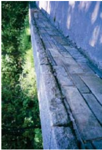
Example 2: TL-2 Rated Approach Wall Baltimore-Washington Parkway Railing (SBO03b)
