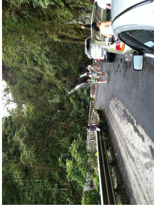
# 30 KUPUKOI missing parapet/wing wall/guardrail
