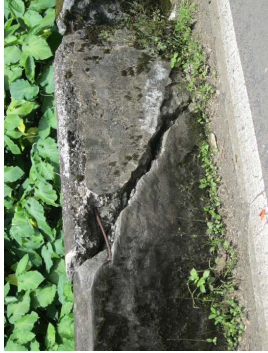
# 9 HAIPUAENA broken parapet
