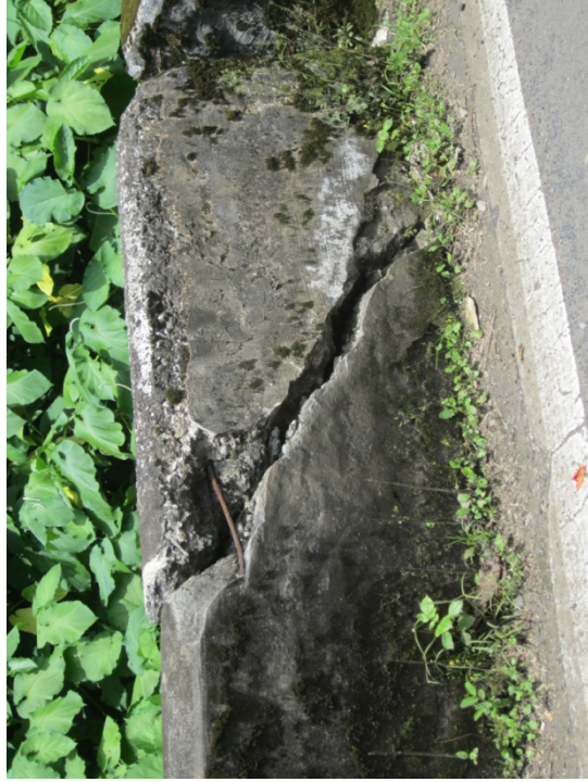
# 11 HONOMANU exposed re-bar / spalling
