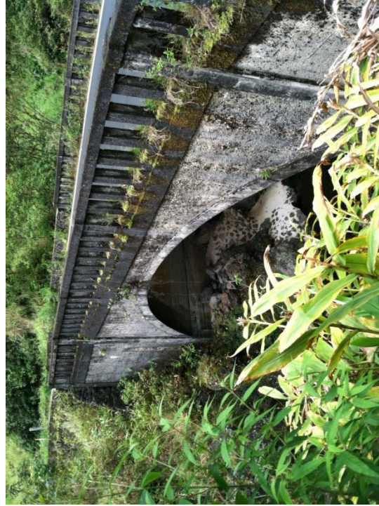
# 26 HANAWI single span concrete arch
