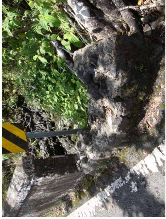
# 23 UNNAMED BRIDGE broken wing wall
