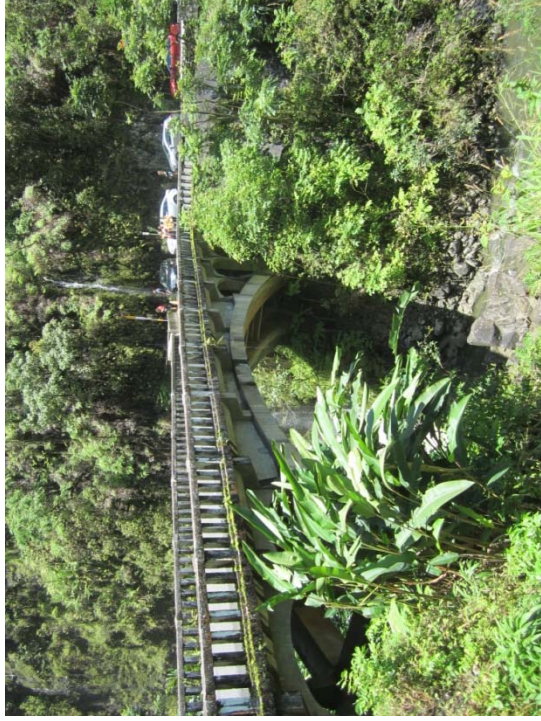
# 16 WAIKANI open spandrel concrete arch
