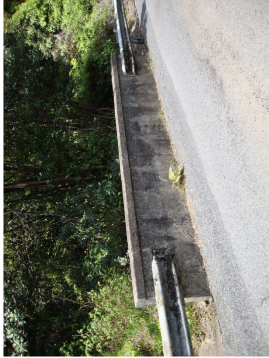
# 22 UNNAMED BRIDGE 1 - WAIOHUOLUA “W” guardrail attachment
