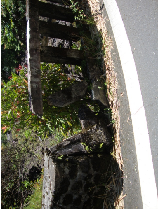
# 33 KAHAWAIHAPAPA broken parapet
