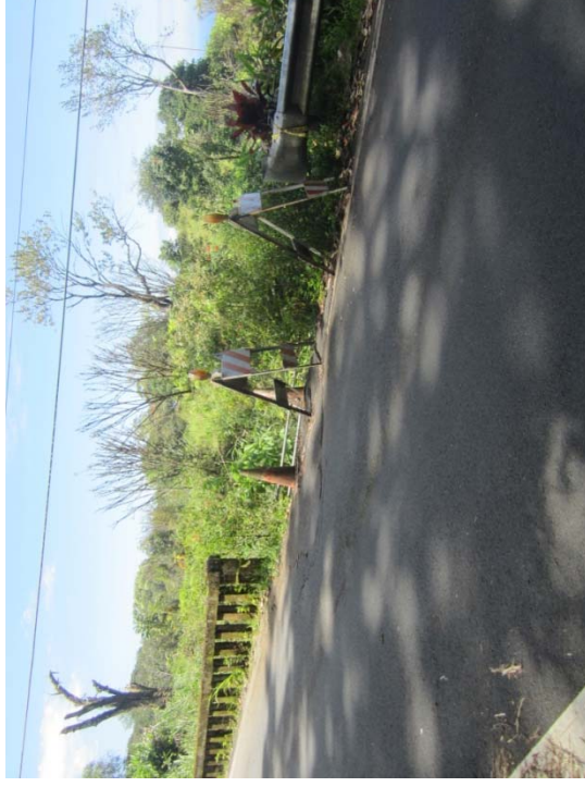
# 30 KUPUKOI missing parapet/wing wall/guardrail
