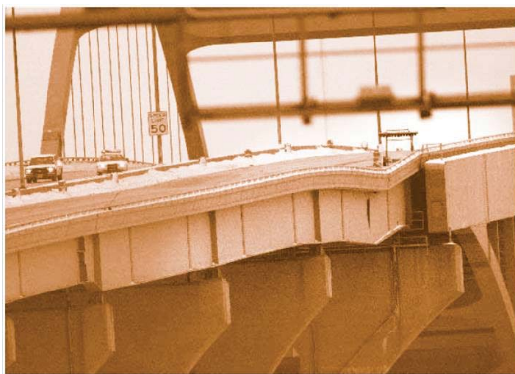
Figure 31 Structural failure on Daniel Webster Hoan Memorial Bridge, December 13, 2000.
