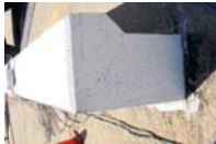
Example 1: TL-2 Rated Approach Wall Reinforced concrete wall with and without CRM façade
