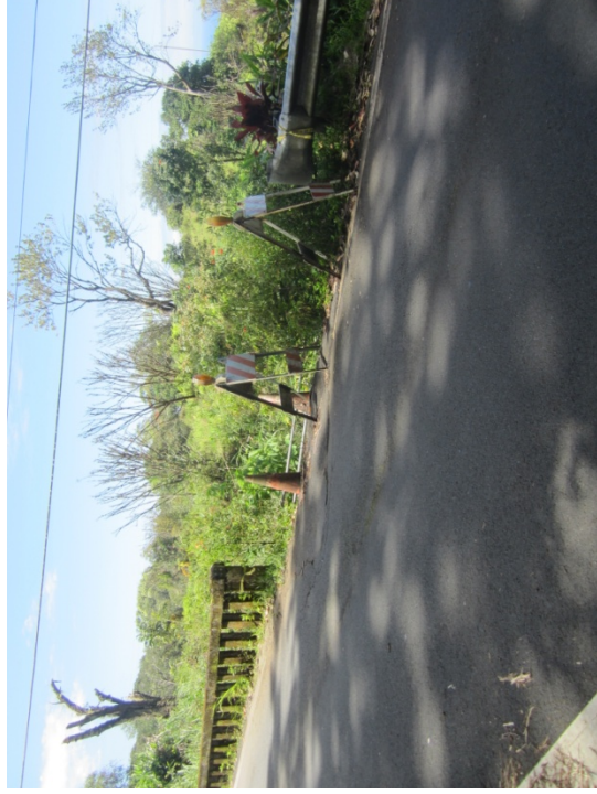
# 30 KUPUKOI missing parapet/wing wall/guardrail
