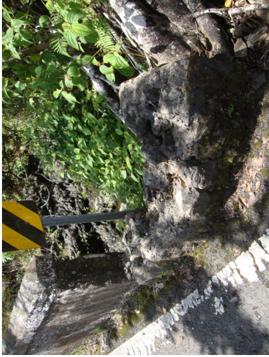
# 23 UNNAMED BRIDGE broken wing wall
