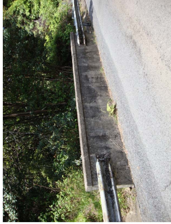
# 22 UNNAMED BRIDGE 1 - WAIOHUOLUA "W" guardrail attachment
