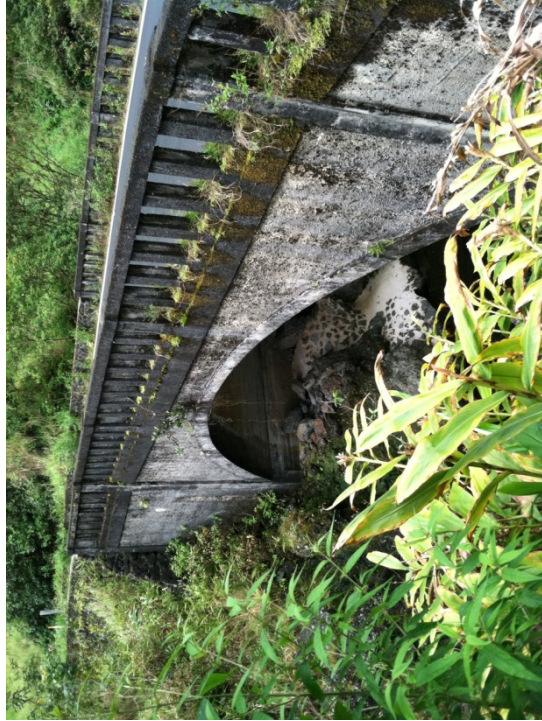
# 26 HANAWI single span concrete arch
