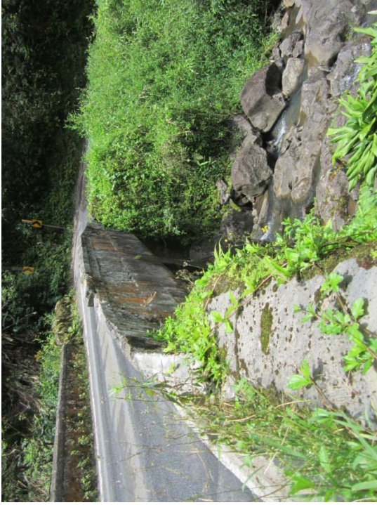
# 9 HAIPUAENA broken parapet
