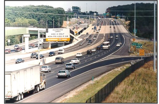
Figure 1-2: HOV Lane on Interstate 95 in Woodbridge, VA
