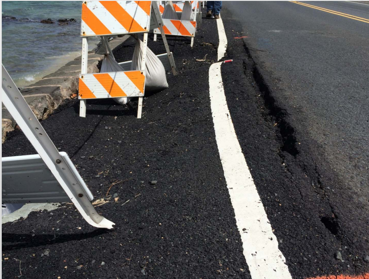
Continual Pavement Cracking along Lane Line
