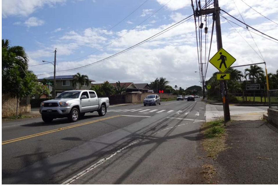
Example 3: Kalaniana'ole Highway at Nakini Street: Painted median and in-road pedestrian warning sign.
