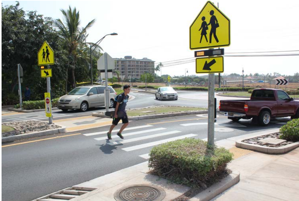
Example 8: Maui: Raised Median and pedestrian activated rectangular rapid flashing beacons.
