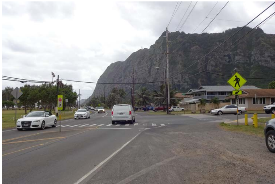
Example 3: Kalaniana'ole Highway at Nakini Street: Painted median and in-road pedestrian warning sign.
