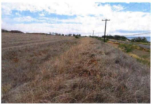
Drainage Basin 12. View along the continuous eight foot high berm above the cane haul road and Honoapi'ilani Highway that prevents any sheet flow rain water from getting down to these roads or to the coast.
