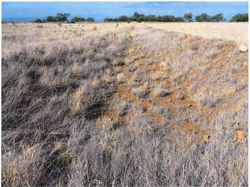
Drainage Basin 11. View down old ditch overflow channel showing straight-line construction and prominent lateral berms. This channel no longer receives water from the ditch or above it and cannot receive water from the sides because of the berms. It has not carried water in it since the plantation shut down fourteen years ago. There is no sign of silt deposition, debris accumulation or Ordinary High Water Mark.
