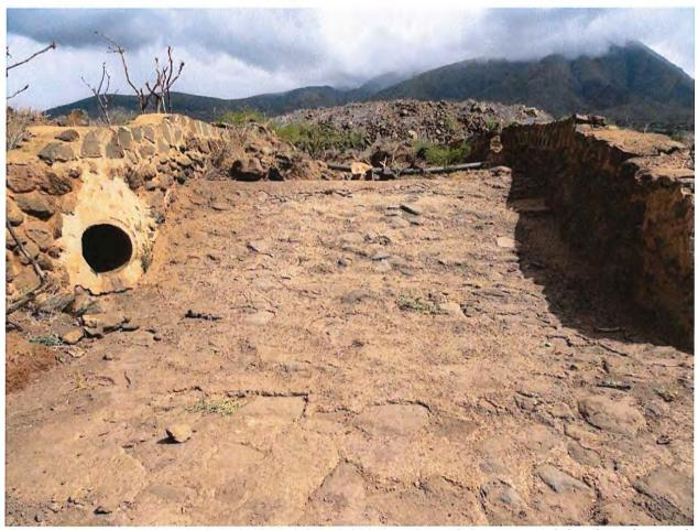
Drainage Basin 7. View upslope in the hardened drainage channel that protected the plantation road crossing which lies on the proposed road alignment. Small culvert on left brings in additional flow from within the same drainage basin.
