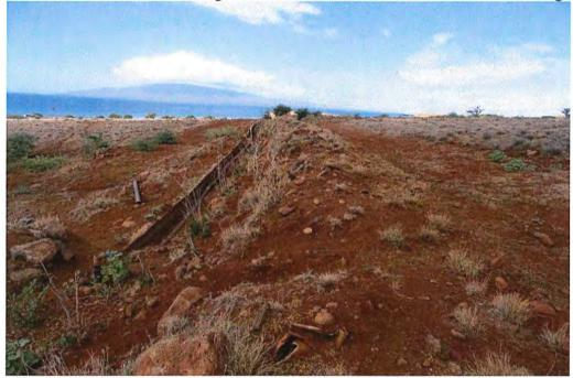
Drainage Basin 6. Proposed road alignment passes just below (to the right) the abandoned Lahaina Pump Ditch. Note: the three foot high berm that restricts any sheet flow from local rainfall from entering the ditch from above.
