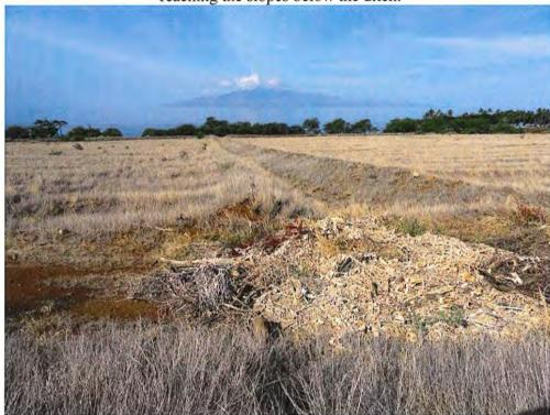
Drainage Basin 11. View downslope from the road alignment showing a straight man-made drainage that used to carry ditch overflow. This channel no longer receives water from the ditch and appears not to have carried water for years. There are no flow marks, debris or Ordinary High Water Marks.
