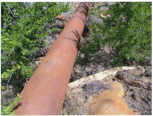
View of the 40 foot long x 30 inch diameter iron pipe spanning Launiupoko Stream channel.
