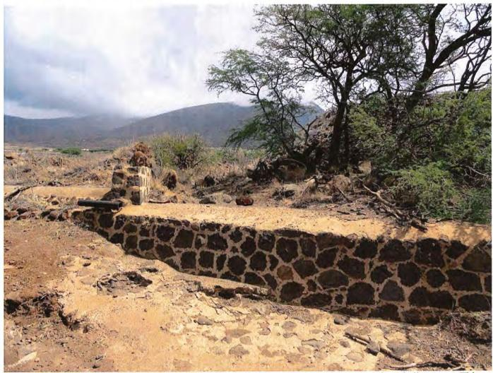
Drainage Basin 9. View upslope in a partially hardened channel above the proposed road alignment. This stream channel, which equates to Drainage Way 2 in the Sept., 2012 report, was found to be a Jurisdictional Ephemeral Stream with direct connections to the Pacific Ocean TNW through culverts under the cane haul road and the coastal highway.
