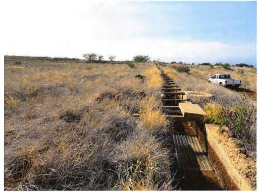
Drainage Basin 11. View along old ditch. Proposed road alignment lies below the ditch on the right. A three foot high berm on the left prevents any sheet flow from above from reaching the slopes below the ditch.
