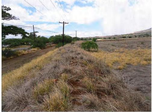
Drainage Basin 11. View along the continuous lateral eight foot high berm above the cane haul road and Honoapi'ilani highway that prevents any sheet flow rain water from getting down to these roads or to the coast.
