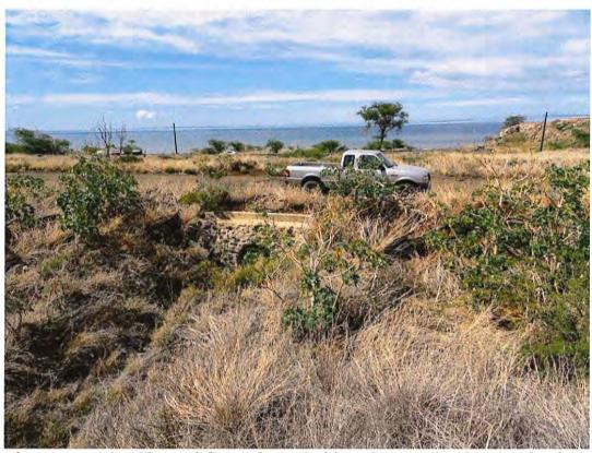
Drainageway 16 – Channel flows through this culvert under the cane haul road, through another box culvert under Honoapi'ilani Highway and directly into the ocean to the left of the kiawe tree.
