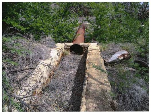
View of a 40 foot length of steel pipe spanning Launiupoko Stream channel to a ditch continuation on the far side that used to carry excess waters to the settling basin.
