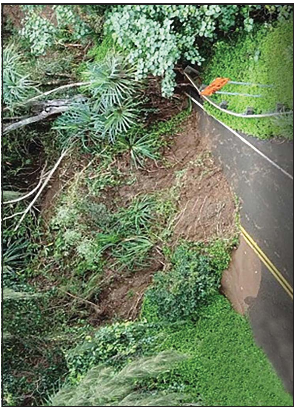
Landslide Site C
