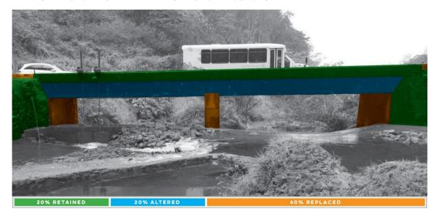
Alternative #2 – Retain Existing Bridge/ New Off-Alignment Bridge
